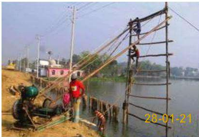
Plate 8: Erosion protection measures
