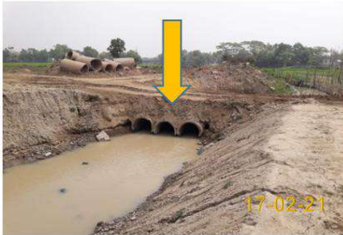
Plate 7: Installation of reinforced pipe (arrow) on temporary diversion to allow surface water flow
