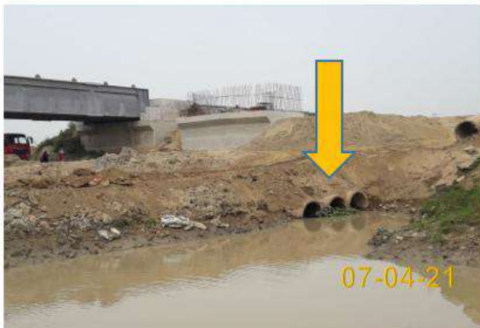
Plate 9: Installation of reinforced pipe (arrow) on temporary diversion to allow surface water flow
