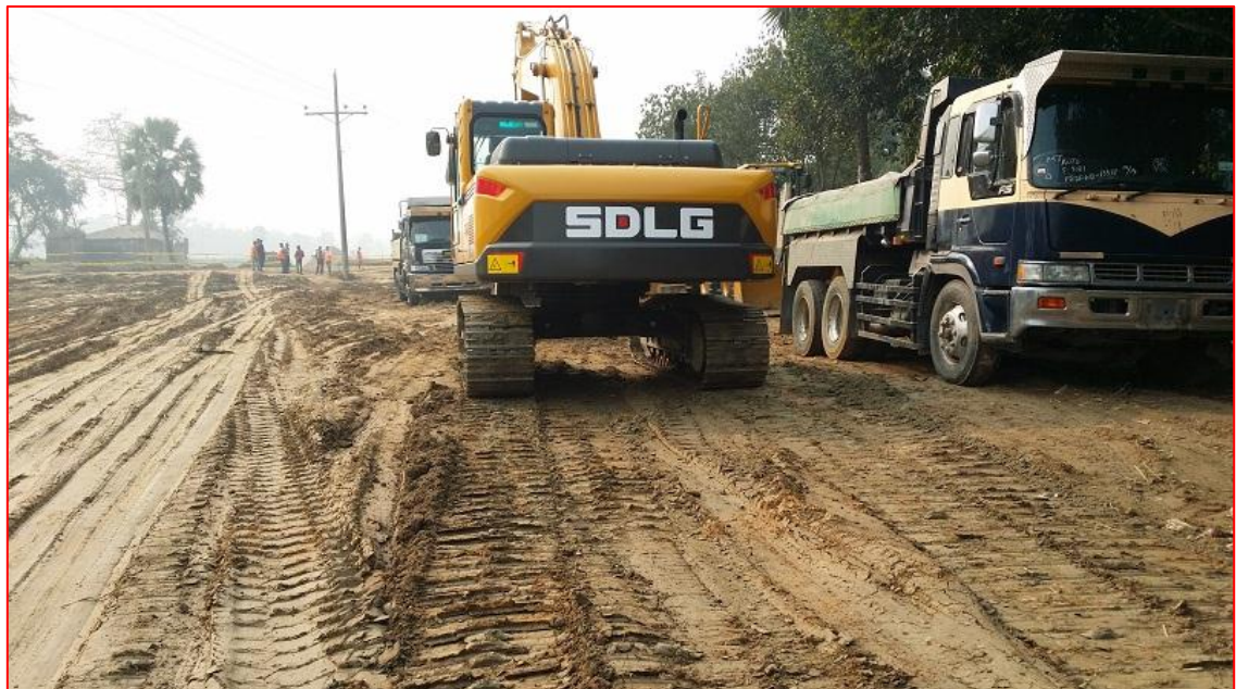
Photo 2. Trimming of slopes with topsoil at chainage .....
