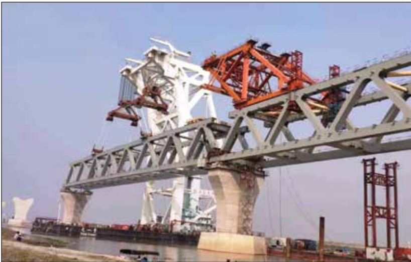
Span installed at Padma Bridge
