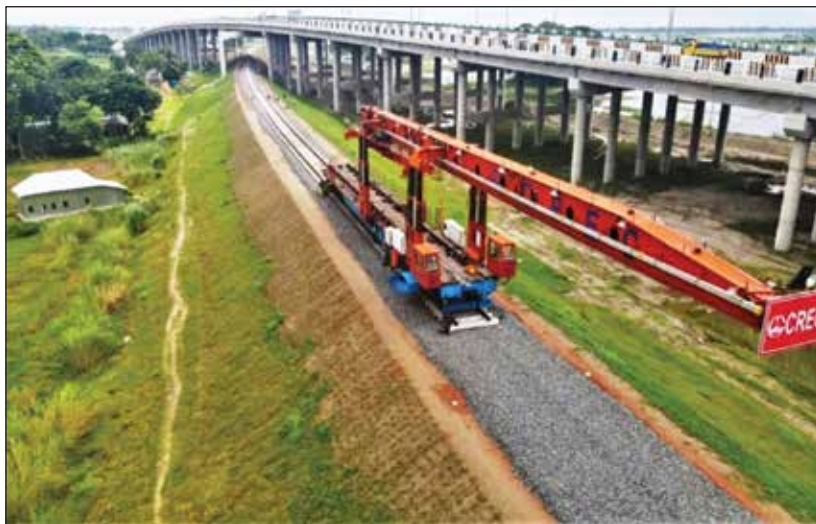
Installation of Railway track under Padma Bridge Rail link project
