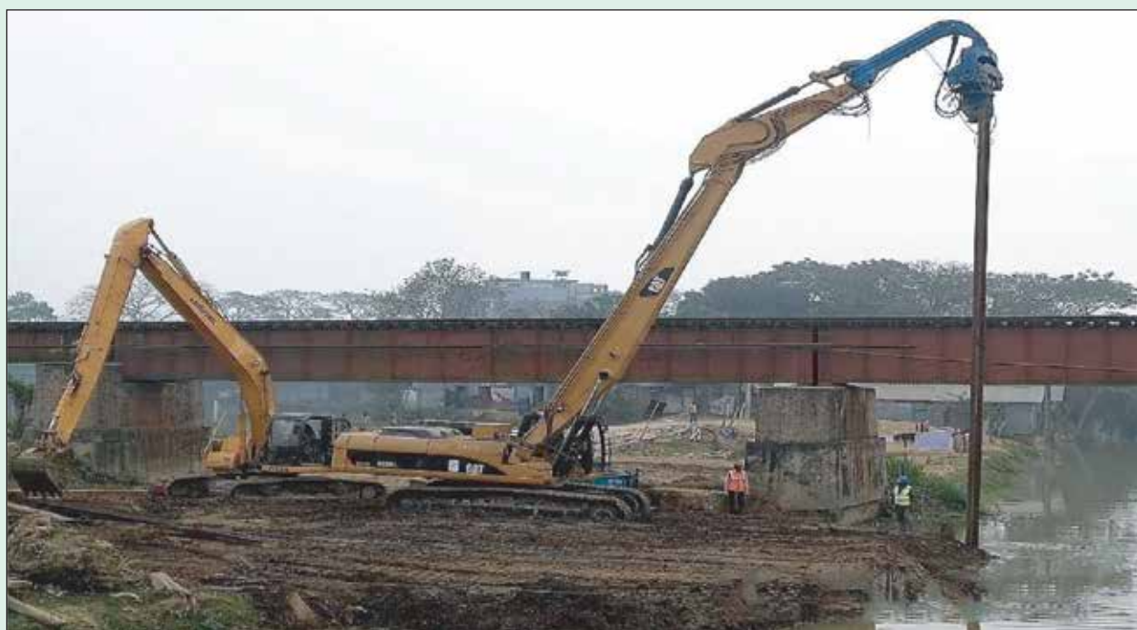
Excavator Working for Piling in a project
