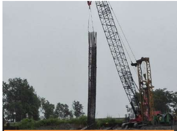
Cage installing-workers are in safe distance
