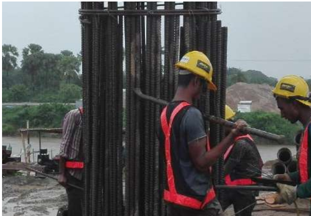
Welding-not all workers using eye protecting device
