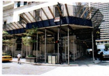
Safety canopy with curb board
