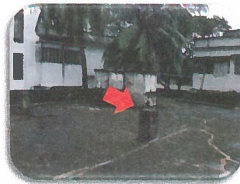
Figure 2.5.9 Possible Place of Collection of Reinforcing-bar Sample
