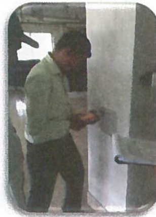
Figure 2.5.7 Schmidt Hammer Test after Stripping off Plaster
