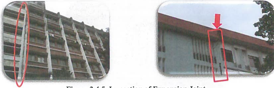
Figure 2.4.5 Inspection of Expansion Joint
