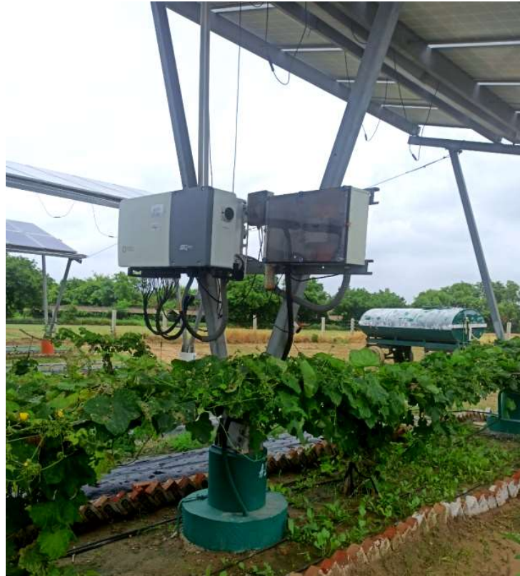
Figure10-7: Trellising of vegetables with wires tied to solar structure
