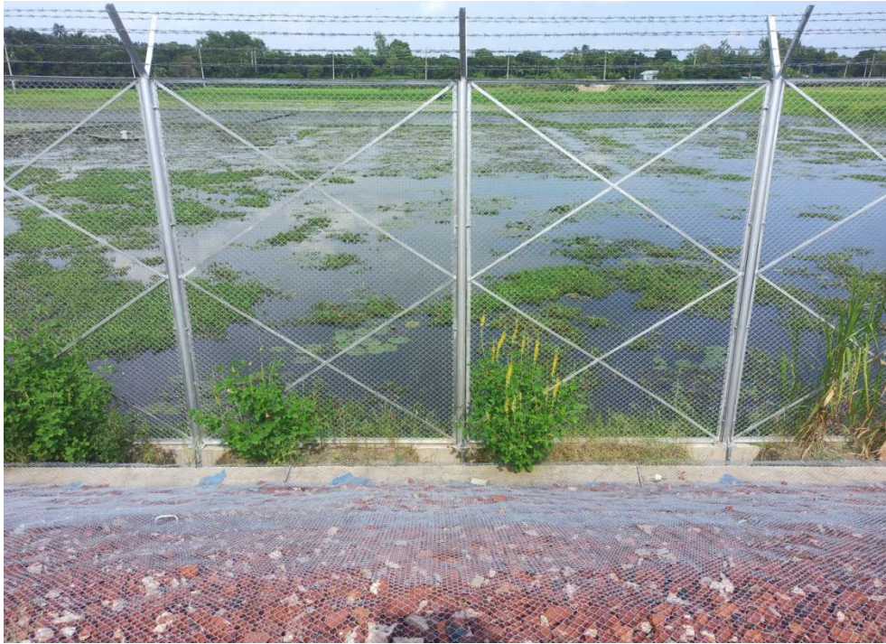
Figure9-7: River Padma on South West side of the Spectra solar plant.
