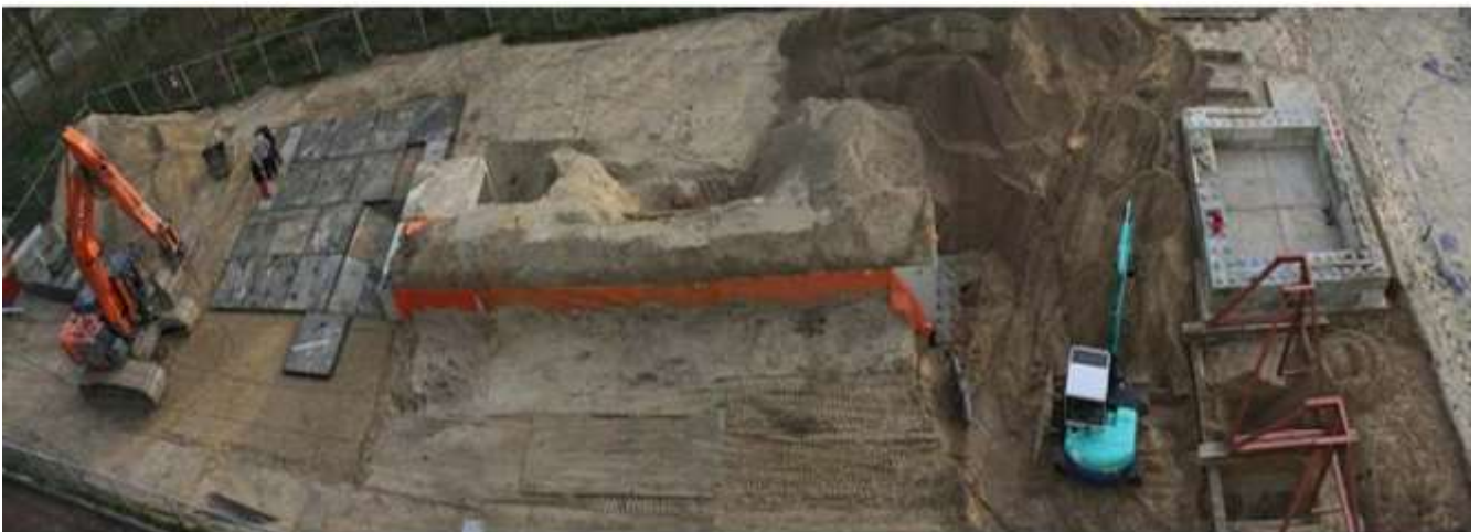
Figure D4 – 8 – Construction of the test side for the prequalification tests of Power Cables with rated voltage above 170 kV
