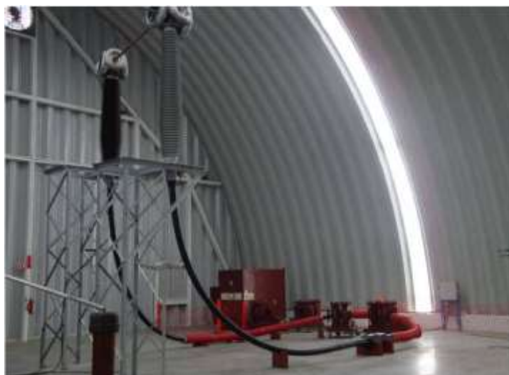
Figure D4 – 5 – Heating test on Power Cables
