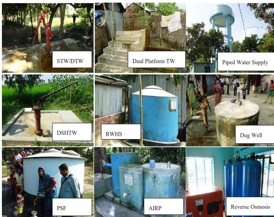
**Figure 7.1: Examples of installed area specific water supply technologies in different HtR areas by NGO Forum**
