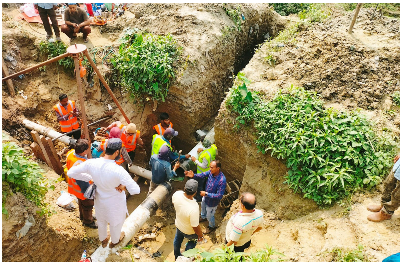
Hook-up activities to supply gas to New DRS by BGDCL
