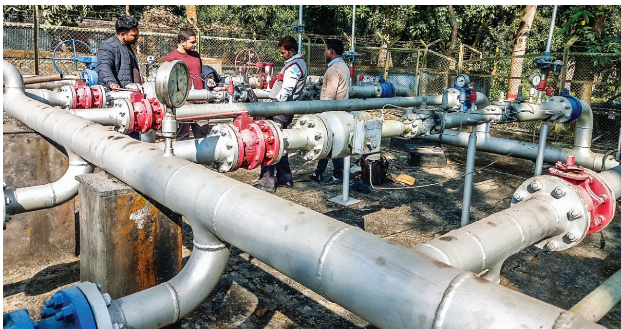
Habiganj DRS Regulator maintenance works by JGTDSL
