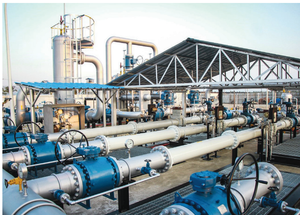
Anowara Citygate Station, Chattogram of GTCL
