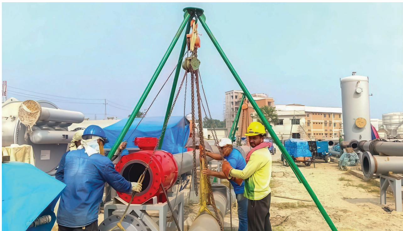
Under construction Rupsha 800 MW CCPP RMS in Khalishpur, Khulna by SGCL
