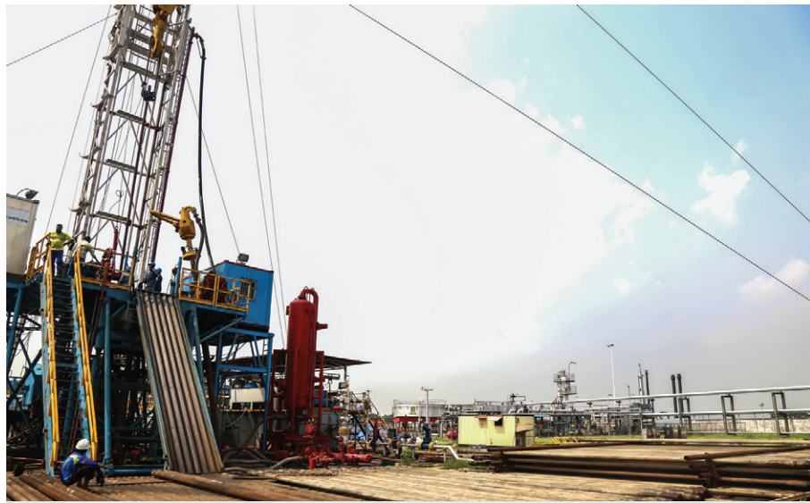
Workover of Titas-24 well by BGFCL
