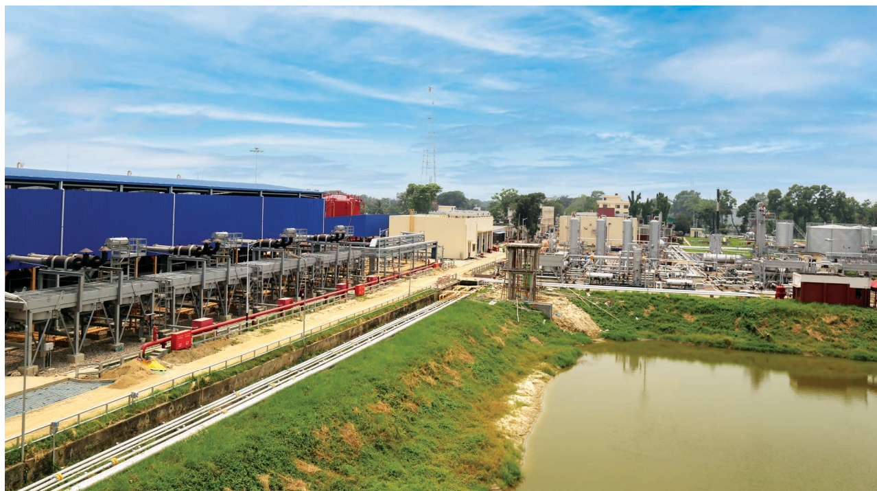
7 nos. wellhead compressors at Titas-A of BGFCL
