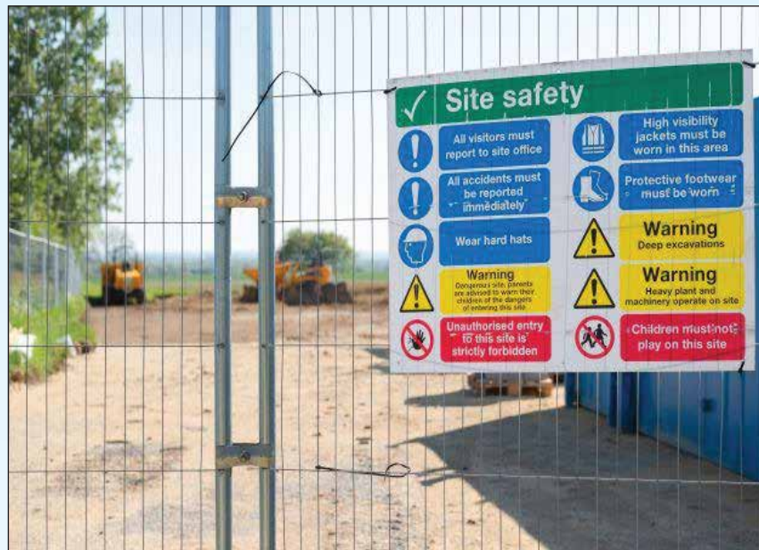
Pic 3. Site safety signs and symbols display
