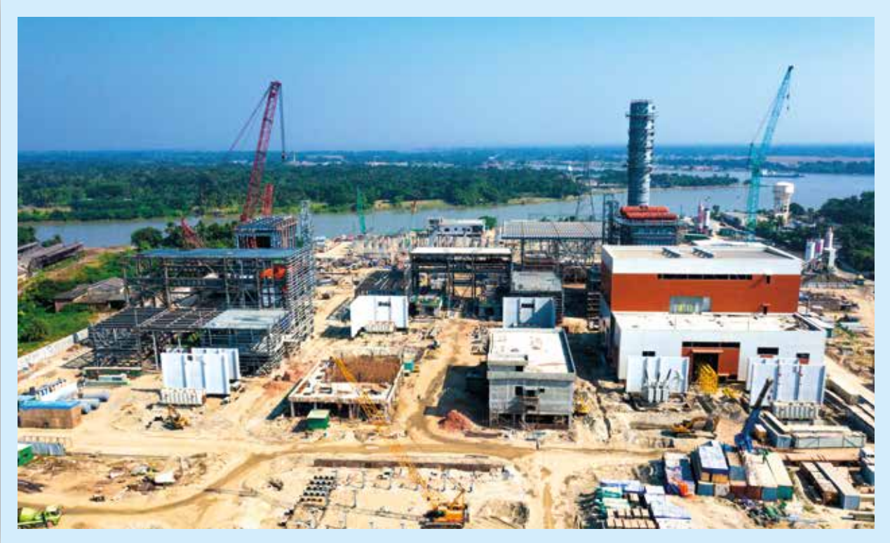
Construction work of Rupsha 800 MW Combined Cycle Power Plant Project
