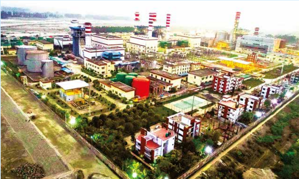
Sirajganj Power Generation Hub (Unit:1, 2, 3 & 4)
