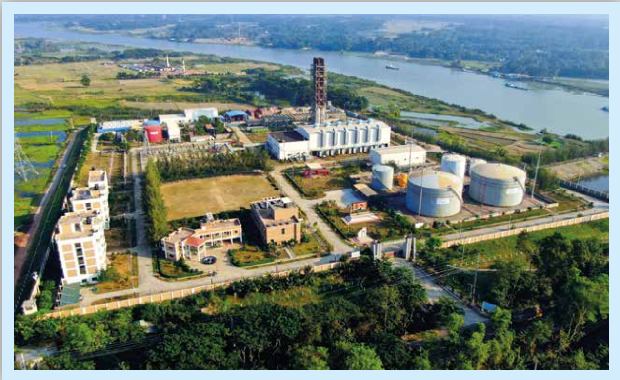
Madhumati 100 MW HFO Power Plant
