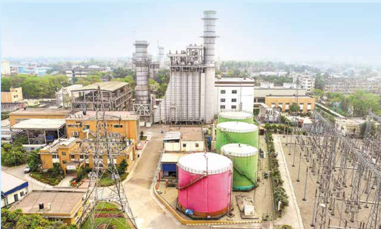
Khulna 225 MW Combined Cycle Power Plant
