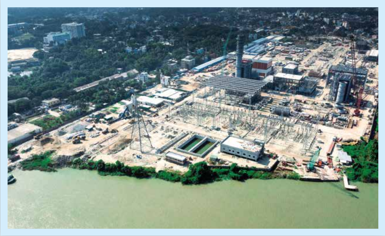
Rupsha 800 MW Combined Cycle Power Plant Project
