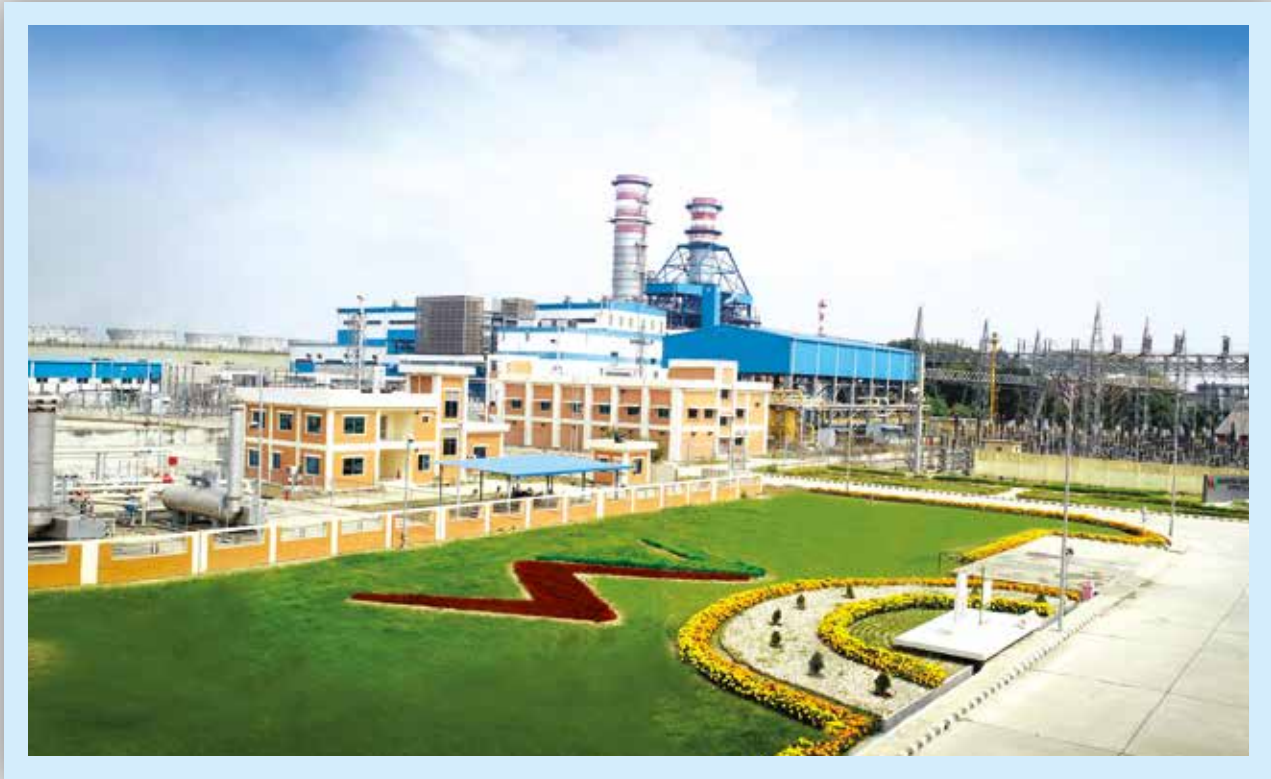
Bheramara 410 MW Combined Cycle Power Plant
