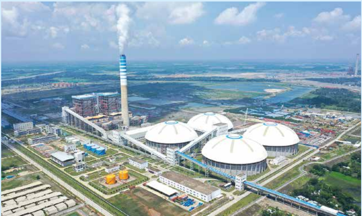
Payra 1320 MW Thermal Power Plant (1st Phase) (Under JVC)
