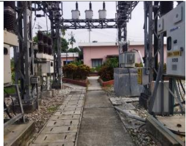
South (Control Room)
