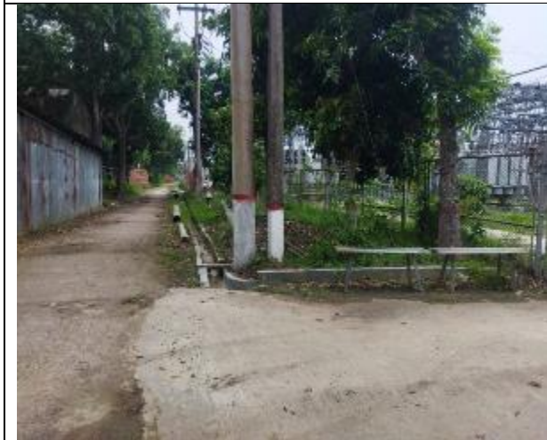
East (Access Road & Substation)
