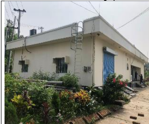
North (Nesco Control room & quarter building)
