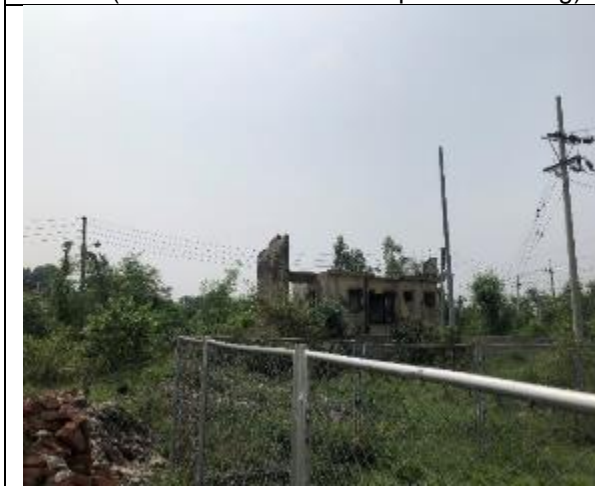
East (Abandon quarter building, Fellow land)
