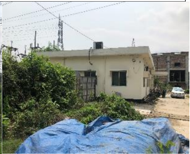
West (Nesco control room)
