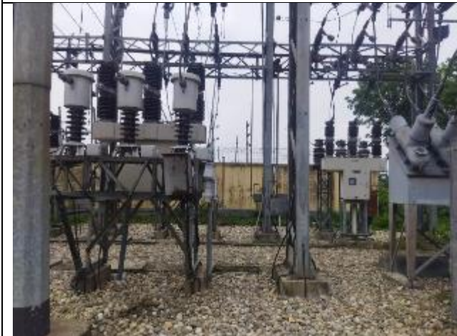
East (Substation & Access Road)
