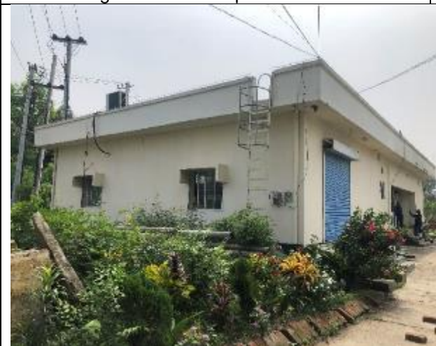
Existing Unaffected Structure
