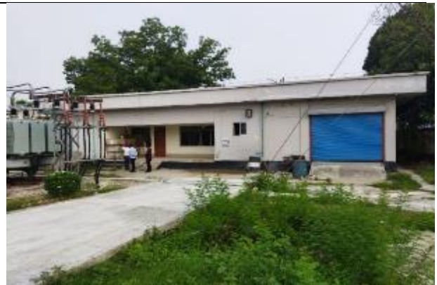
South (NESCO Control room)
