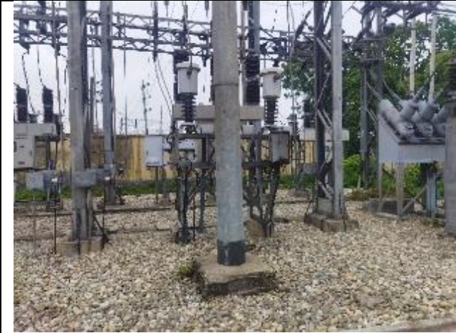
Existing substation/ Proposed bay station
