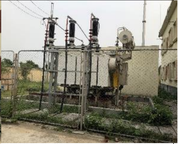
Existing substation/Proposed Renuvation
