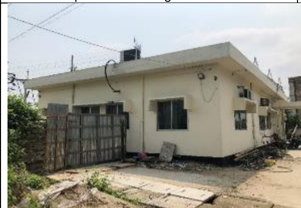
Existing Structure Picture
