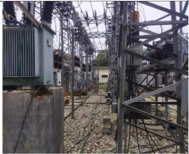
West (Control room & Existing Substation)
