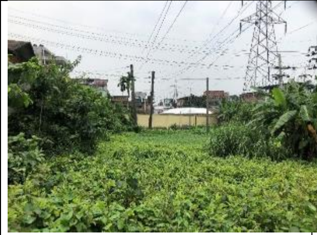
Proposed switching and bay station
