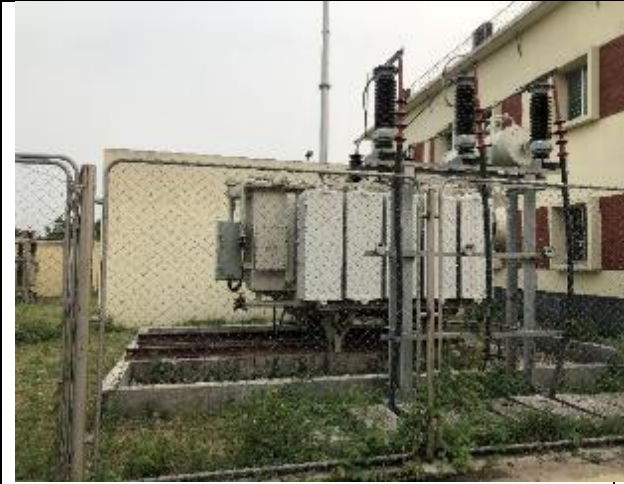
Existing substation/Proposed Renovation
