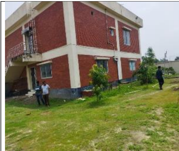
North (Control room)
