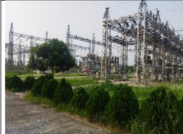
Existing Substation/Proposed bay station
