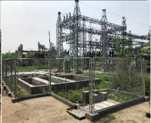
Existing substation/ Proposed Renovation
