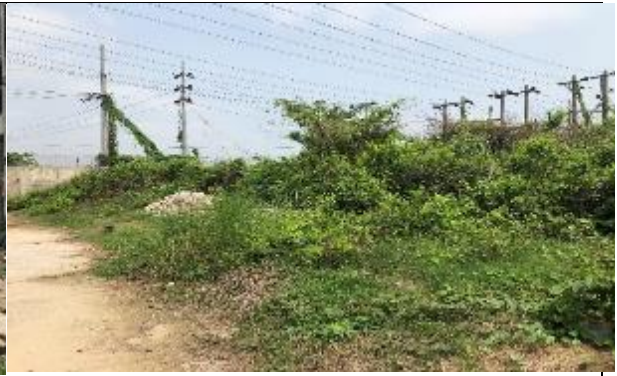
Proposed substation picture
