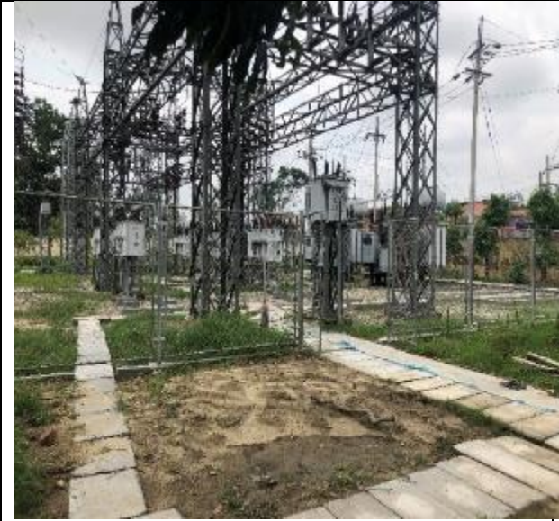
Existing substation/Proposed Renovation
