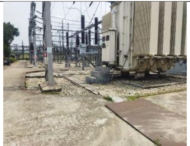
South (PGCB Building)
