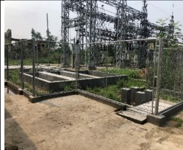
Existing substation/Proposed Renovation
