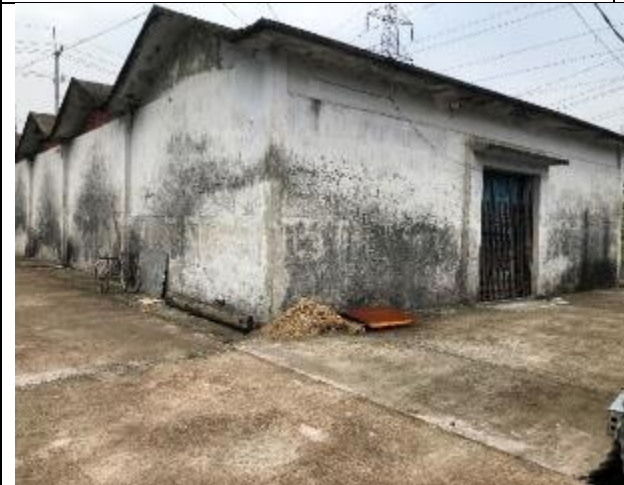
Existing Structure picture
