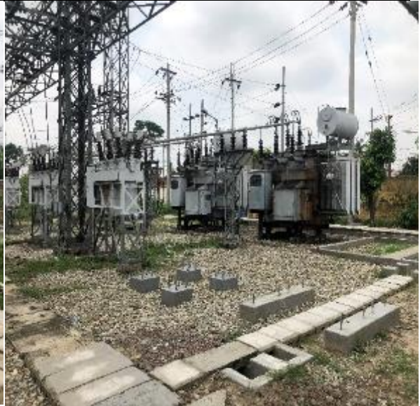
Existing substation/ Proposed Renuvation
