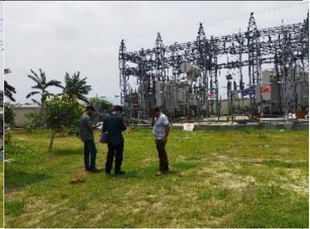
Existing Substation/ Proposed bay station
