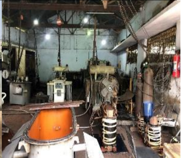
Existing workshop picture
