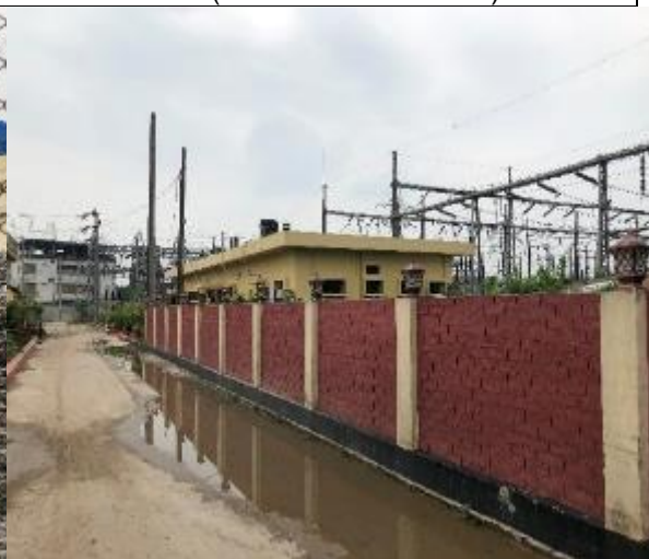
West (PGCB sub station)
