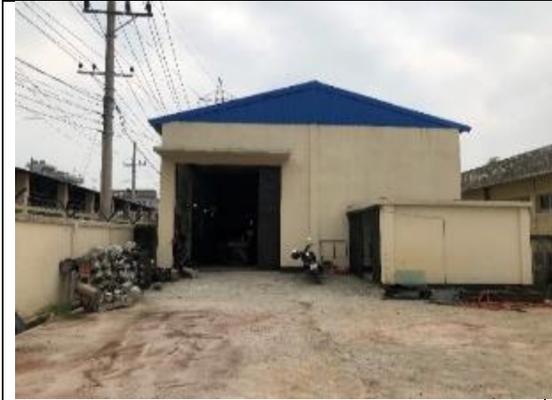
Existing Workshop picture
