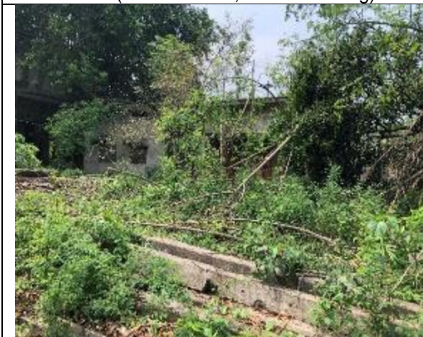
East (Nesco Abandon Building)
