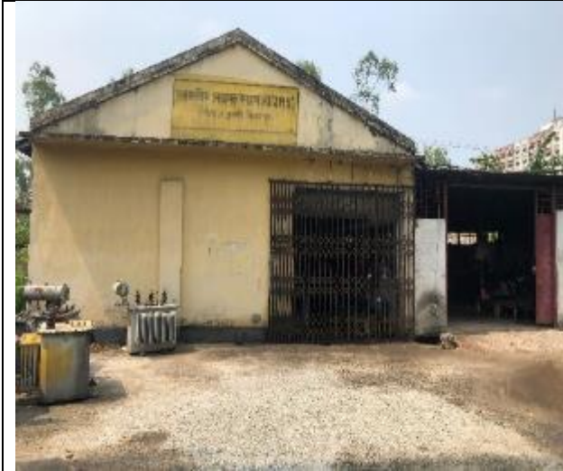
Existing workshop picture
