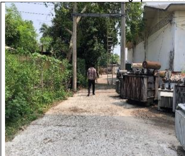
North (Access Road, Nesco building)
