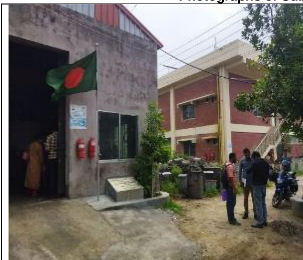
North (Work shop and Control room)
