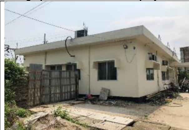
Existing Structure Picture
