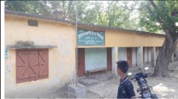
Char Nowshera Government Primary School and High School, Asariadhaho; Alaituli, Godagari, Rajshahi.
