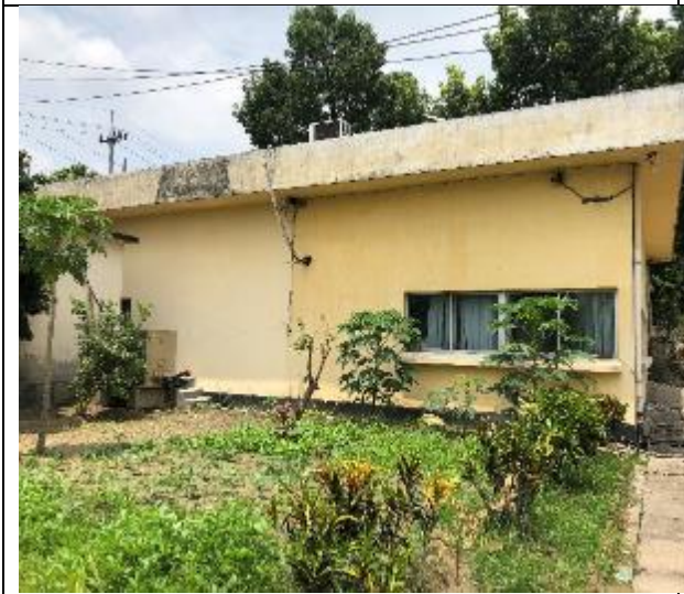
Existing Structure picture
