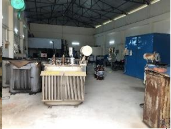
Existing Workshop picture
