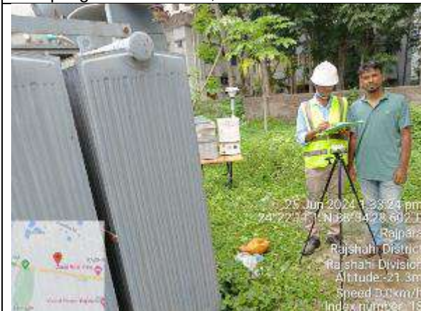
Fig: ANL-02, (Day Time) Chandipur Substation Area, Rajshahi GPS Co-Ordinate: 24°22'11.17"N; 88°34'28.47"E Sampling Date: June 25, 2024
