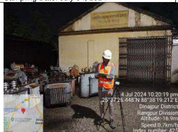
Fig: ANL-15, (Night Time) S&D-2, Workshop Area, Dinajpur GPS Co-Ordinate: 25°37'26.52"N; 88°38'19.34"E Sampling Date: July 04, 2024
