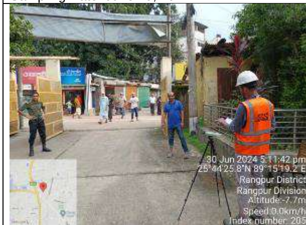
Fig: ANL-08, (Day Time) S&D-1 Campus, Substation Area, Rangpur GPS Co-Ordinate: 25°43'43.24"N; 89°15'8.33"E Sampling Date: June 30, 2024
