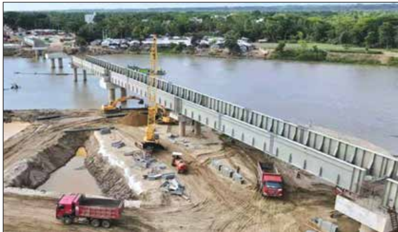
Girder erection of Bridge No. 3 over Sangu River under "Construction of Single Line Dual Gauge Railway Track from Dohazari to Cox's Bazar via Ramu and Ramu to Gundum near Myanmar" Project.
