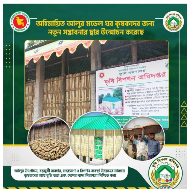
Figure 4-2: Refrigerant Free Potato Cold Storage by Natural Cooling
