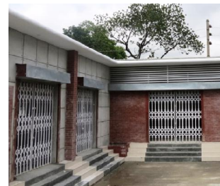
3. Generator & Power Station Building
