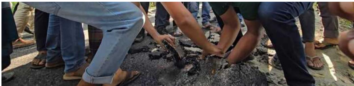
Figure 2 Weak prime coating can lead to debonding at low stress
