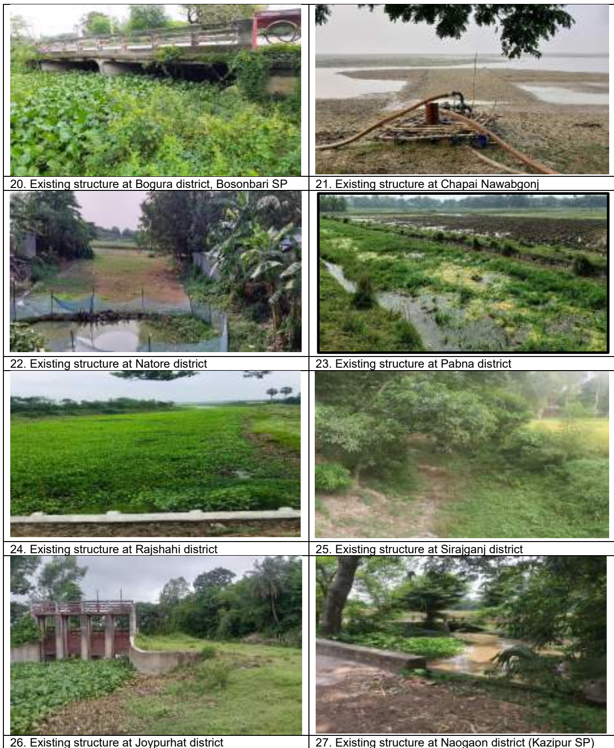
Photo plate 4: Photographs of Existing structure of SP in Districts of Rajshahi Division
