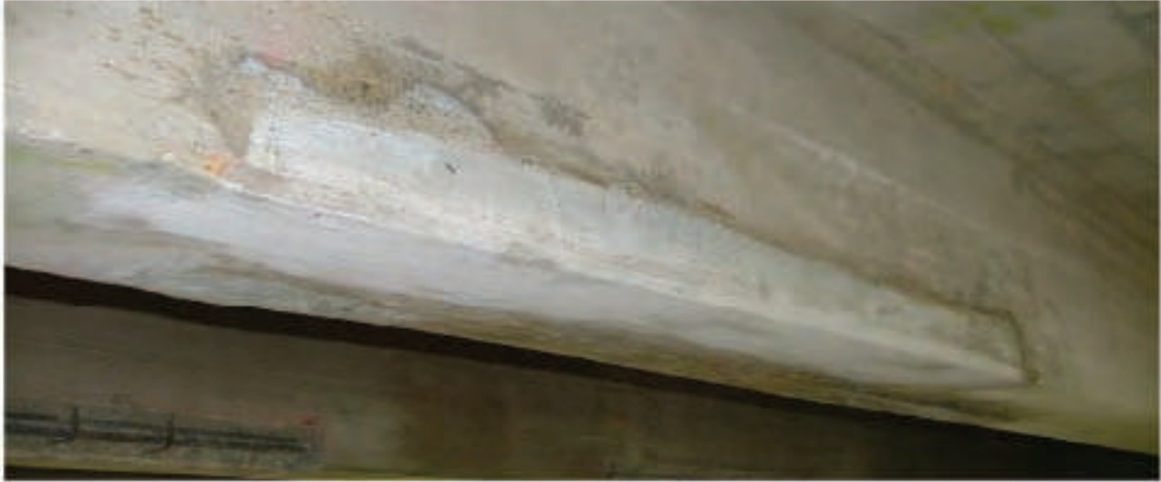
Figure 9.9: Completed Form Repair
