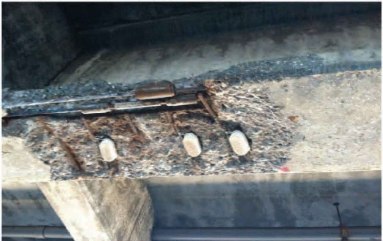
Figure 9.5: Concrete Super-structure Ready for Patch
