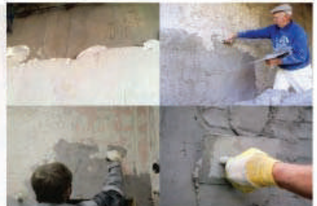
Figure A.8.9: Figure: Plastering for different concrete surface
