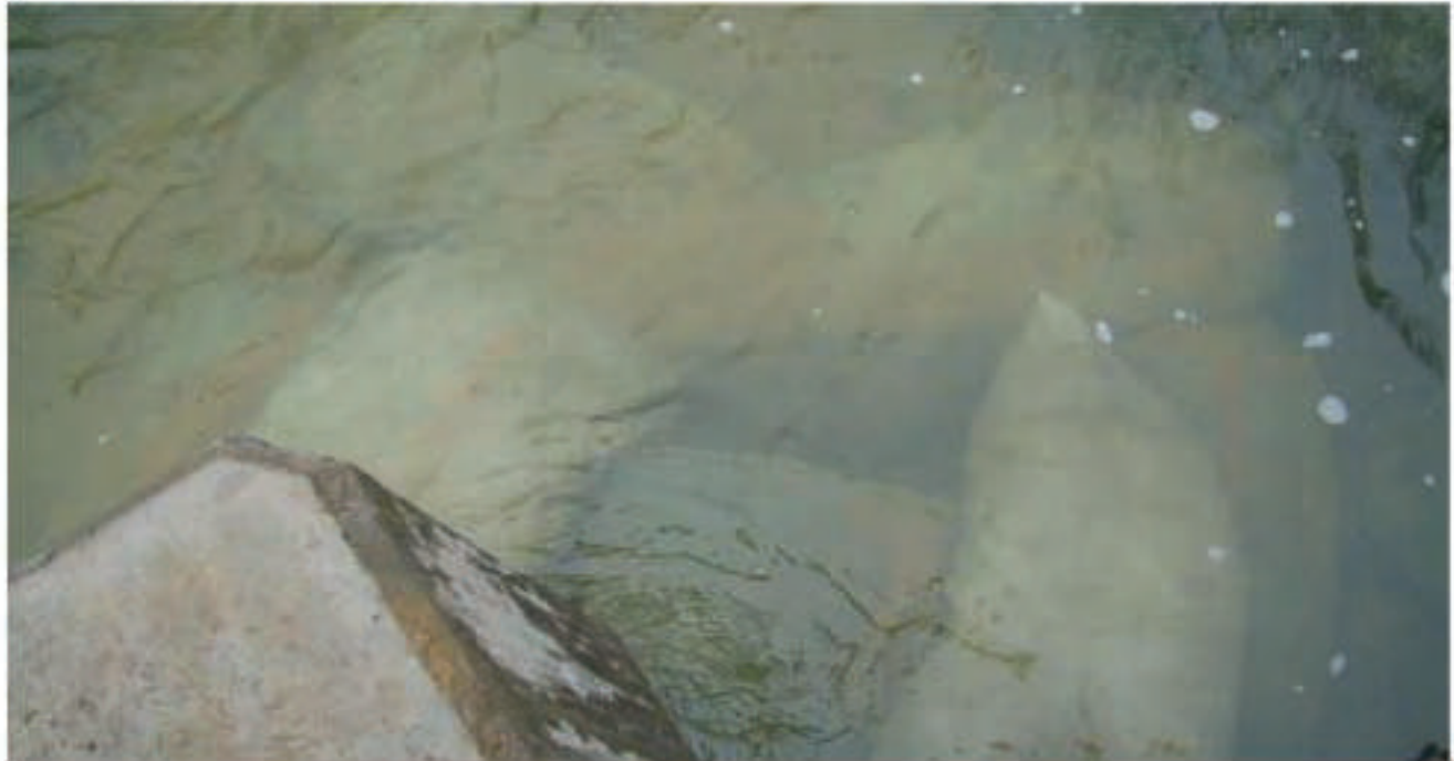
Figure 10.26: Grout Bags Used to Prevent Undermining
