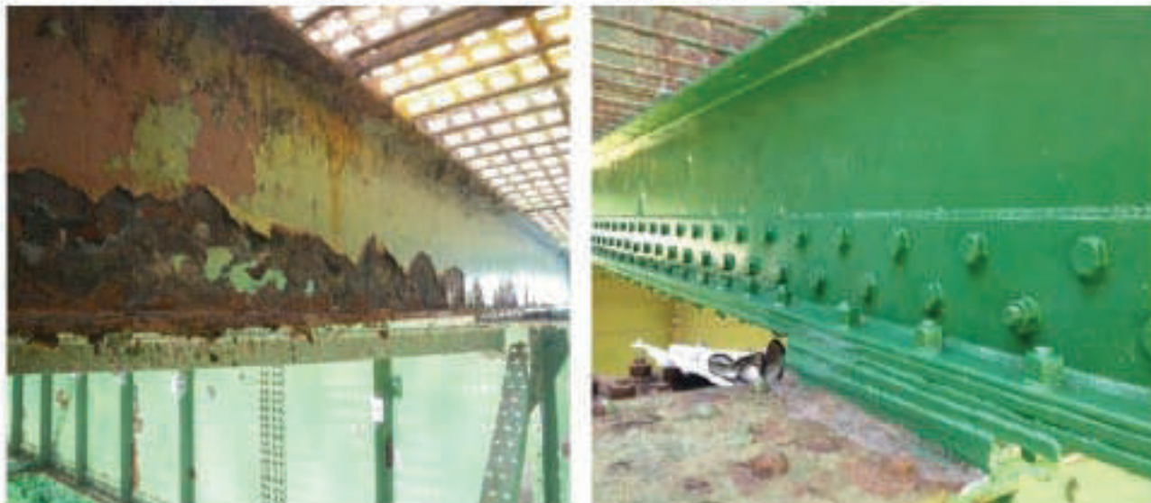
Figure 9.29: Girder Repair. Before (left) and After (right).
