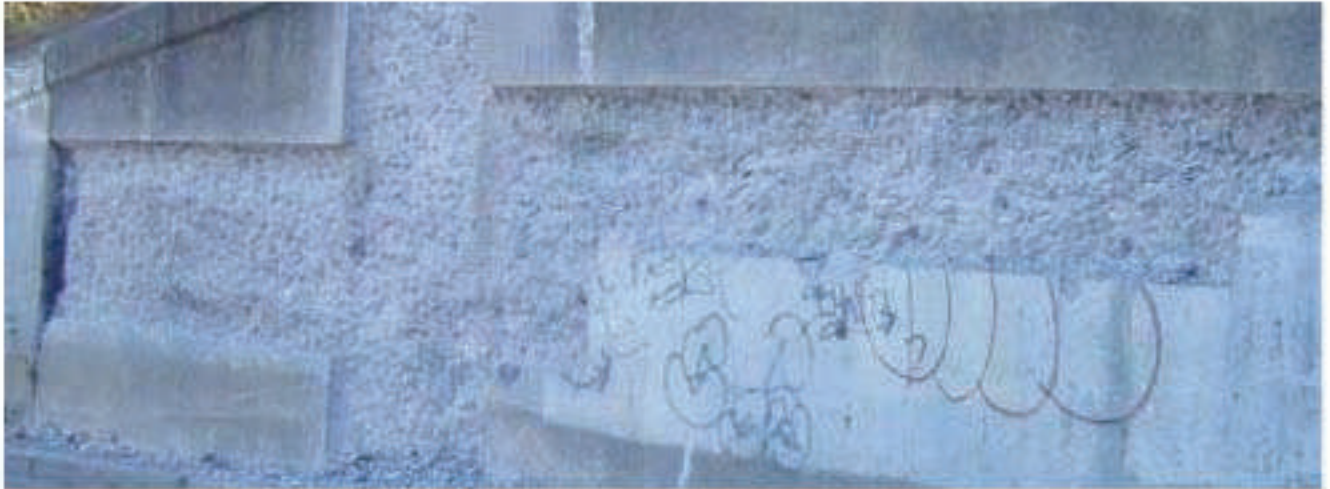
Figure 10.10: Preparation for Repair of Retaining Wall
