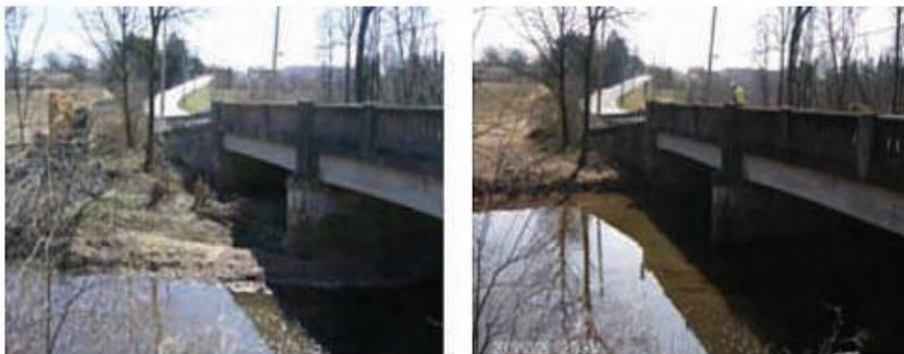
Figure 11.11: Deposited Sediment Removal to Maintain Hydraulic Opening (a) Before, (b) After
