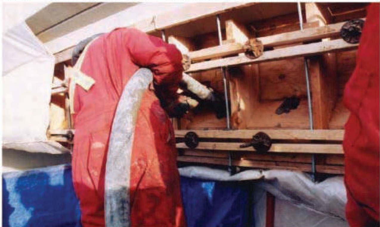
Figure 9.8: Forming Repair. Pumping Concrete into the Form
