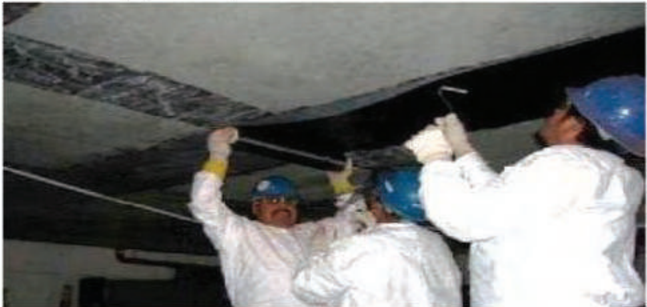
Figure 9.16: Applying FRP to Strengthen a Beam
