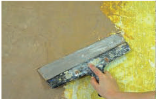
Figure A.8.6: Application of Patching compound
