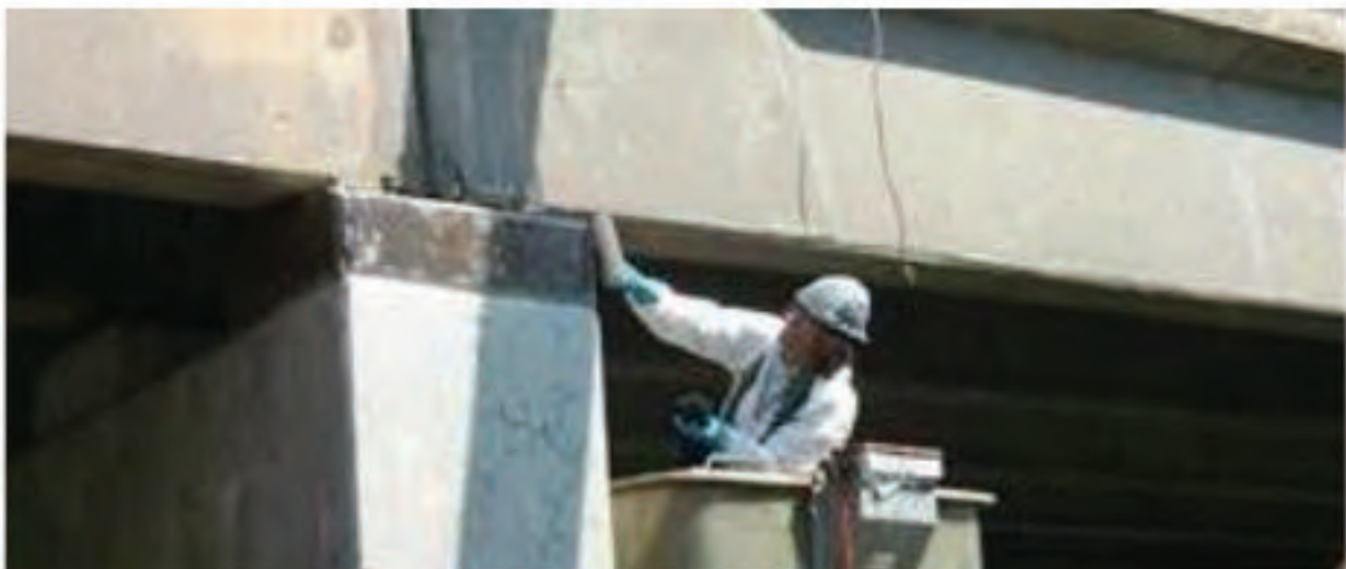
Figure 10.36: Pedestal Repair with FRP
