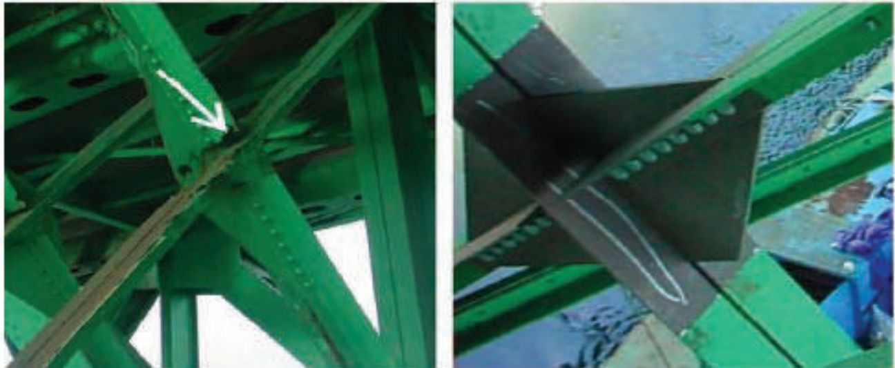
Figure 9.32: Replacement of Bracing and Connection Plate. Before (left) and After (right)
