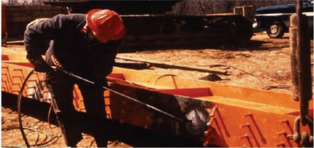
Figure 9.50: Example of Heat Straightening Procedure
