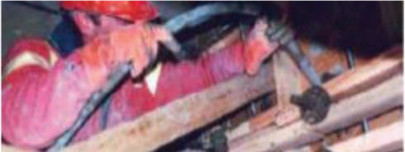
Figure 10.47: Pouring concrete
