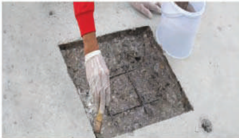
Figure A5.4: Preparation of Concrete Deck for Application of Polymer Concrete
