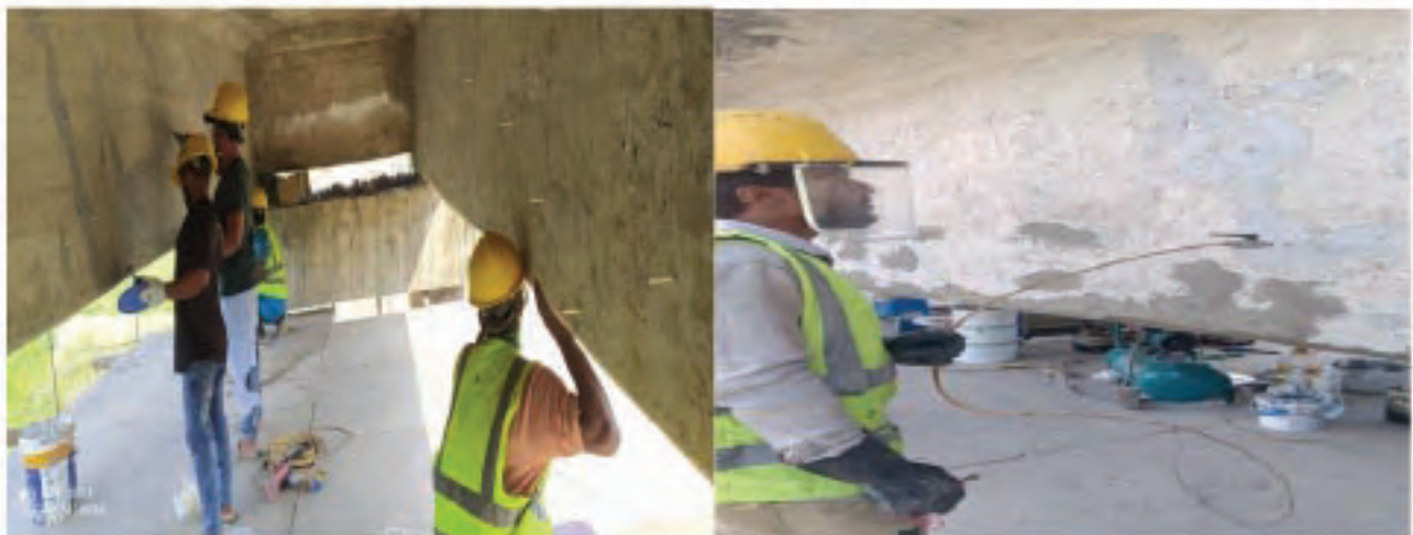
Figure A4.3: Injection of Epoxy to fill the Cracks
