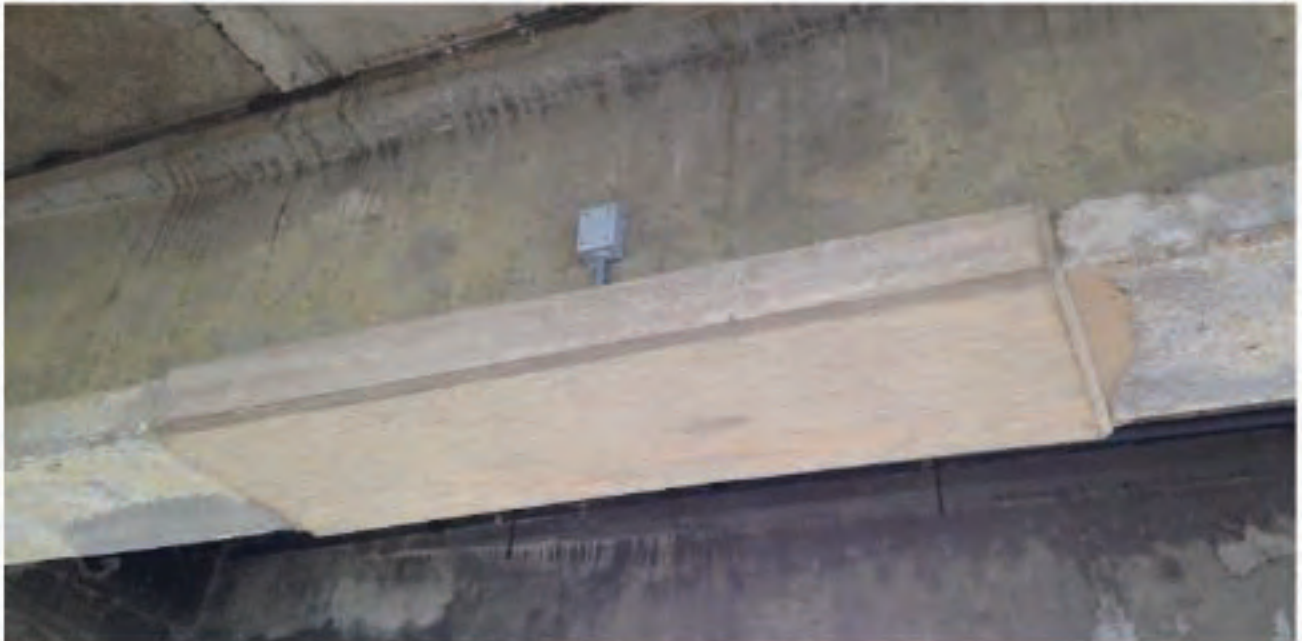
Figure 9.6: Concrete Super-structure with Wood Form
