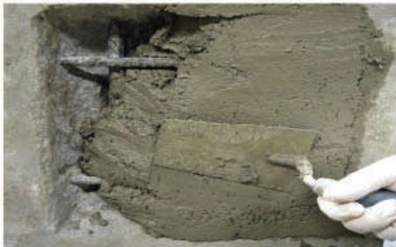
Figure A5.5: Application of Polymer Concrete
