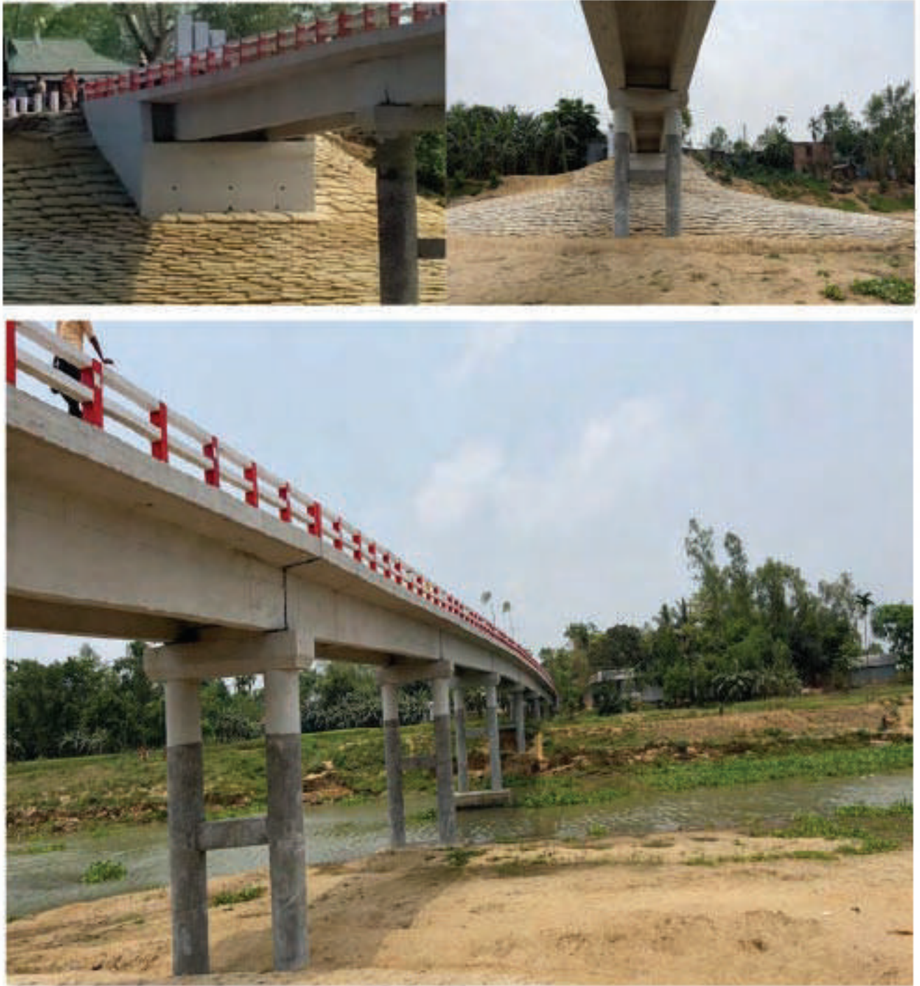
Figure A7.7: Rehabilitated Bridge
