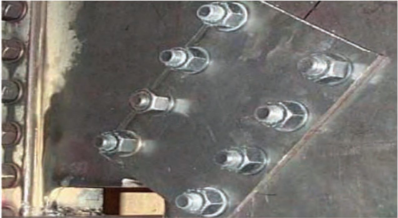
Figure 9.46: Example of Reinforcement Plate Repair
