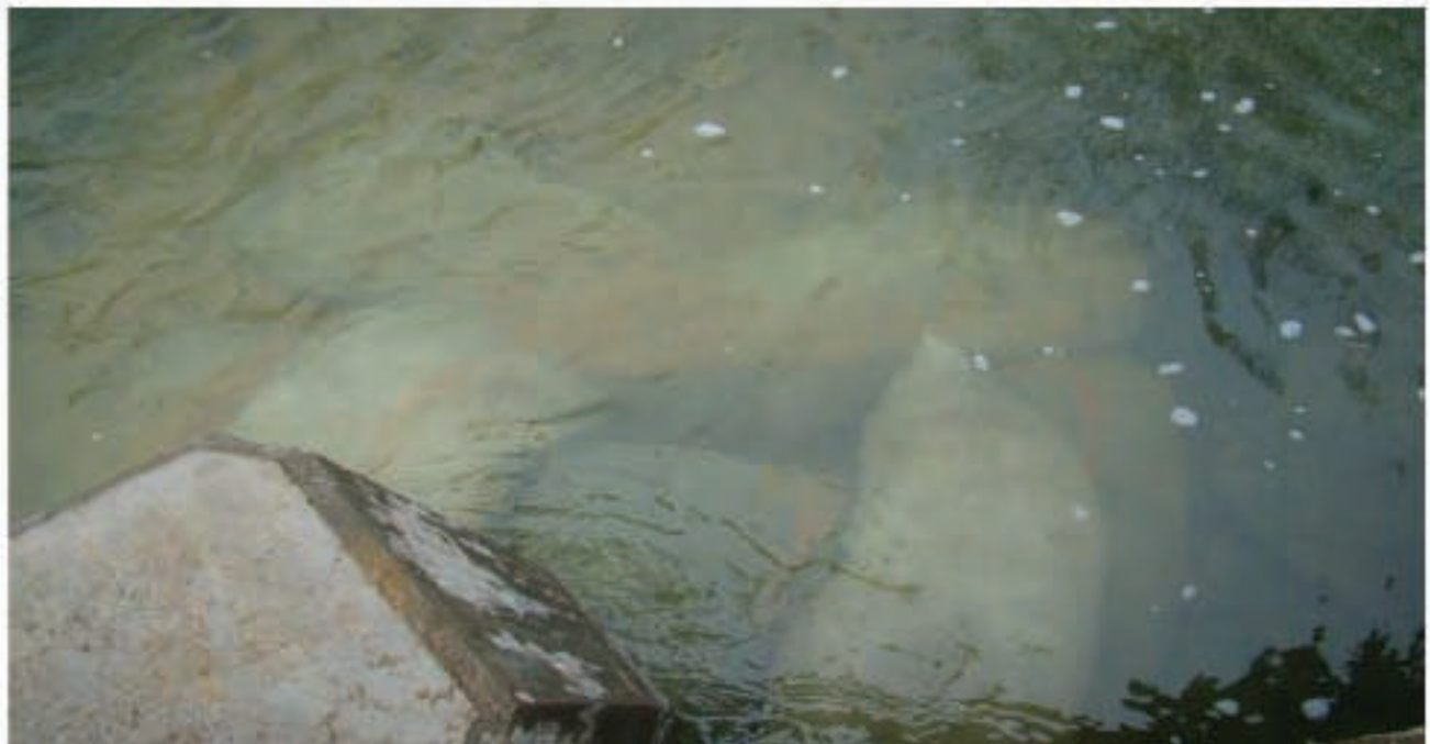
Figure 11.23: Grout Bags Installed around a Pier Nose
