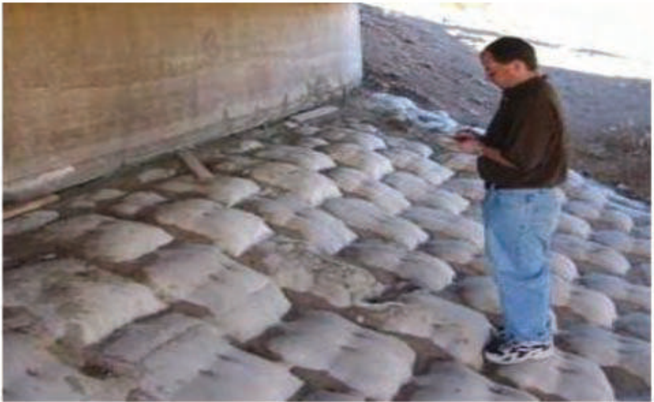
Figure 11.24: Grout-Filled Mat Used for Scour Protection at a Bridge Abutment
