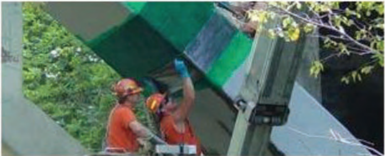
Figure 10.35: Strengthening a Spandrel Arch with FRP
