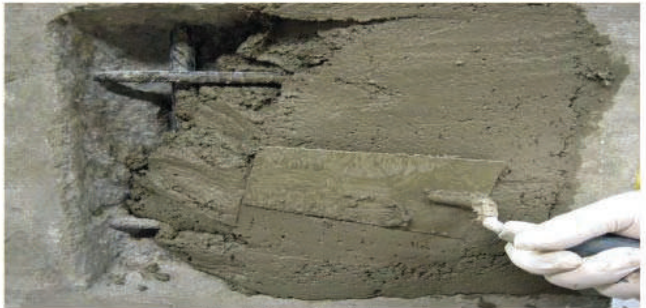
Figure 10.46: Application of polymer mortar
