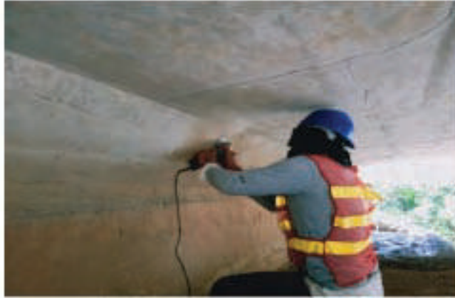
Figure A.8.4: Surface preparation for Skim coat treatment slab
