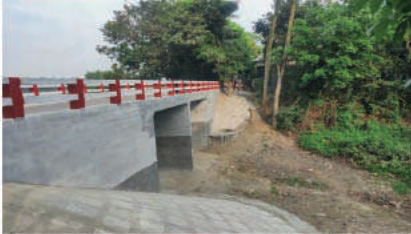
Figure A5.3: Culvert repair using Polymer Mortar
