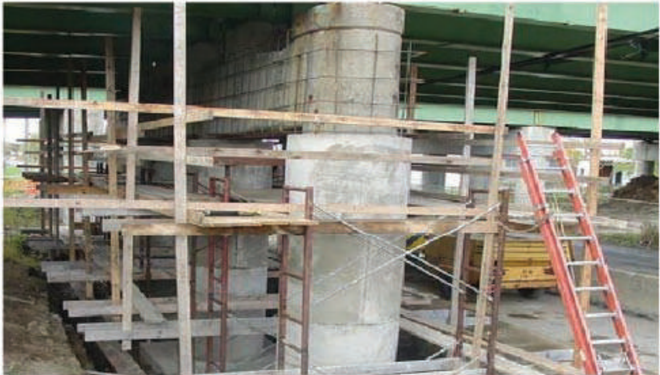
Figure 10.9: Non-Structural Repair of a Column
