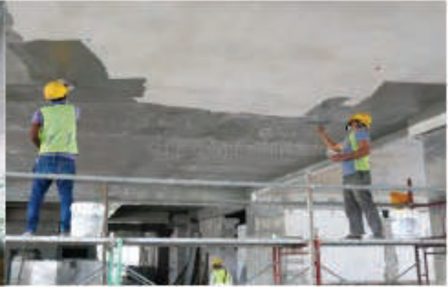
Figure A.8.5: Skim coat application in Ceiling or bottom of deck slab
