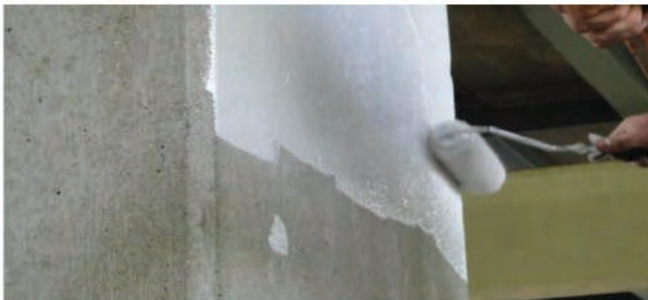
Figure 10.4: Protective Coating Applied on the Sub-structure
