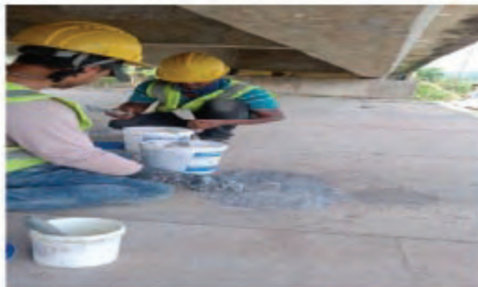
Figure A4.2: Mixing of Epoxy material
