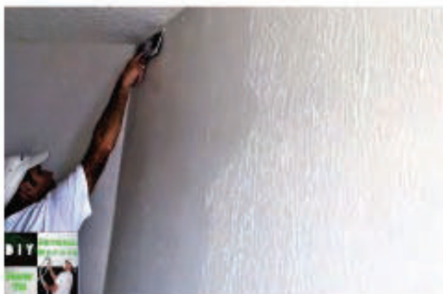
Figure A.8.8: Skim coat application
