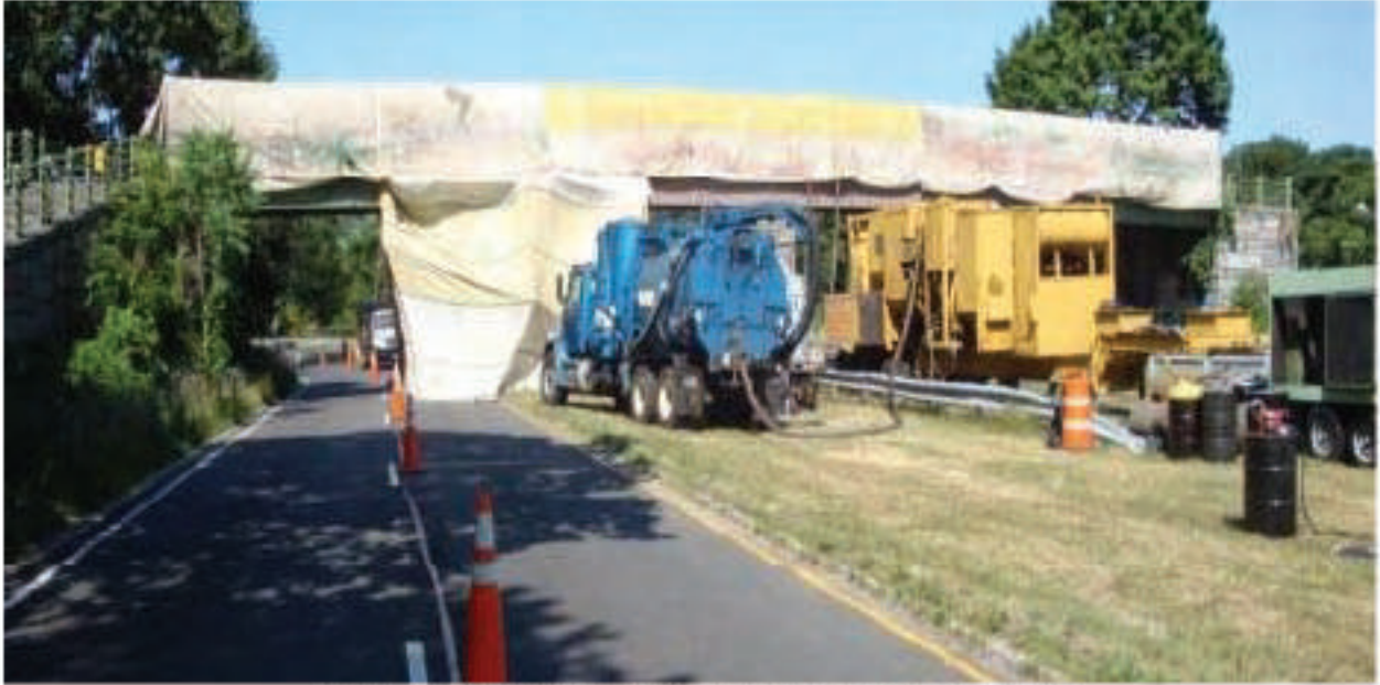
Figure 9.22: Painting Project with Approved Containment System
