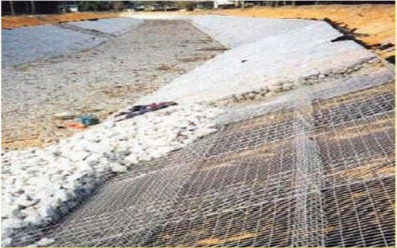
Figure 11.18: Field Installation of Gabion Mattresses on Channel Bed and Banks
