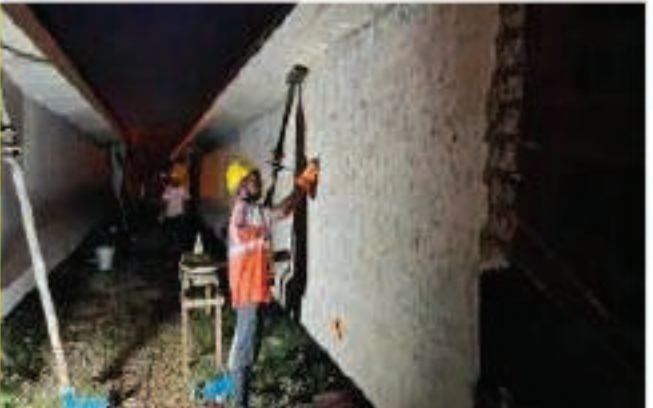
Figure A.8.7: Surface voids repairing
