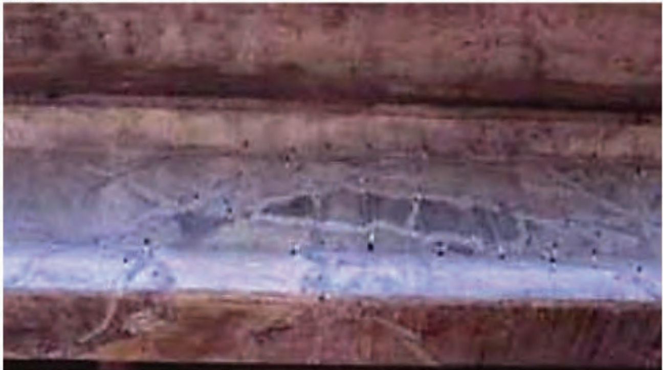
Figure 9.12: Completed Epoxy Crack Repair
