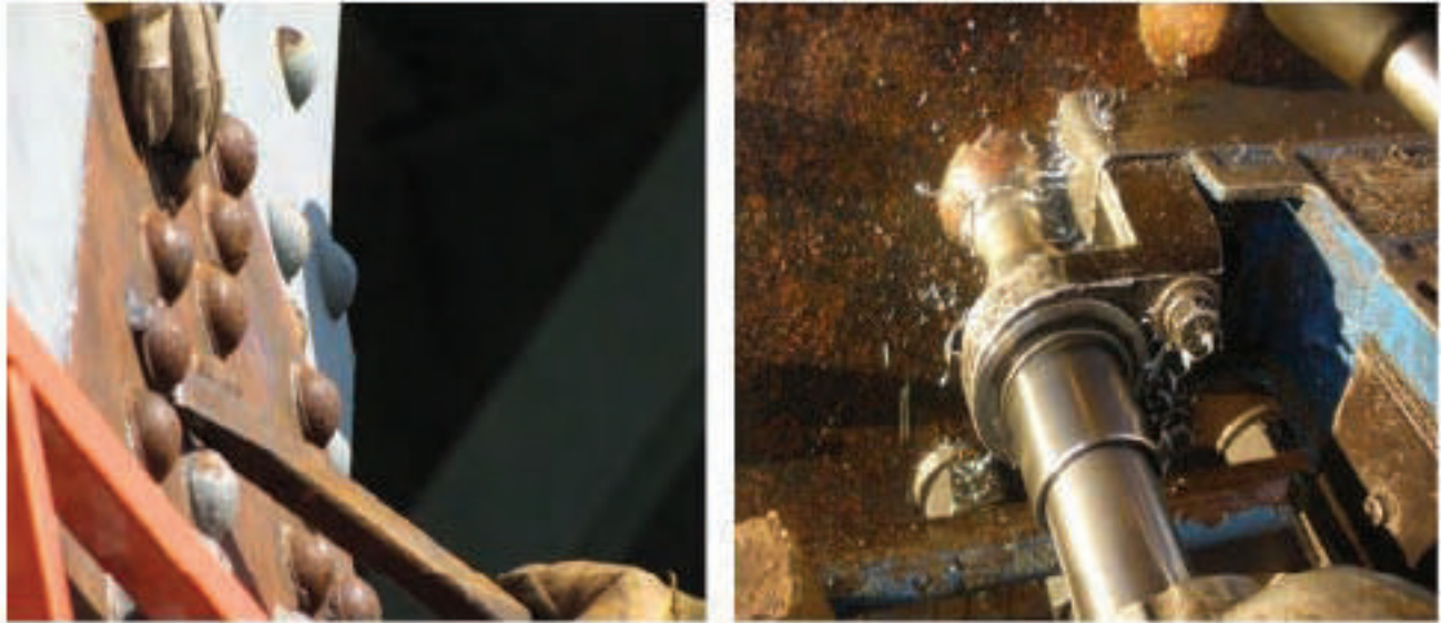
Figure 9.41: Rivet Removal. Pneumatic Rivet Breaker (left) and Drill Removal (right)
