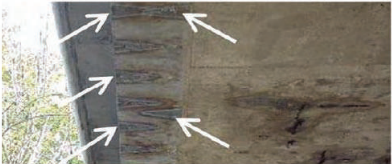
Figure 9.51: Nearly Completed Girder Repair Made Utilizing Heat Straightening
