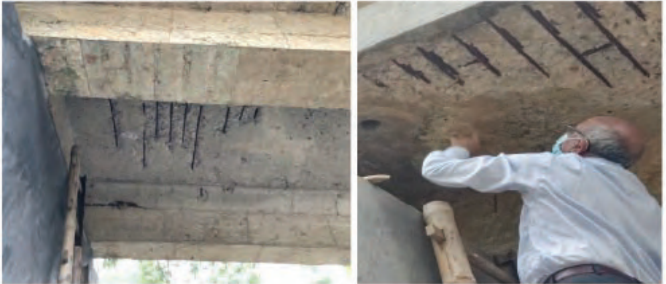
Figure 10.43c: Surface condition of bottom slab – suitable for polymer application
