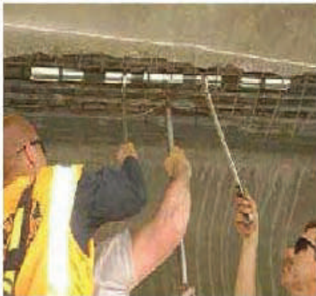
Figure 9.19: Tensioning the Splice
