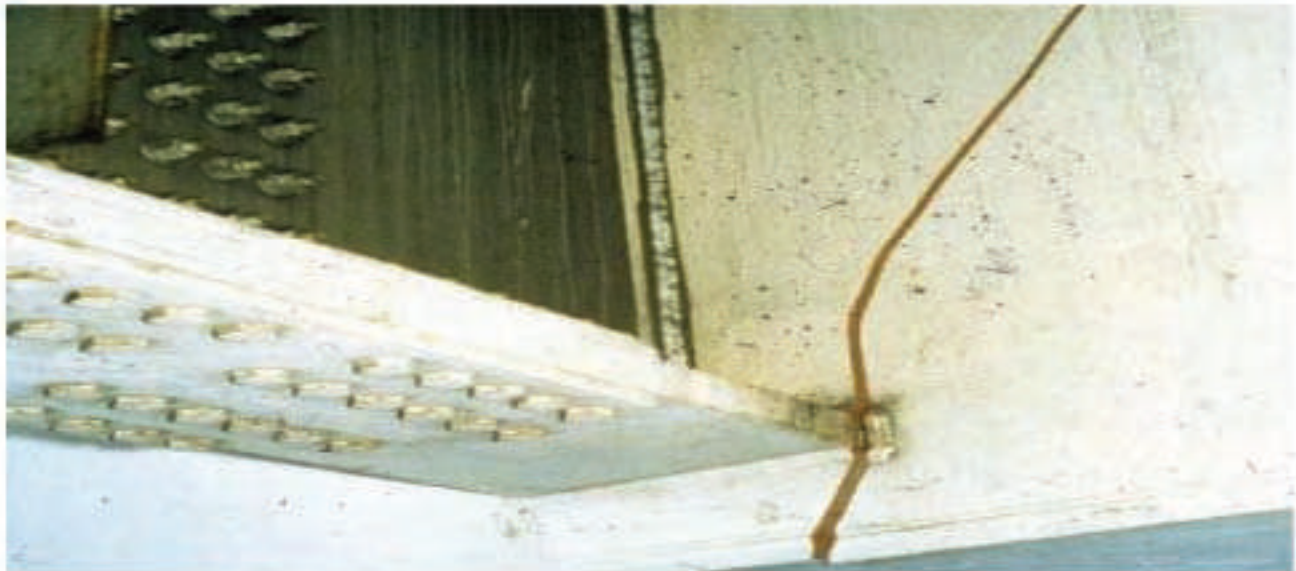
Figure 9.42: Fatigue Crack
