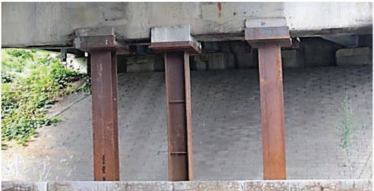
Figure 10.60: Temporary Steel Shoring used to Support Deteriorated Concrete Pier Cap
