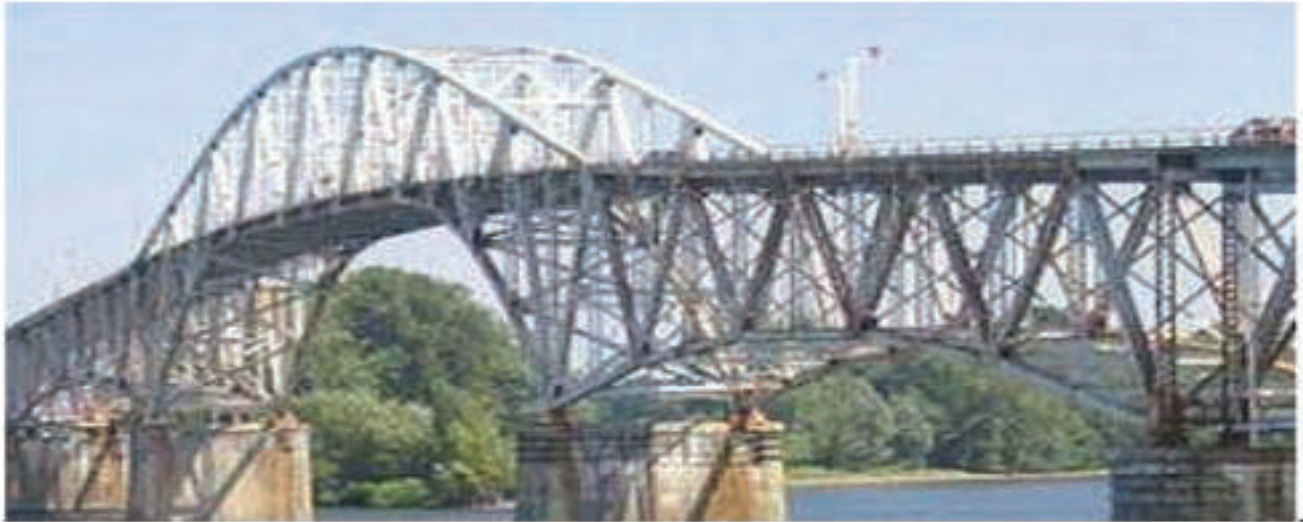
Figure 10.38: External Post-Tensioning Rods used in Pier Containment
