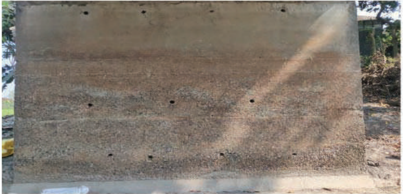
Figure A5.1: Detreated (scaled) Abutment Surface
