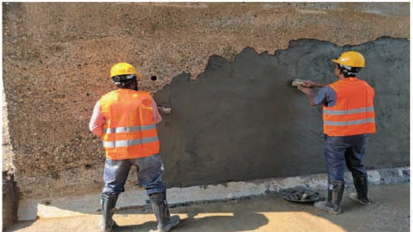
Figure A5.2: Application of Polymer Mortar
