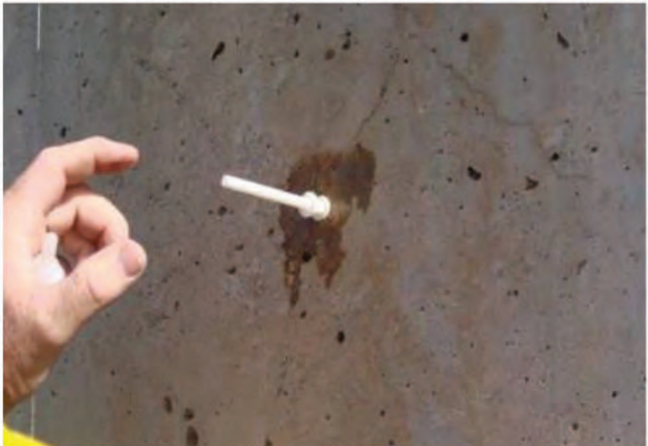
Figure 10.19: Installation of Epoxy Injection Ports (Courtesy of MDOT)
