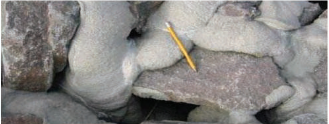
Figure 11.20: Close-Up View of Partially Grouted Riprap
