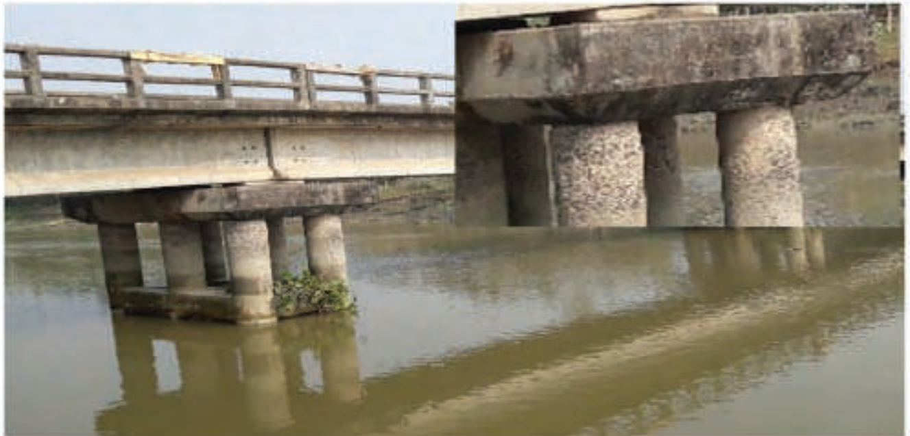
Figure 10.43b: Surface condition – suitable for polymer application
