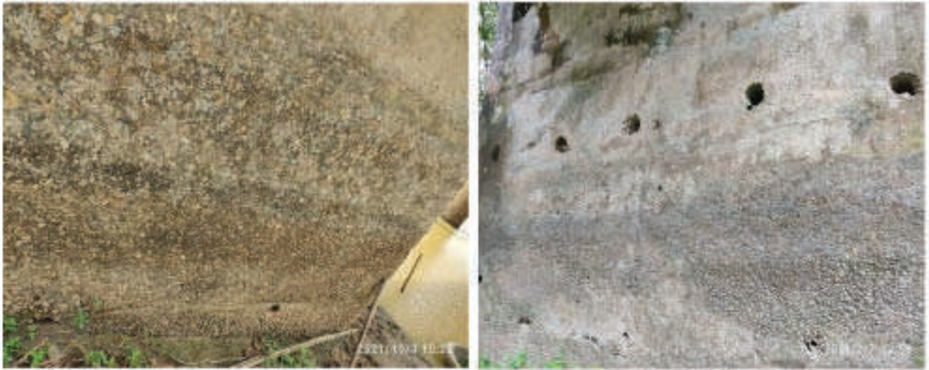
Figure 10.43a: Surface condition – suitable for polymer application
