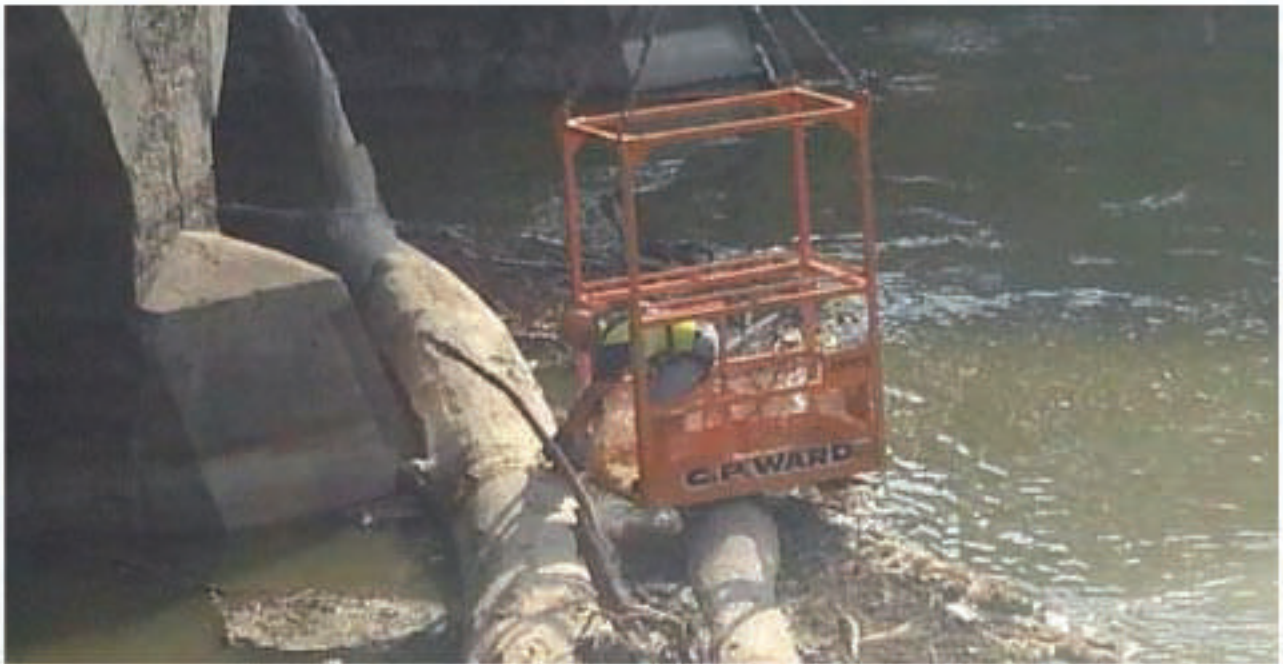
Figure 11.7: Debris Removal Operation
