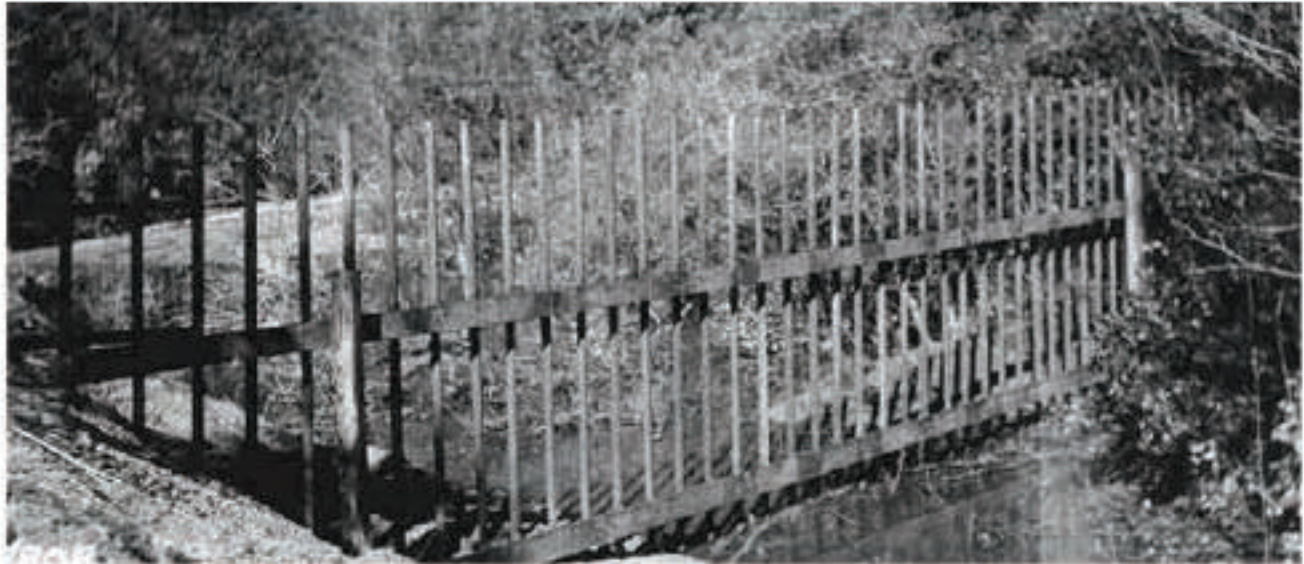
Figure 11.9: Post and Rail Debris Rack Installed 100 Feet Upstream of Culvert
