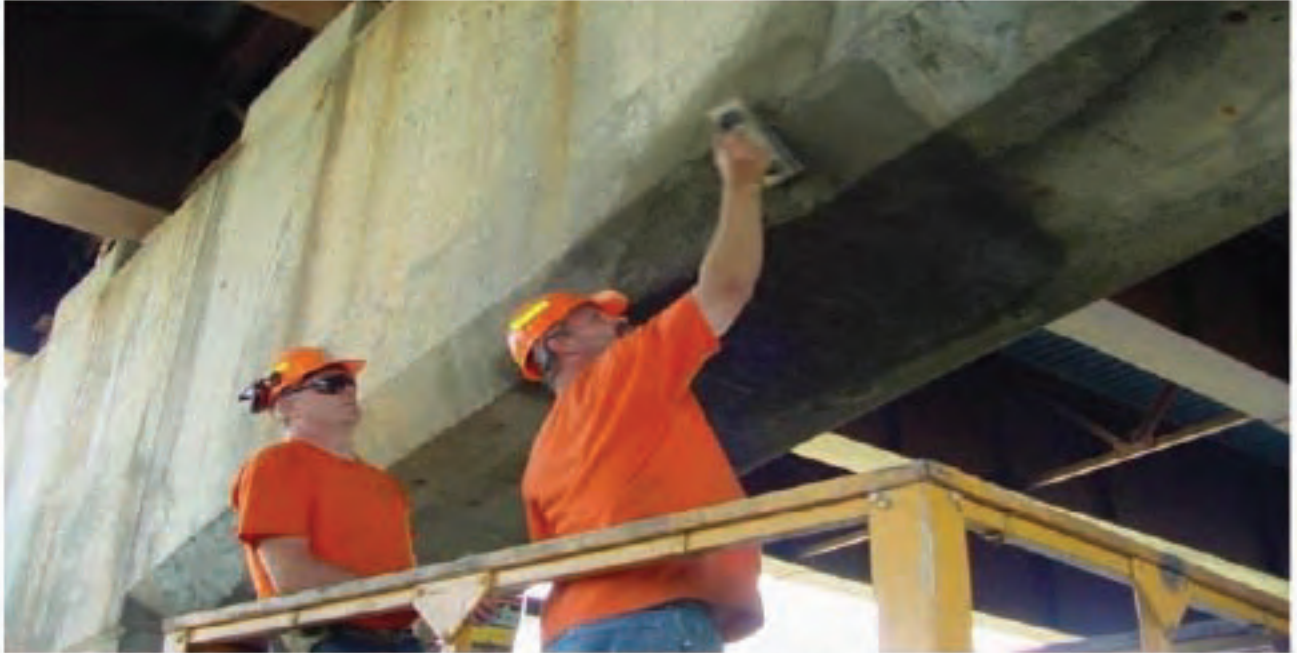
Figure 9.4: Patching of Concrete Super-structure
