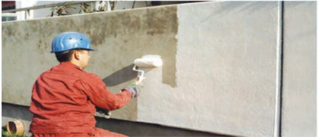
Figure A.8.13: Painting on railing
