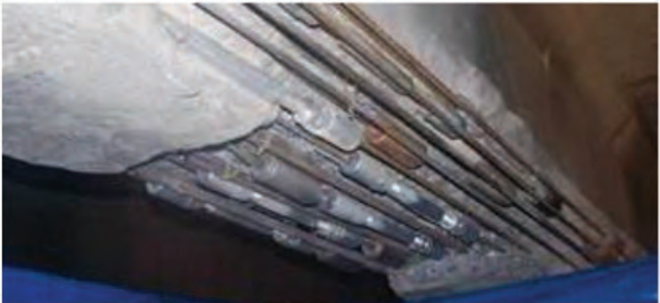
Figure 9.21: Completed Strand Coupling System in Prestressed Girder Repair
