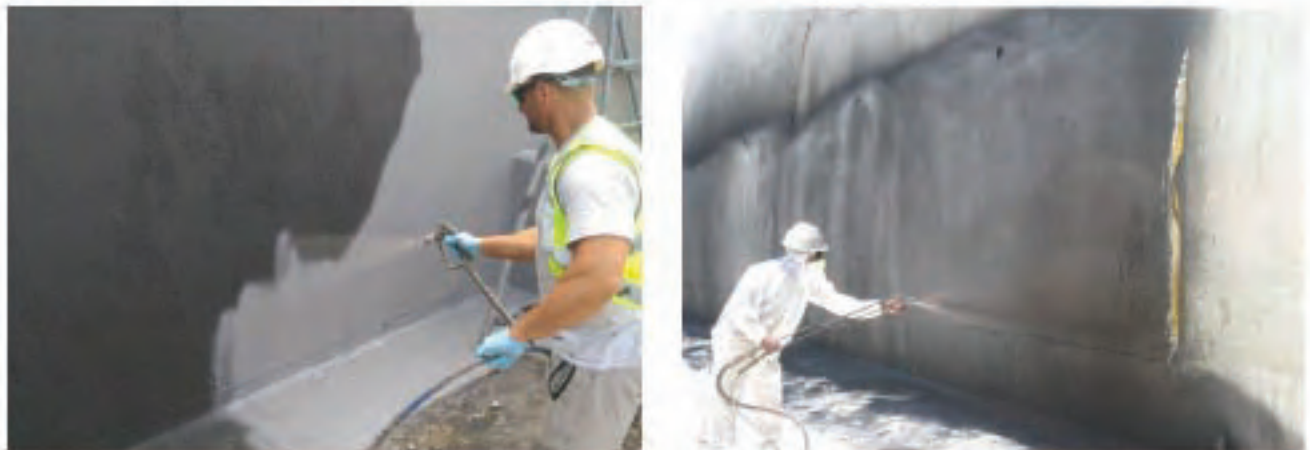
Figure A.8.11: Applying water Proofing materials in abutment wall
