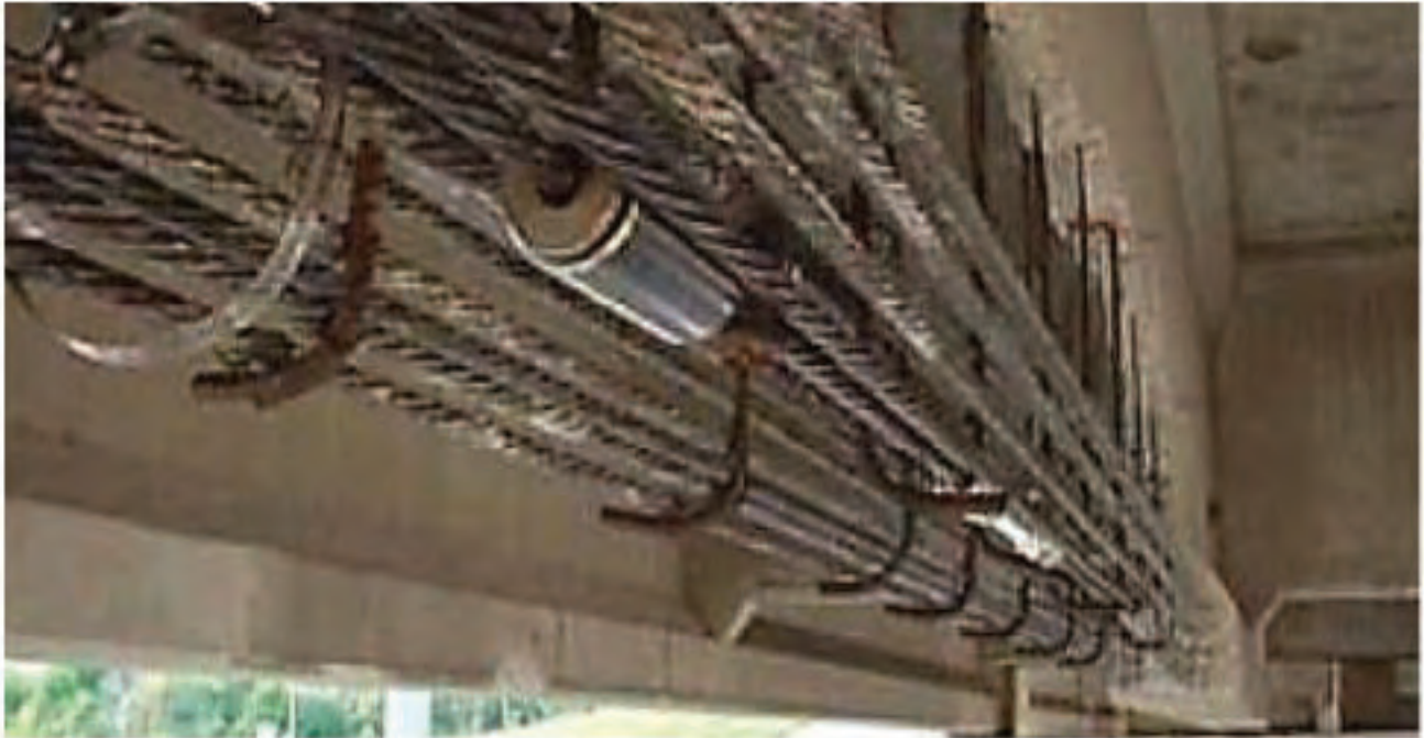
Figure 9.20: Completed Splice Ready for Concrete
