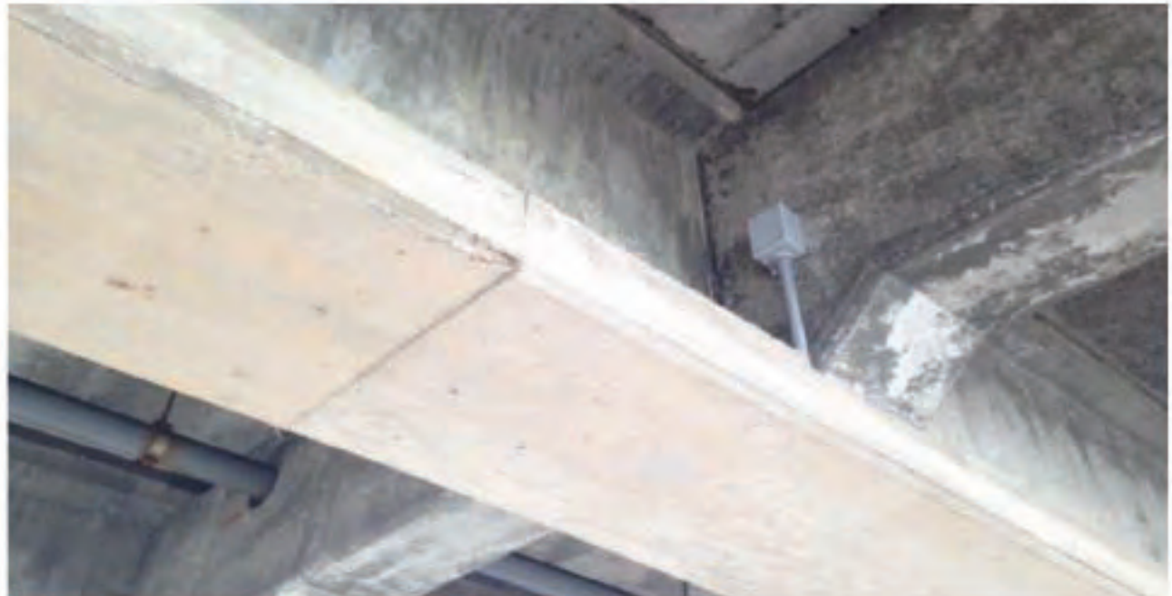
Figure 9.7: Completed Repair of Concrete Superstructure
