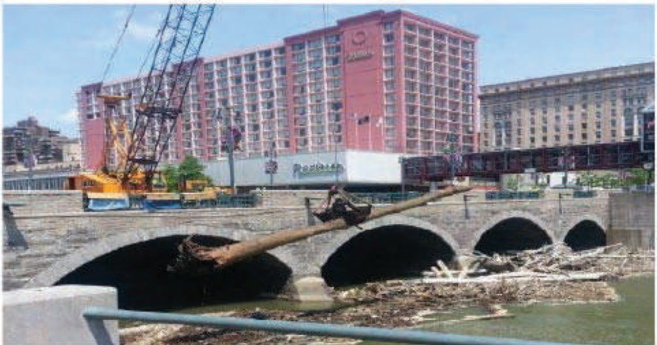
Figure 11.8: Debris Removal Operation
