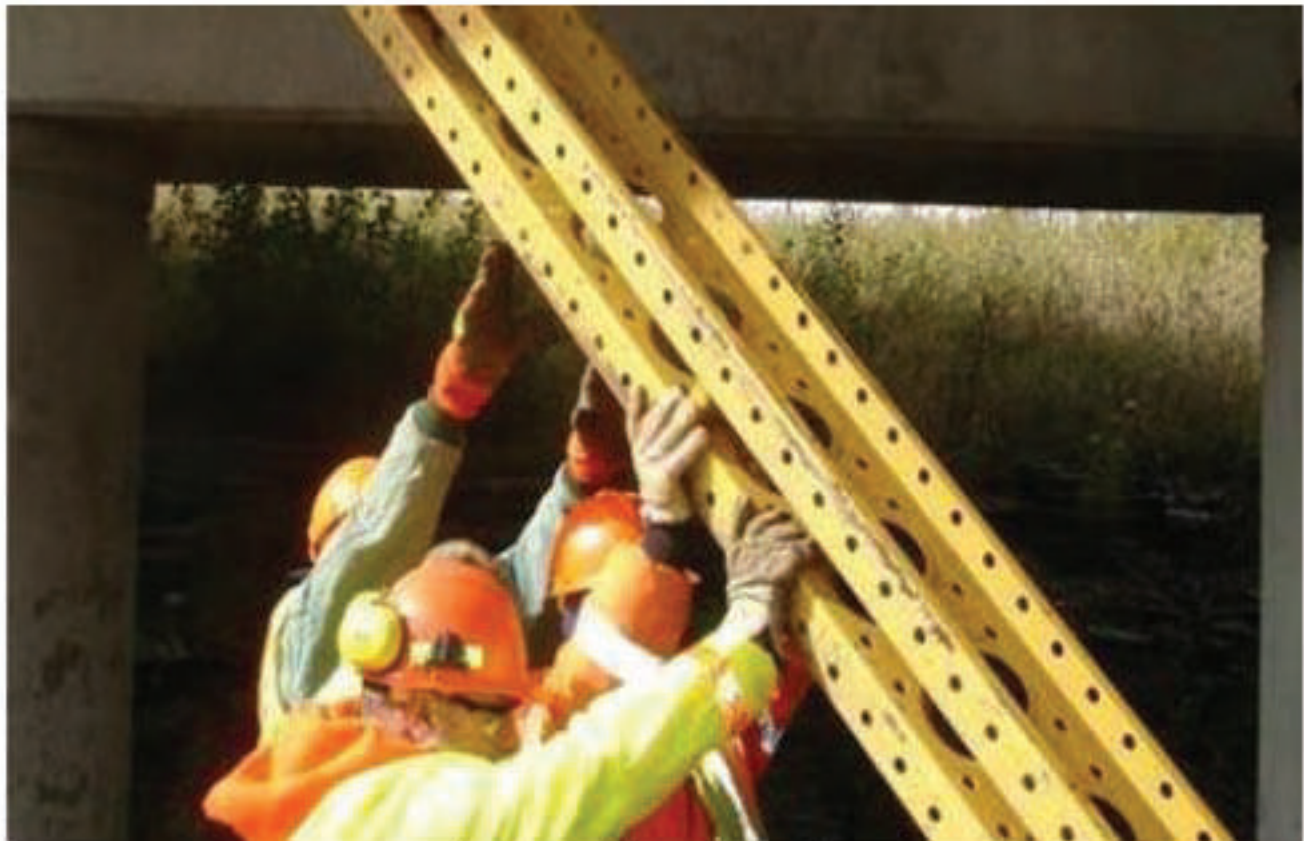
Figure 10.57: Lifting a Support Column
