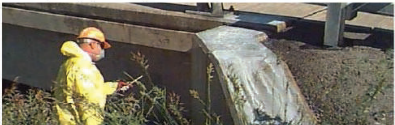
Figure 10.3: Hand Sealing the Sub-structure
