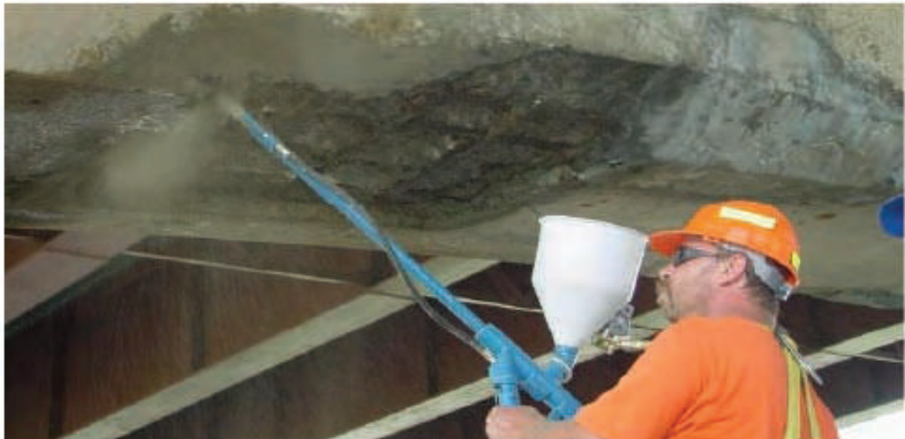
Figure 9.11: Shotcrete Application
