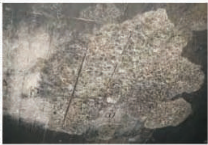
Figure A.8.3: Deteriorated concrete surface
