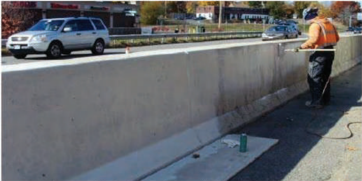
Figure 8.46: Application of Elastomeric Paint on Alkali-Silica Reactivity-Affected Barrier
