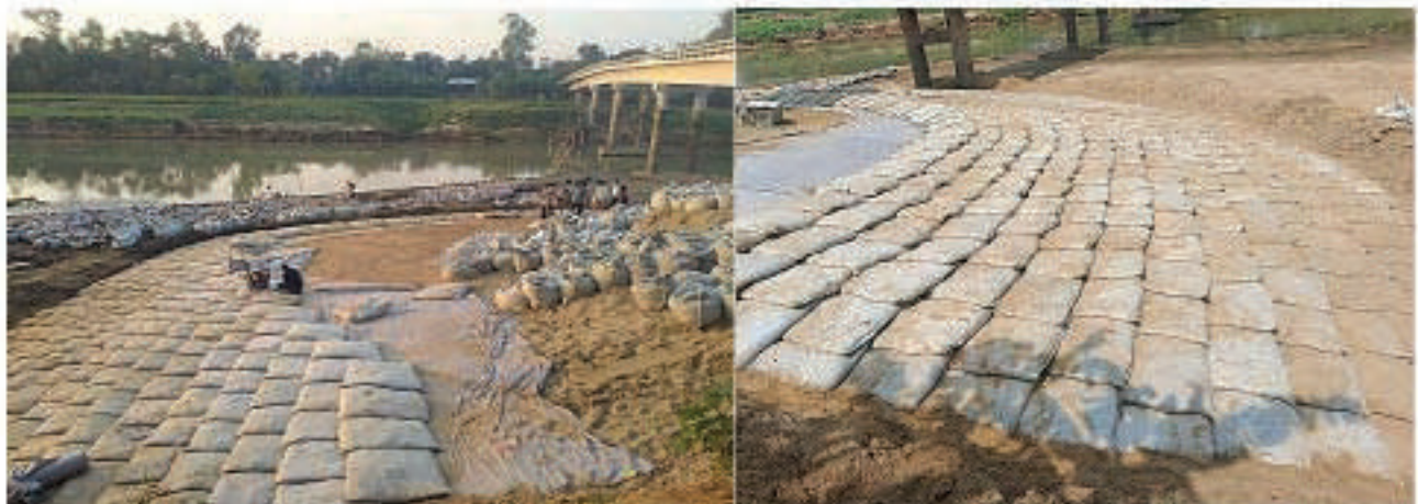
Figure A7.6: Repaired Scour near Abutment
