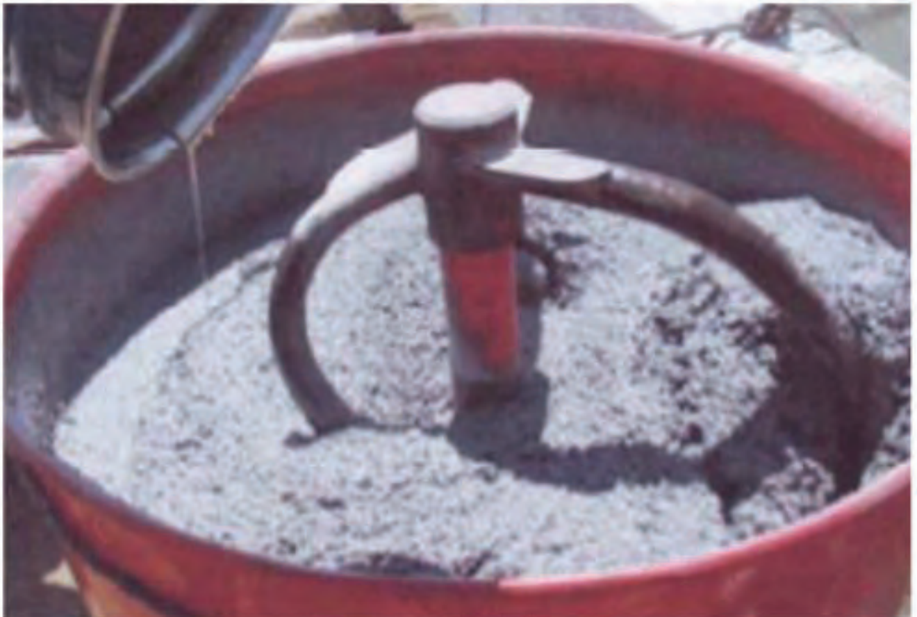
Figure 10.44: Application of polymer mortar
