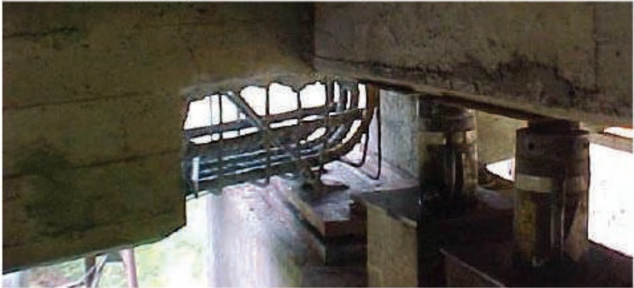
Figure 9.14: Beam End Repair Preparation
