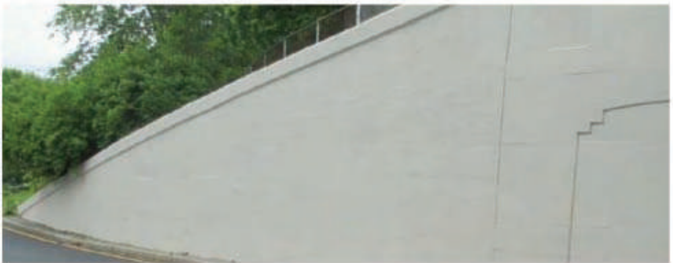
Figure 10.11: Retaining Wall After Repairs
