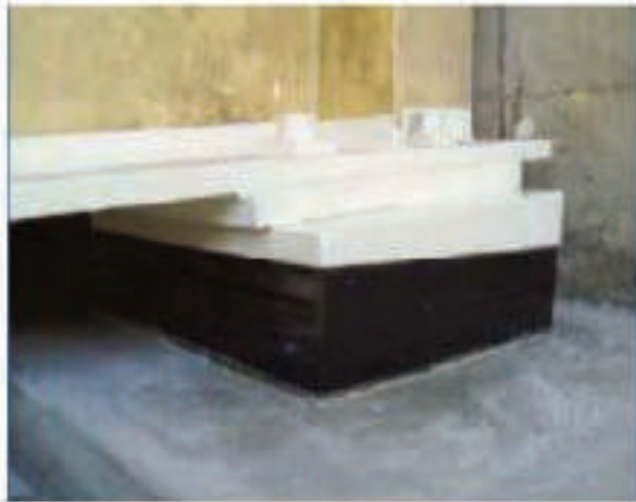
Figure 9.53: Bearing Shoe
