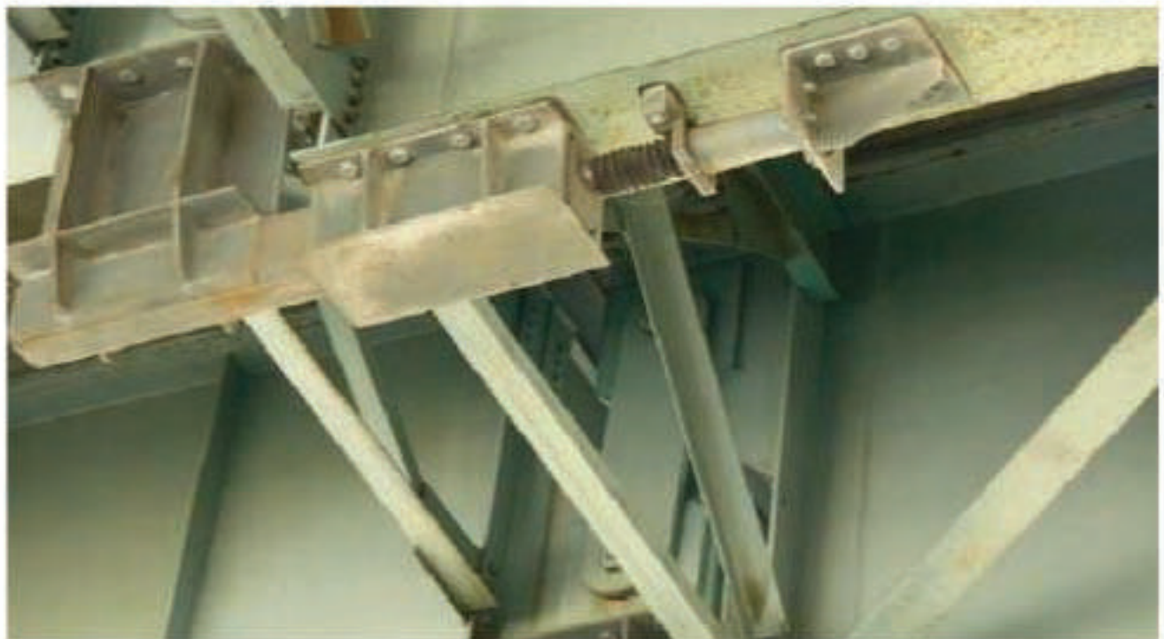
Figure 10.50: Viscous Dampers
