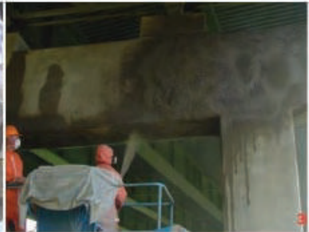
Figure 6.59: Shotcrete Repair of a Pier
