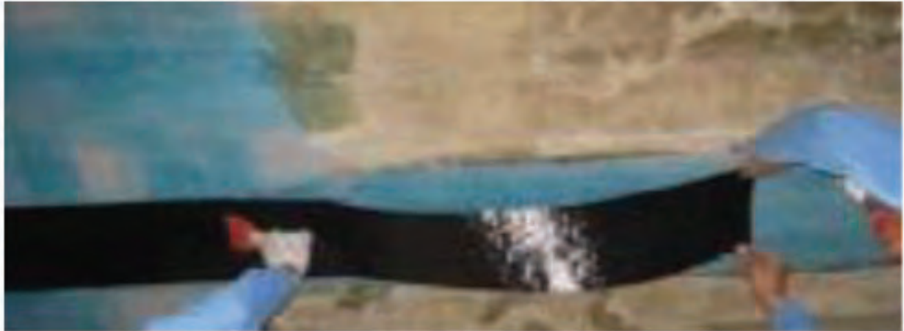
Figure 8.16: Putting Longitudinal Layer of CFS
