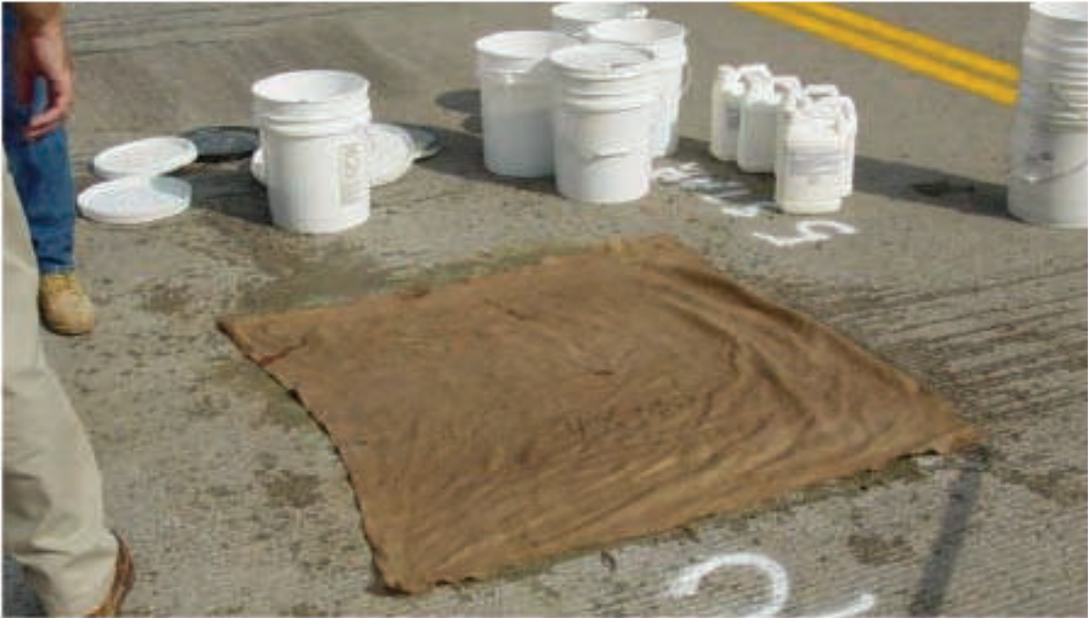
Figure 6.65: Wet Cure of a Small Deck Patch Using Pre-Soaked Burlap
