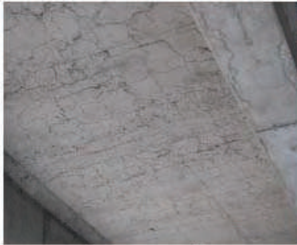
Figure 7.8: Map Cracking
