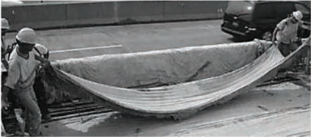
Figure 8.35: Curing the Concrete
