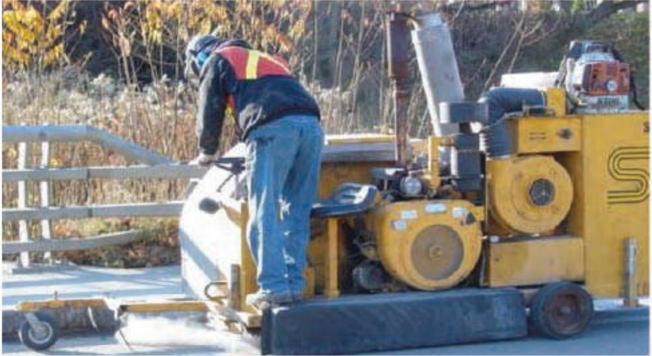
Figure 6.32: Shotblasting a Bridge Deck
