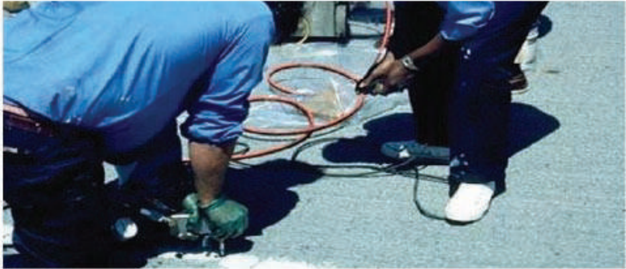
Figure 8.5: Epoxy Injection Repair
