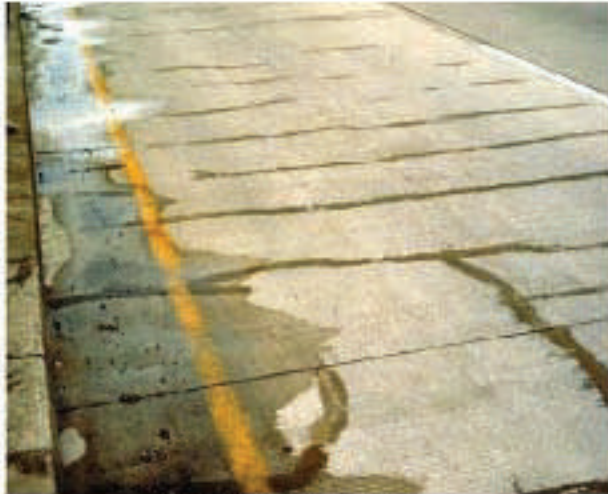
Figure 7.6: Plastic Shrinkage
