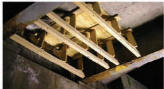
Figure 6.44: Forming for Deck Repair
