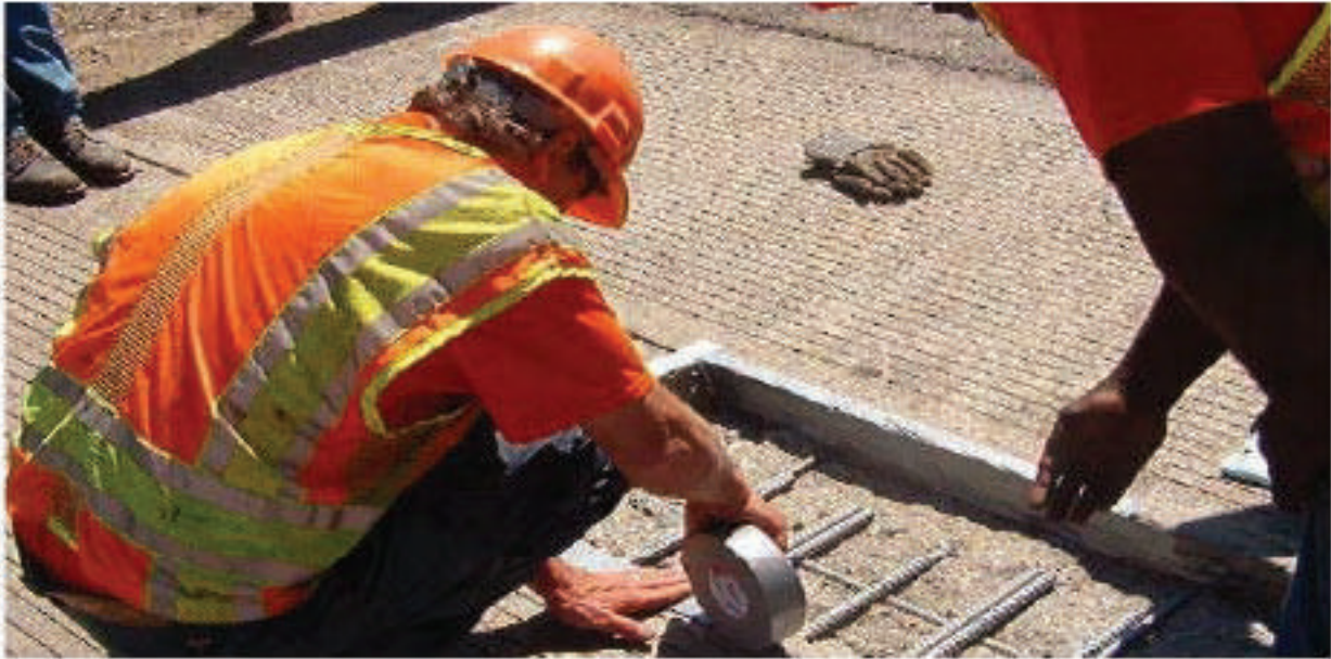
Figure 6.53: Taping the Perimeter for a Clean Look
