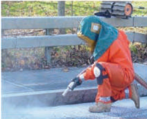
Figure 6.30: Abrasive Blast Cleaning Along the Curb Line
