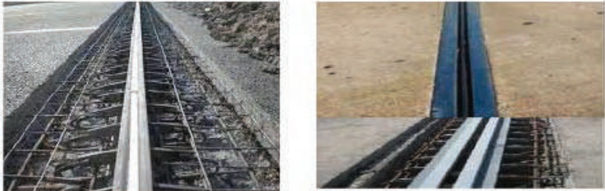
Figure 8.42: Expansion Joint Maintenance and Replacement
