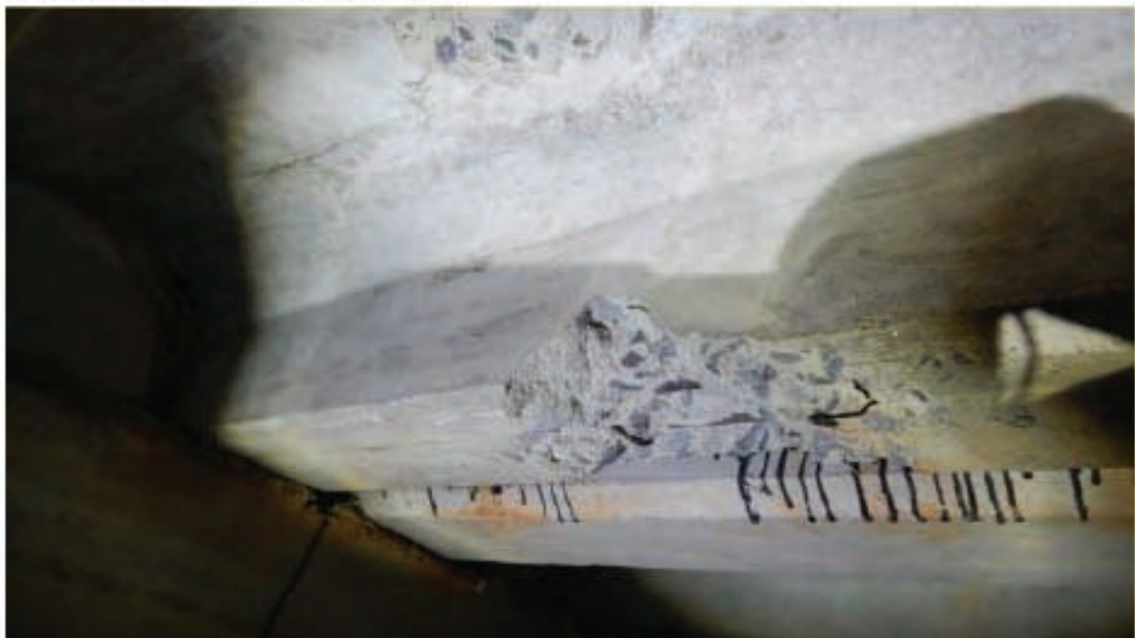
Figure 7.13: Spalling Concrete
