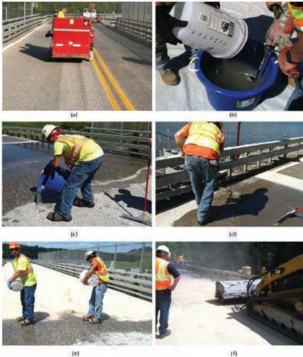
Figure 8.39: Common Steps in Epoxy Polymer Overlay
