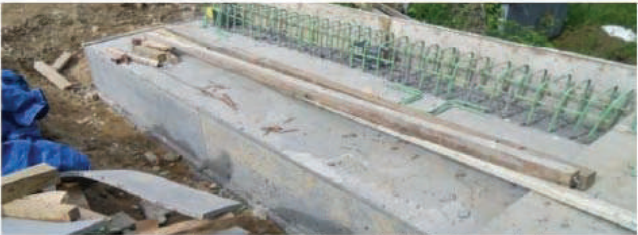
Figure 5.11: Reinforced Concrete Moment Slab (Under Construction)
