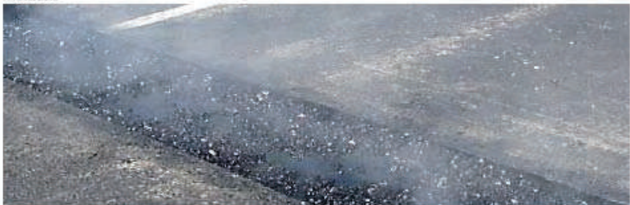
Figure 8.44: Plug Installation Showing Coated Aggregate and Binder
