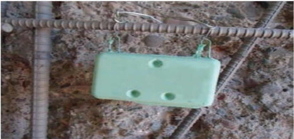
Figure 6.40: Sacrificial Anode Secured to Rebar
