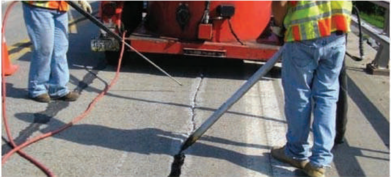
Figure 7.4: Placing Crack Sealing into "Working Cracks"
