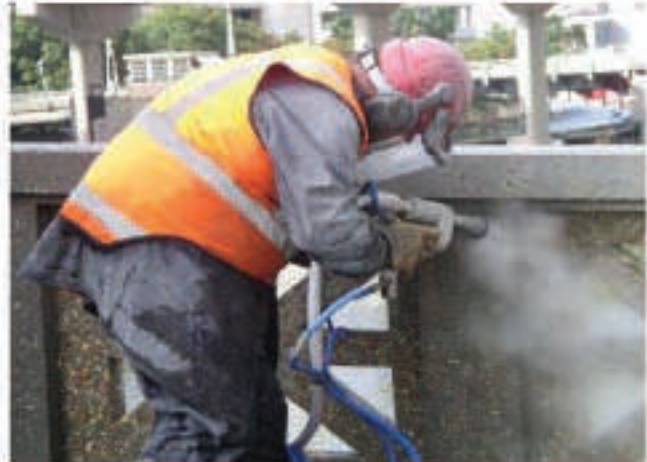
Figure 6.31: Abrasive Blast Cleaning a Concrete Barrier
