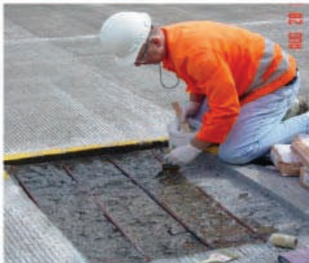
Figure 6.51: Priming a Patch with Polymer
