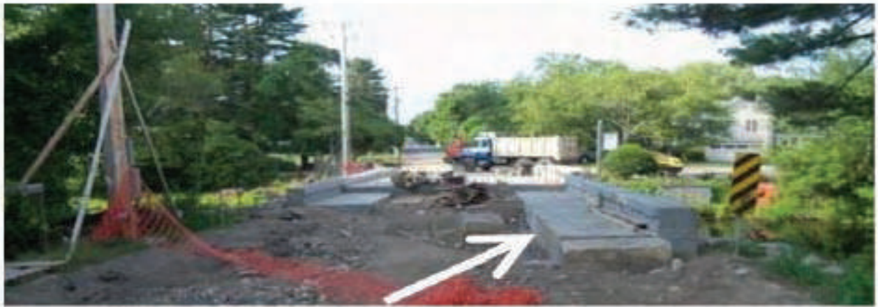
Figure 5.12: Moment Slab (indicated by arrow)
