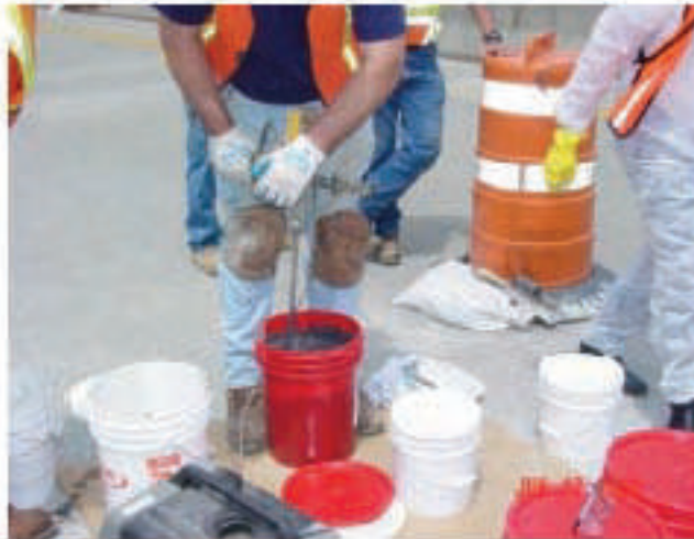
Figure 6.49: Five Gallon Bucket Mixing Method for Small Patches
