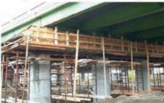
Figure 6.43: Forming for a Pier Cap Repair
