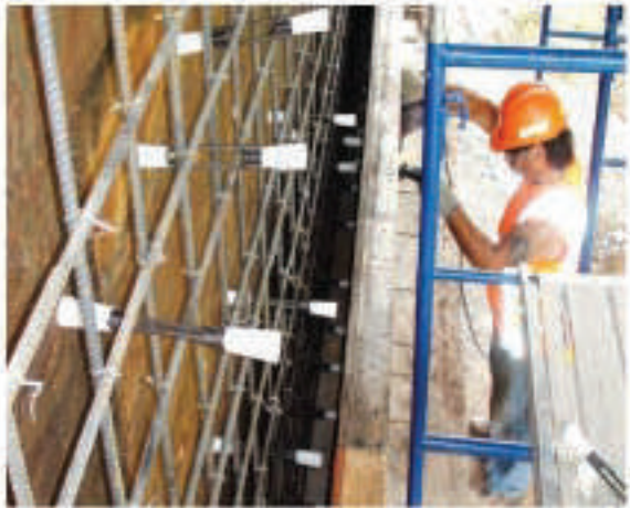
Figure 6.41: Forming for a Wingwall Repair
