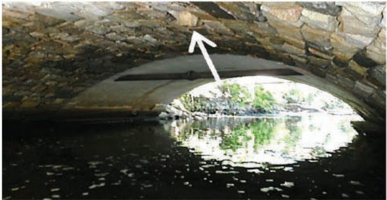
Figure 5.4: Single Slipped Stone
