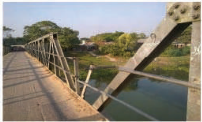
Figure 3.6: Accident damage of guardrails
