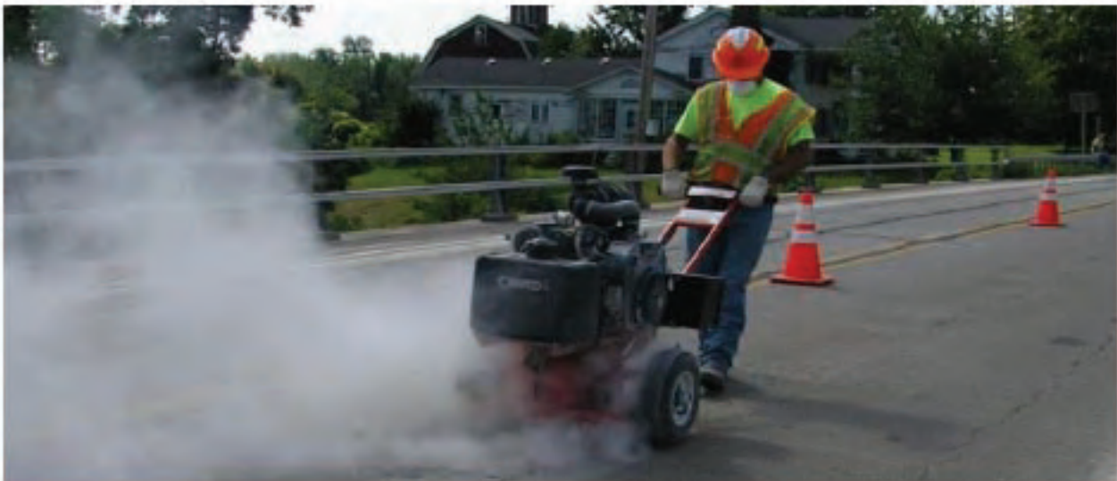
Figure 7.3: Routing Longitudinal Cracks
