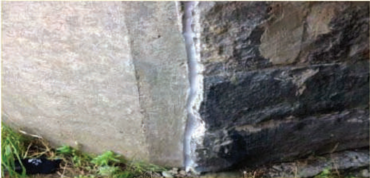
Figure 7.11: Active or live cracks sealed with an appropriate flexible sealant
