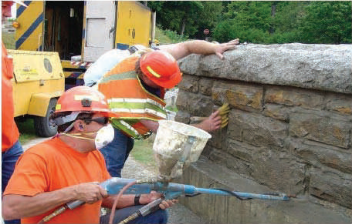
Figure 6.62: Re-Pointing a Laid-Up Stone Parapet with a Small Volume Shotcrete Tool
