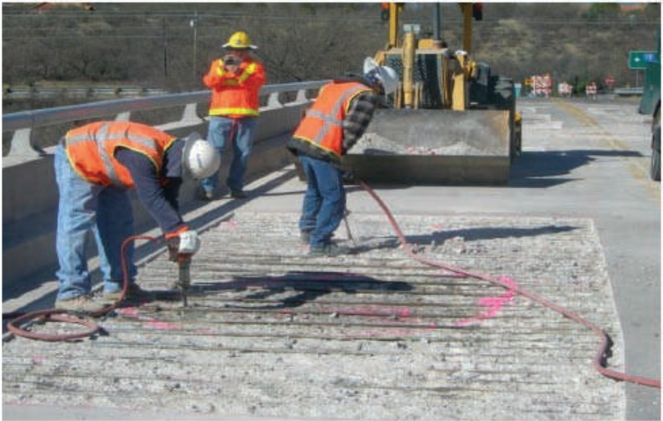
Figure 8.32: Removing the Delaminated Concrete
