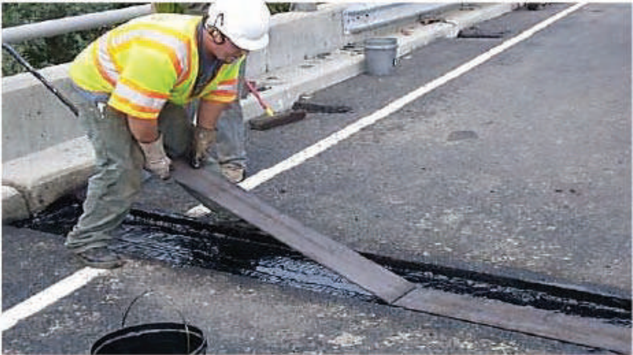
Figure 8.45: Bridging Plate Installation
