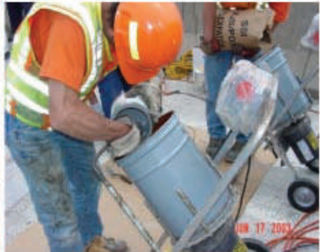
Figure 6.50: Power Mixers for Larger Patches
