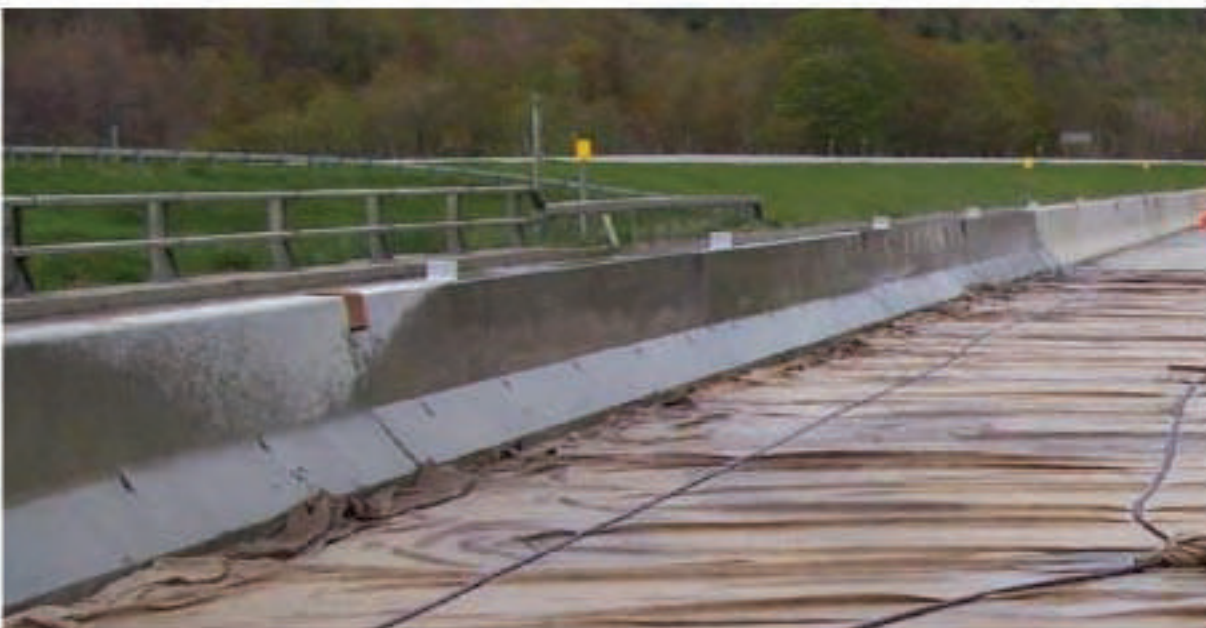
Figure 6.66: Wet Cure with Pre-Soaked Burlap for a Large Deck Repair
