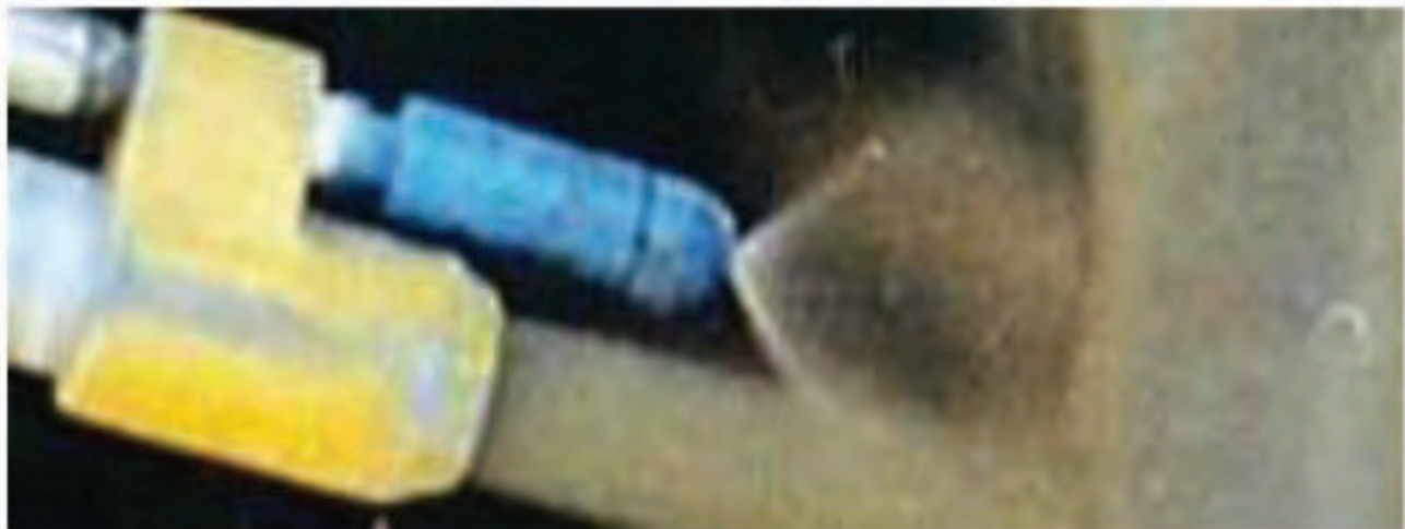
Figure 6.57: Mix Water Added at Nozzle
