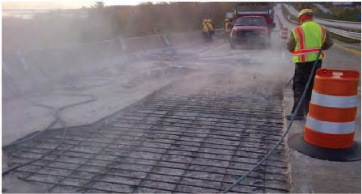
Figure 8.26: Cleaning with Compressed Air
