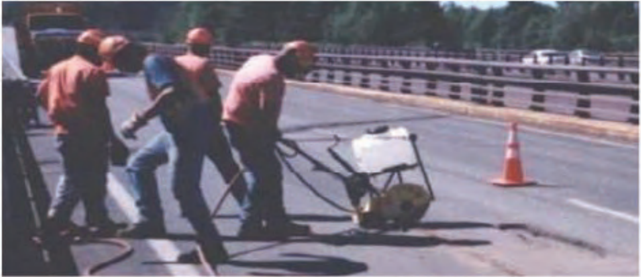
Figure 6.33: Saw cut and Removal of Deck Cover Concrete
