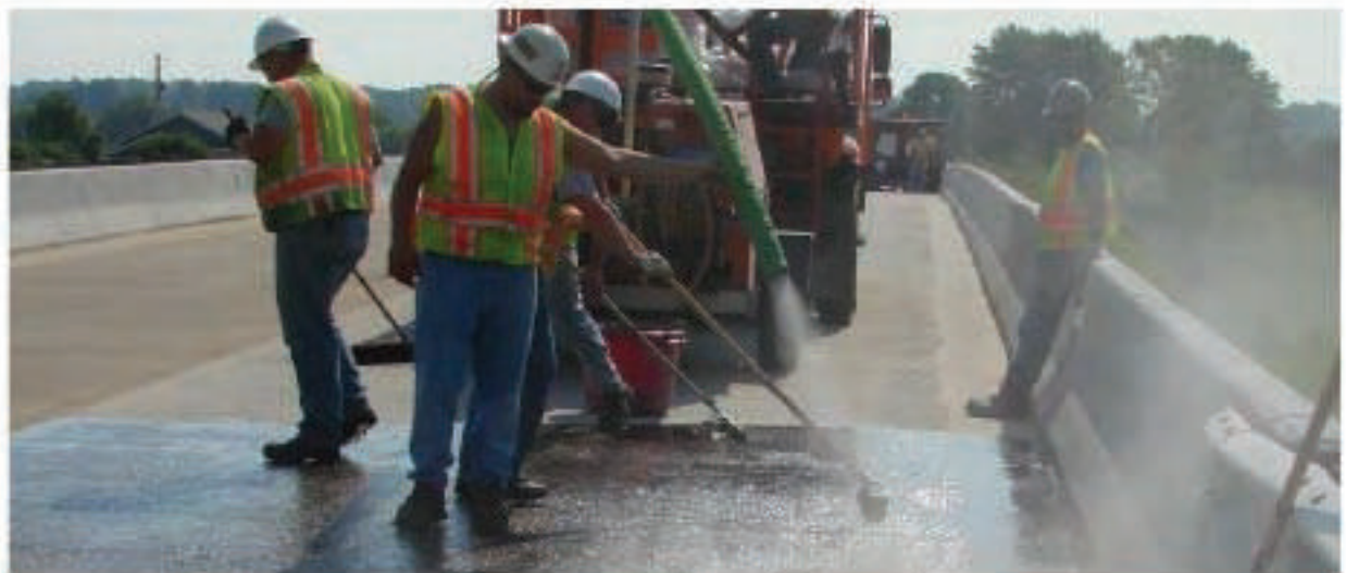
Figure 8.9: Broadcasting Sand (Aggregate)
