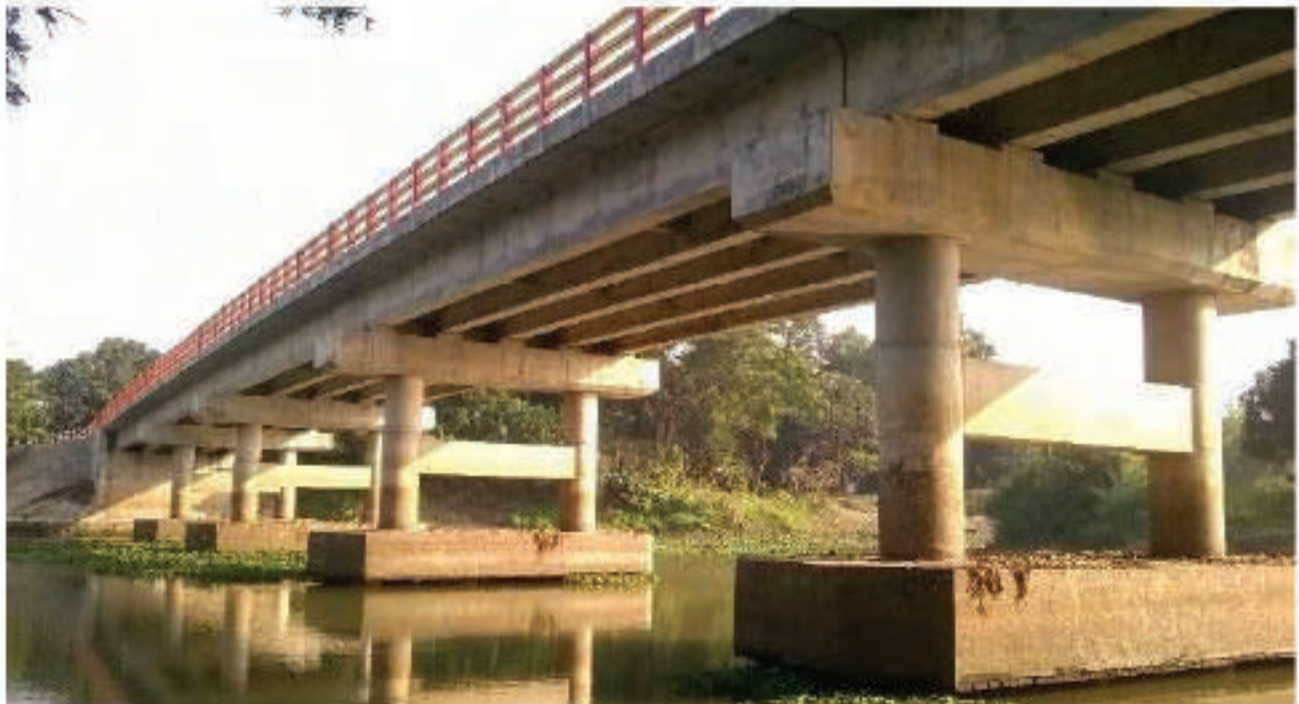
Figure 3.11: Vegetation removed from the adjacent area of the structure
