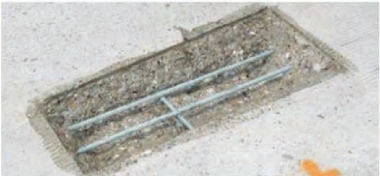
Figure 6.34: Saw cut Around Reinforcing Steel with Concrete Removed on an Angle
