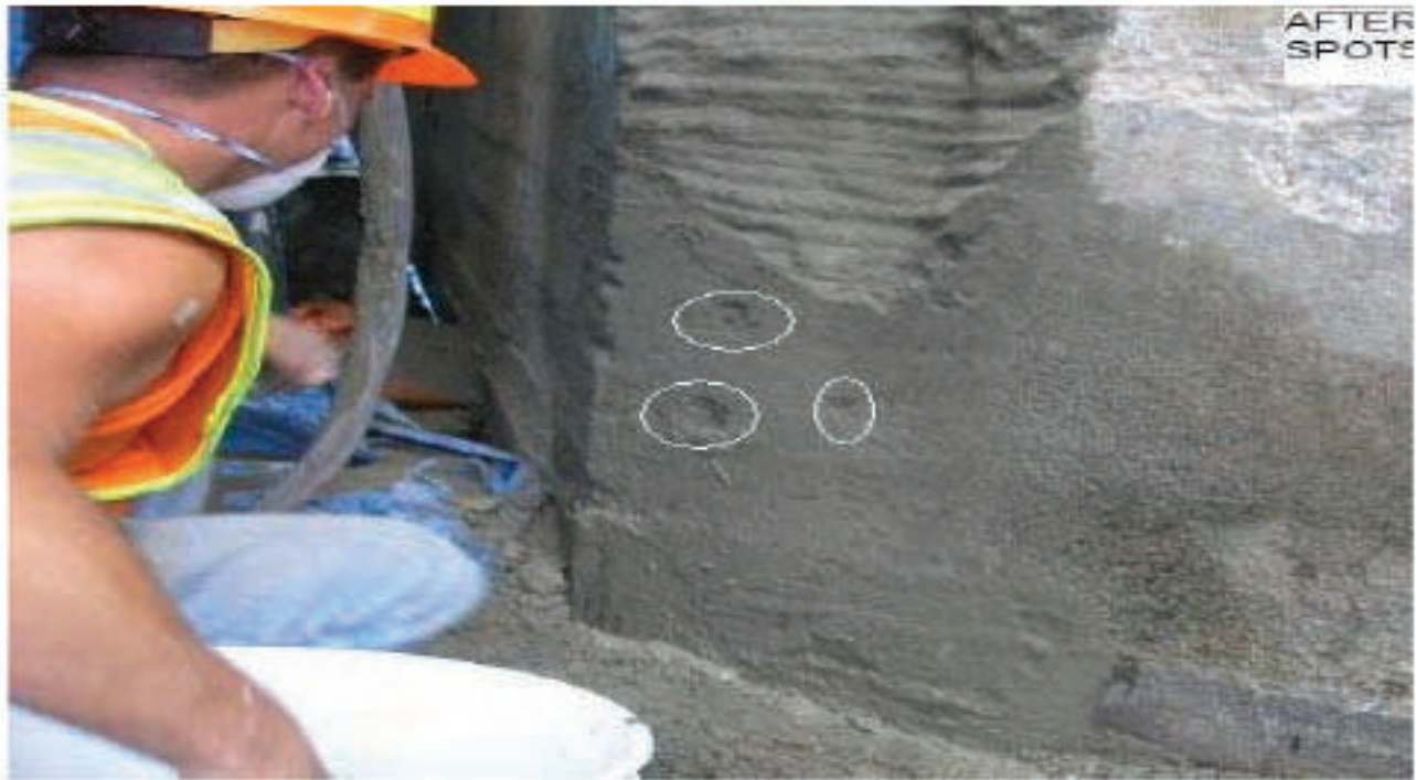
Figure 6.60: Repair "Bug-Holes" after Placing Shotcrete
