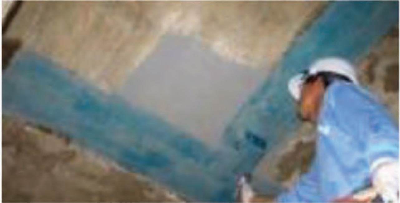
Figure 8.15: Application of Epoxy Resin for Undercoat
