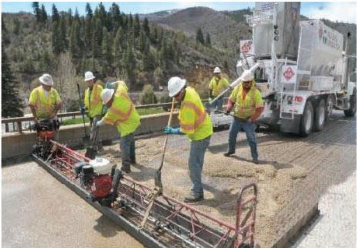
Figure 8.34: Placing the New Polyester Concrete
