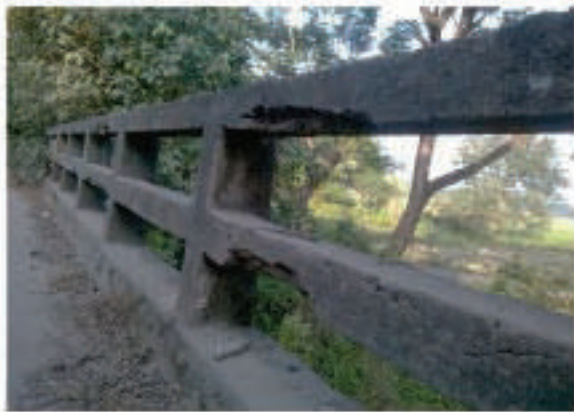
Figure 3.6: Accident damage of guardrails
