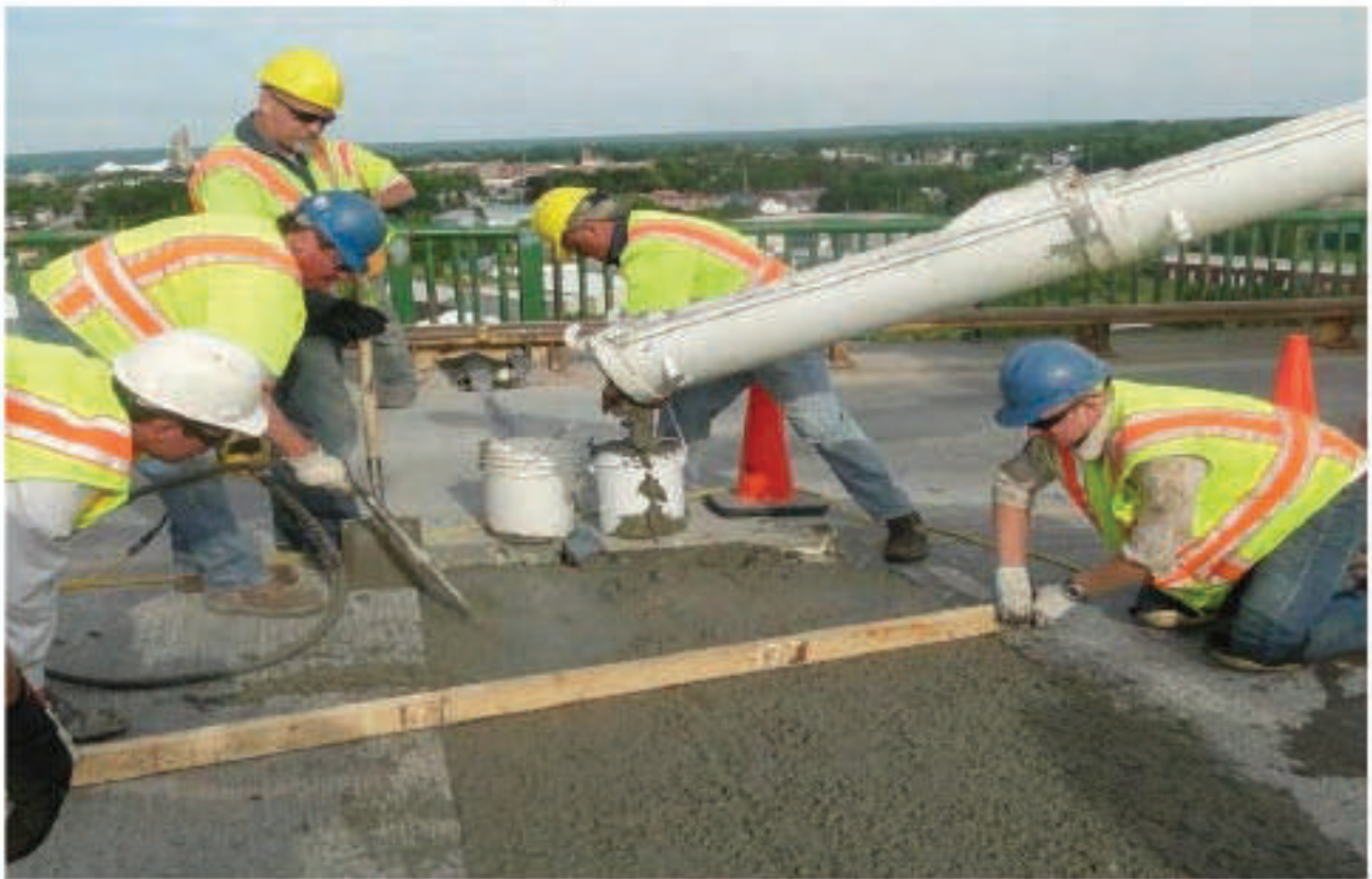
Figure 8.29: Vibration and Finishing
