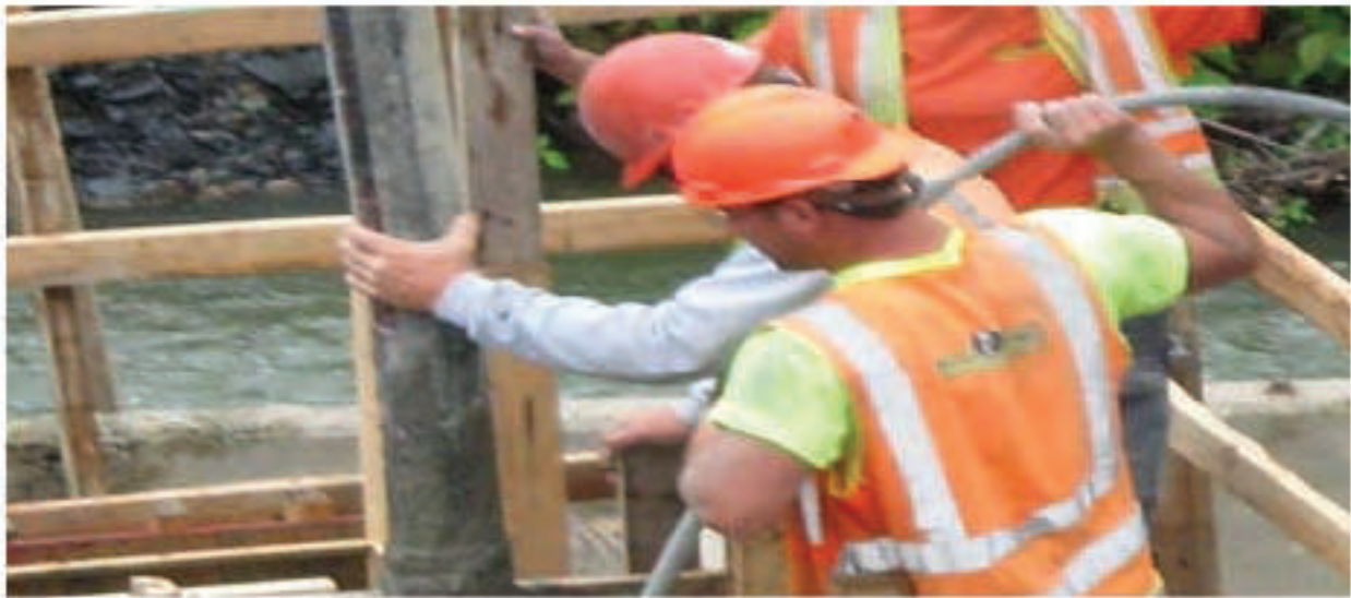
Figure 6.46: Pumping with Elephant Trunk and Consolidating with Vibrator
