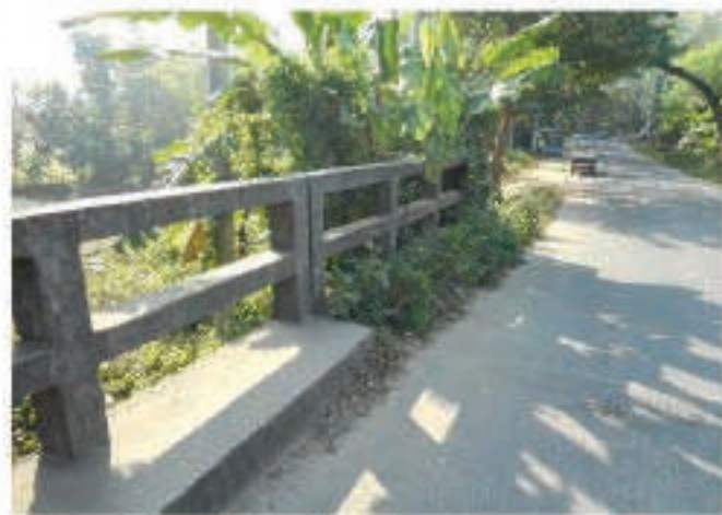
Figure 3.5: Growth of vegetation on the wearing surface
