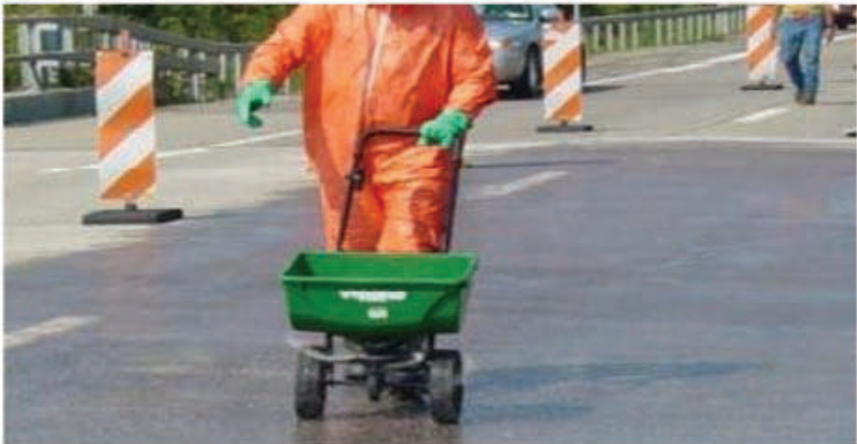
Figure 7.5: Spreading Mortar Sand onto Topical Crack Sealer
