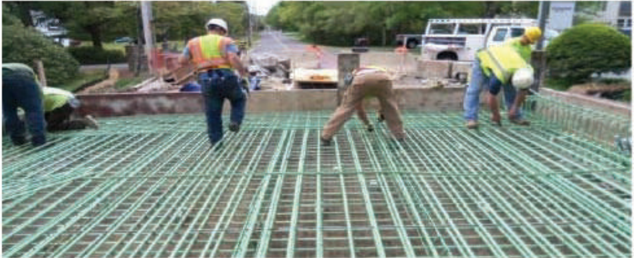
Figure 5.10: Reinforced Concrete Relieving Slab (Under Construction)
