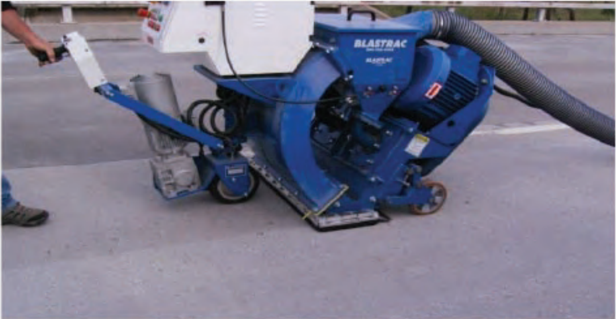
Figure 8.37: Preparing the Deck with Shot Blasting.
