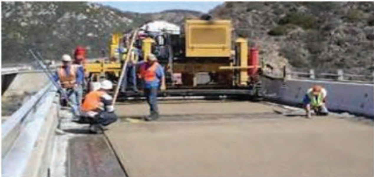
Figure 8.38: Placing the Concrete Overlay
