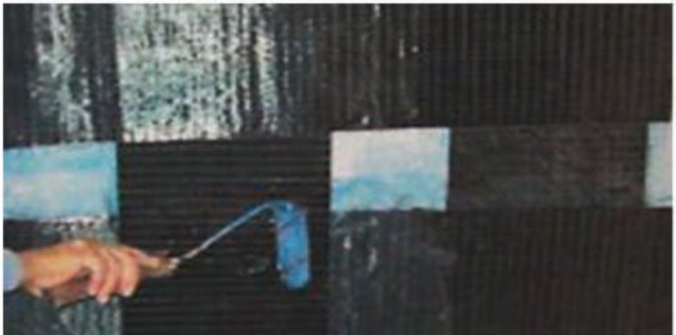
Figure 8.19: Squeezing of Strip to Entrapped Air
