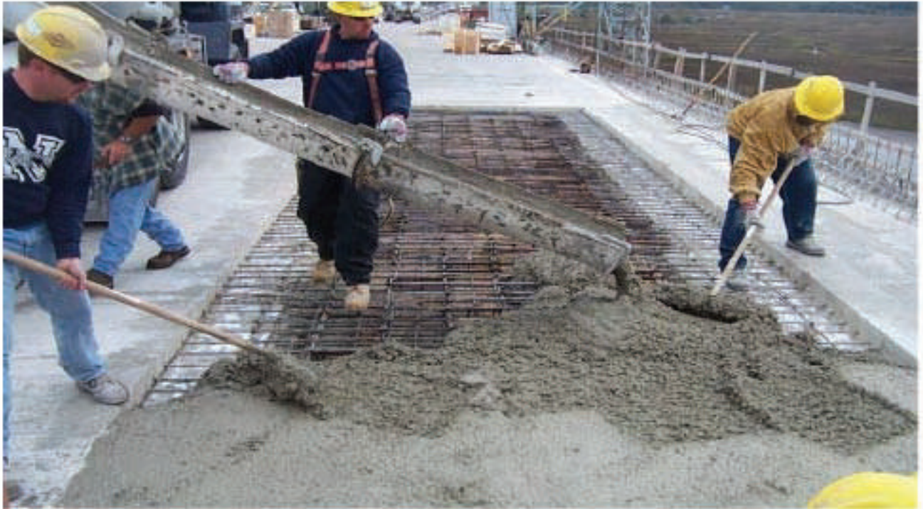
Figure 8.28: Concrete Placement
