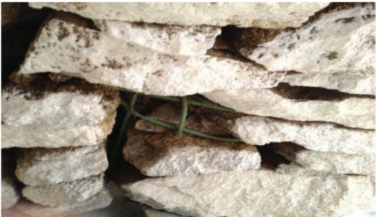
Figure 4.11: Reinforcing Steel Installed Prior to Grouting Stone Masonry
