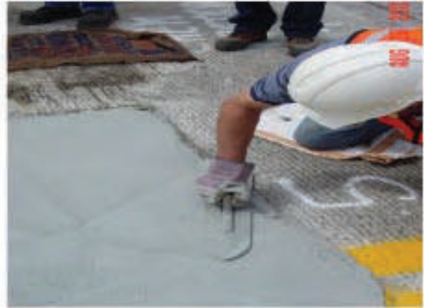
Figure 6.64: Trowel Finish on a Deck Patch
