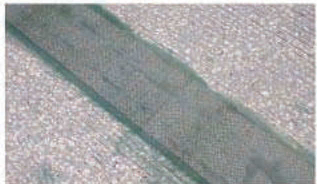
Figure 8.6: Surface Epoxy Sealing with Optional Fabric
