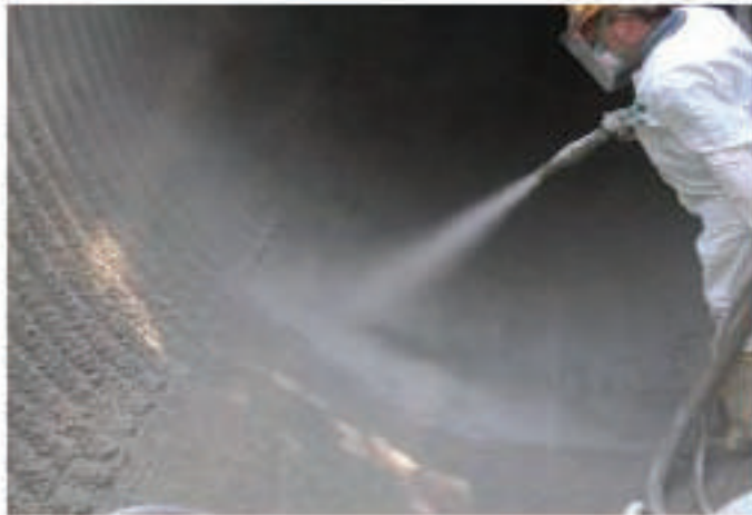
Figure 6.58: Shotcrete Repair of an Invert of a Corrugated Metal Culvert
