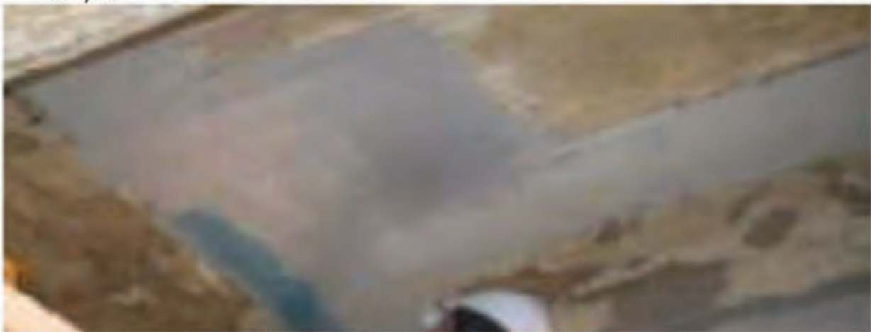
Figure 8.14: Adjustment of Unevenness with Putty
