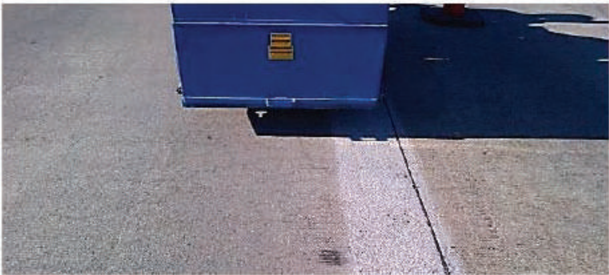
Figure 8.7: Shot Abrading Deck Preparation
