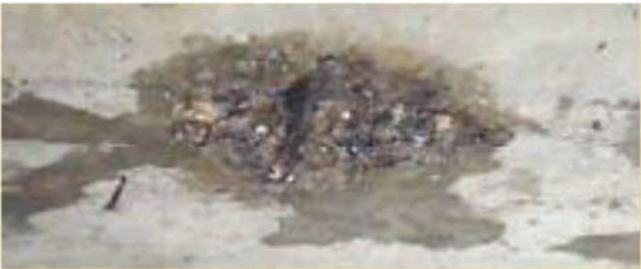
Figure 6.38: Epoxy bonding coat
