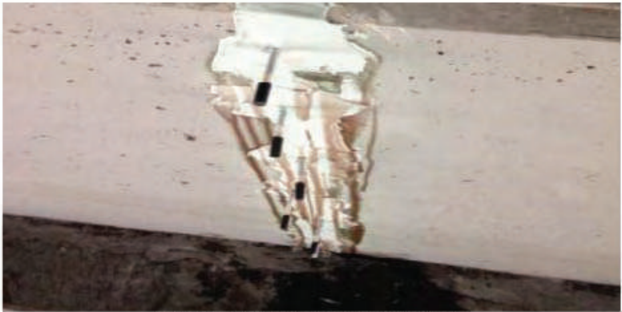
Figure 7.9: Injected cracks with epoxy resin through ports
