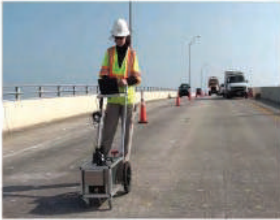
Figure 6.22: USW on Bridge Deck
