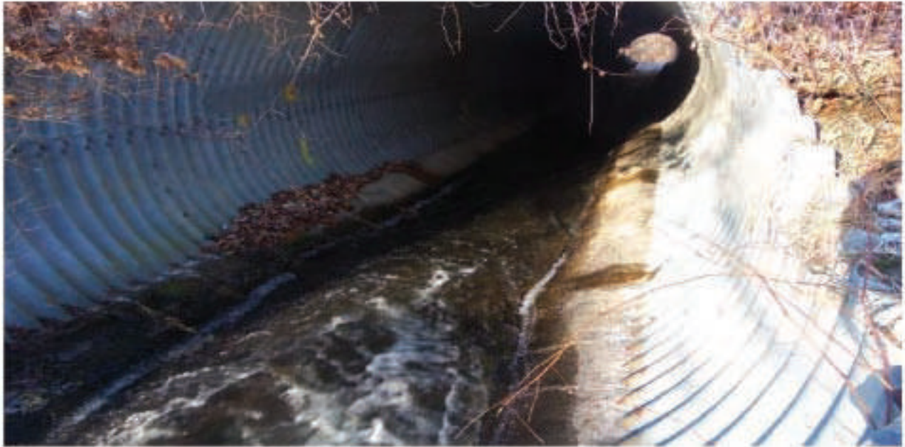
Figure 4.8: Concrete Paved Invert
