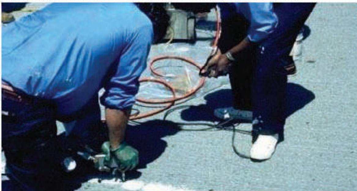
Figure 7.6: Epoxy Injection Repair (Horizontal Surface)
