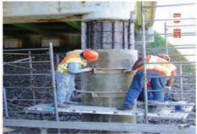
Figure 6.42: Manufactured Forms for Columns
