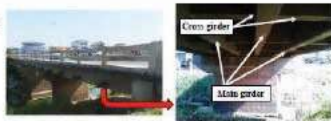
Photo 1.31 Girder Components
