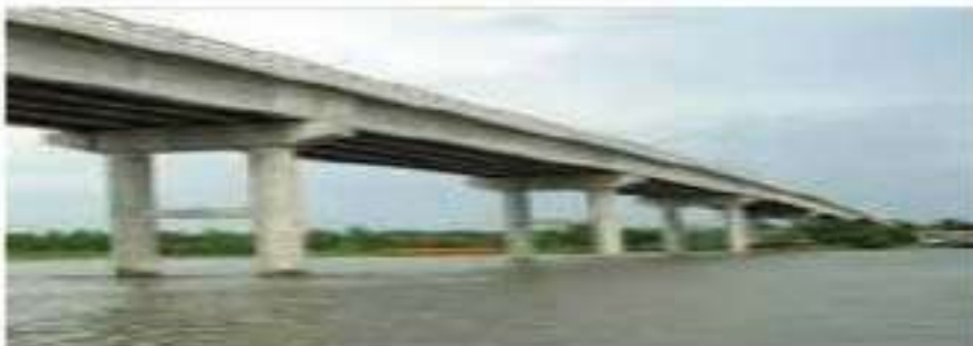
Fig: 1-4-4 RCC Girder Bridge
