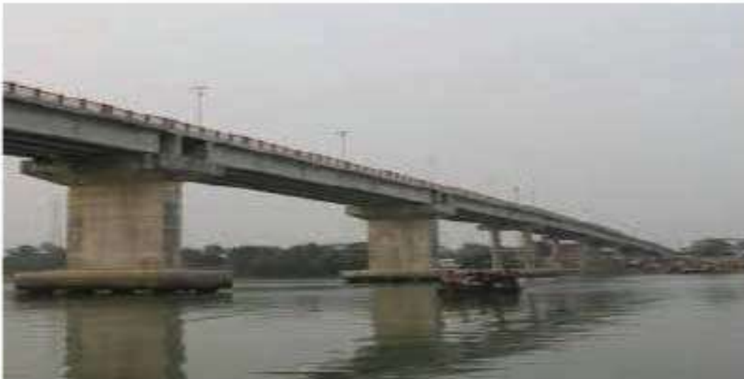
Fig: 1-4-5 PC Girder Bridge
