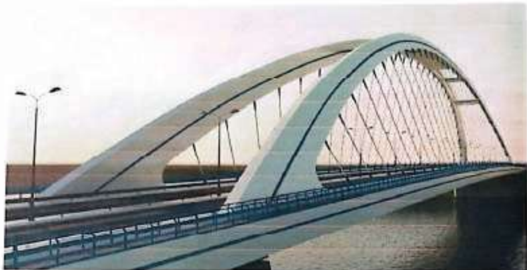
Photo: Arch Rib of Variable Depth (Tapered Rib)
