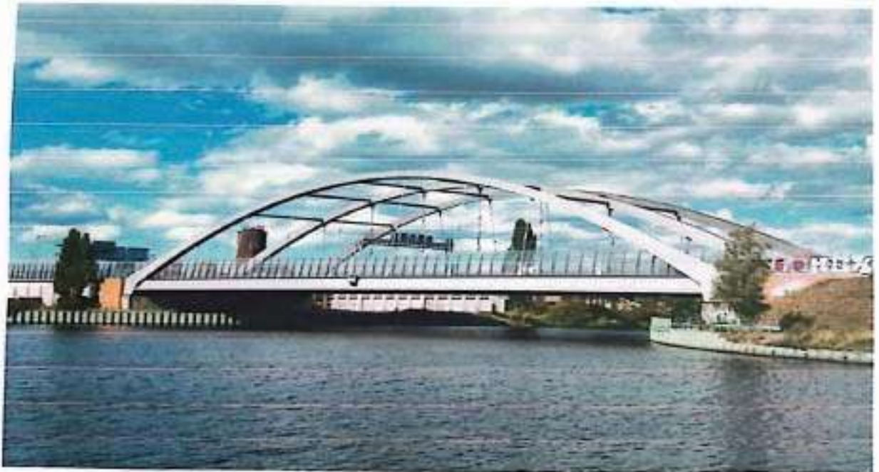
Photo: Tied Arch Bridge
