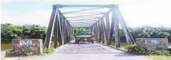
Fig: 1-4-9 Bailey with Steel Deck Bridge
