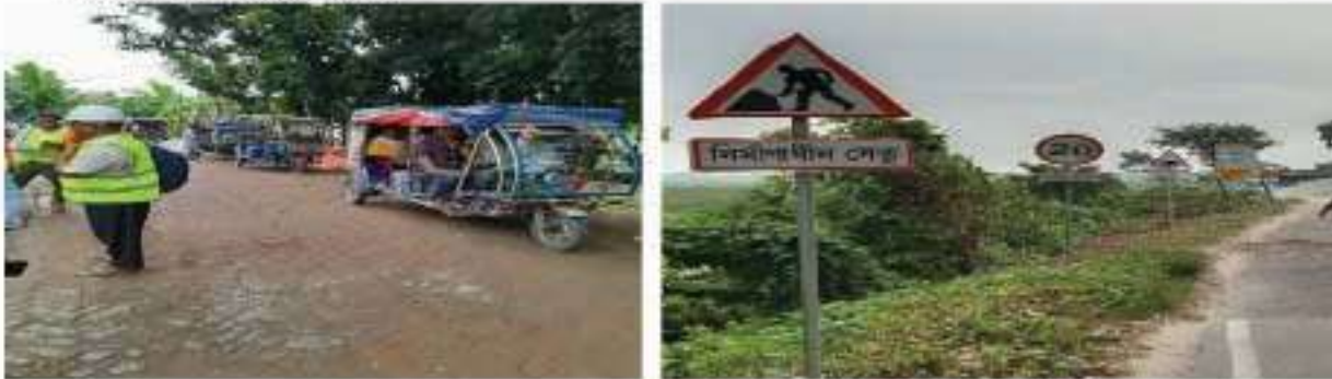
Figure: Road Diversion
