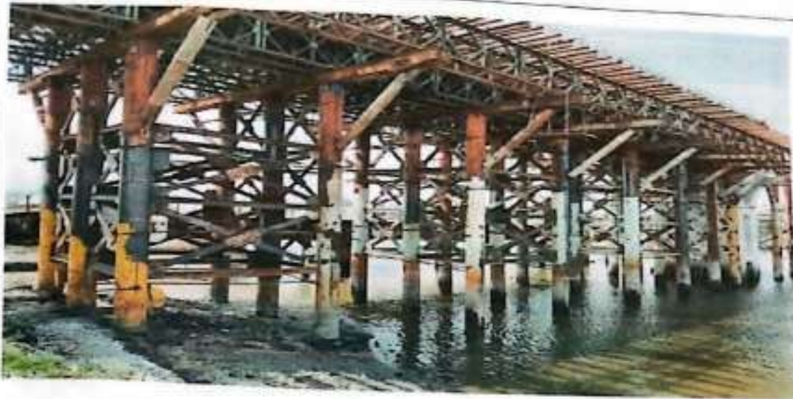
Standard Scaffolding for Bridge Works
