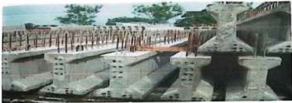
Pre-tensioning of Girders
