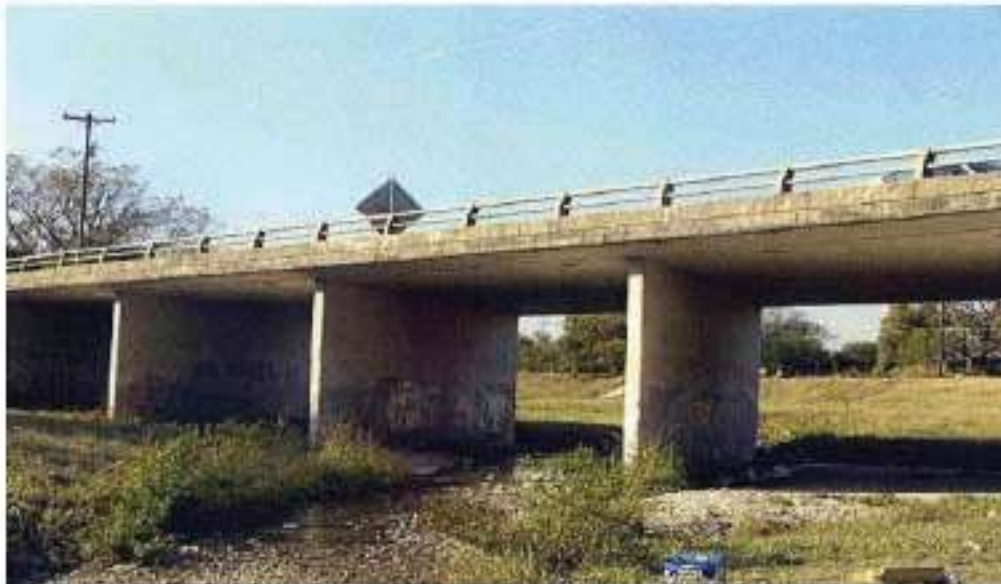
Fig: 1-4-7 Slab Bridge
