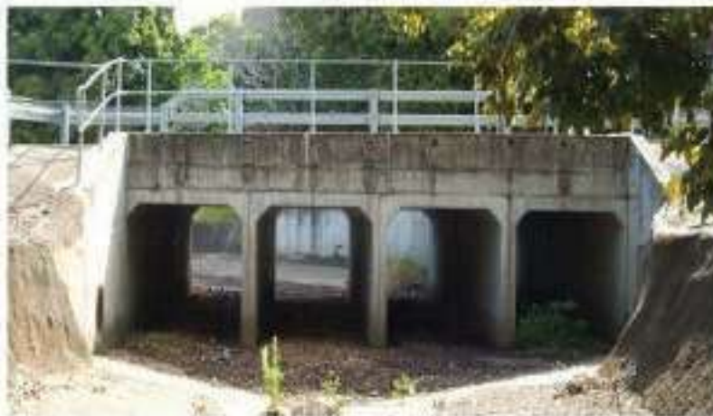
Fig: 1-4-2 Typical Box culvert
