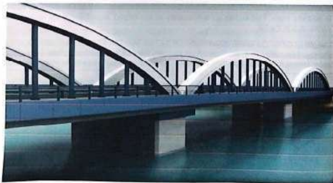
Photo: Arch Rib of Constant Depth (Tapered Rib)
