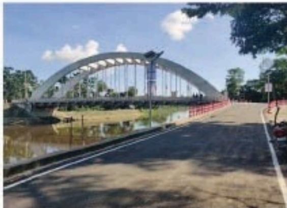
Fig 5.52.: 50.00m long RCC arch Girder Bridge
