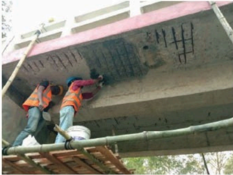
Fig 5.27.: Repairing of Deck Soffit (Side)
