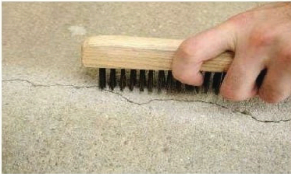
Fig. 5.22. Surface Cleaning before application
