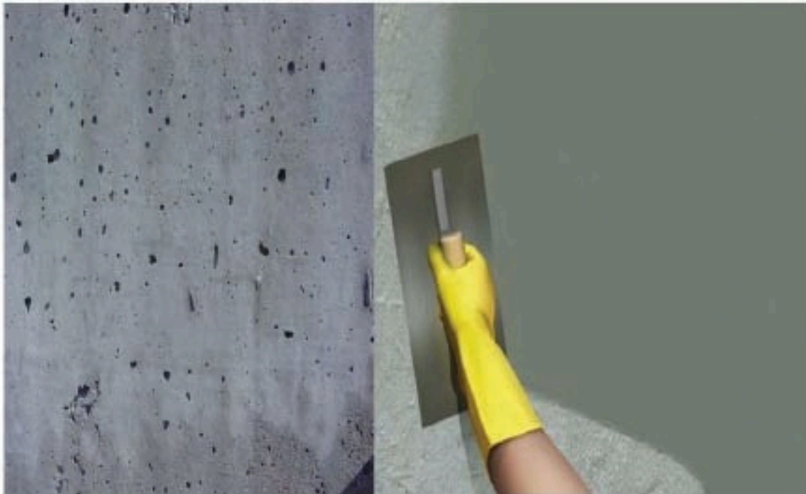
Figure 5.11.: Skim Coat Application before and after Condition
