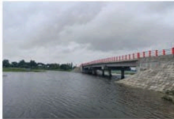
Fig 5.53.: 60.05m long RCC Girder Bridge new construction on existing gap
