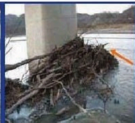
Fig.5.8. Pier with flow obstruction
