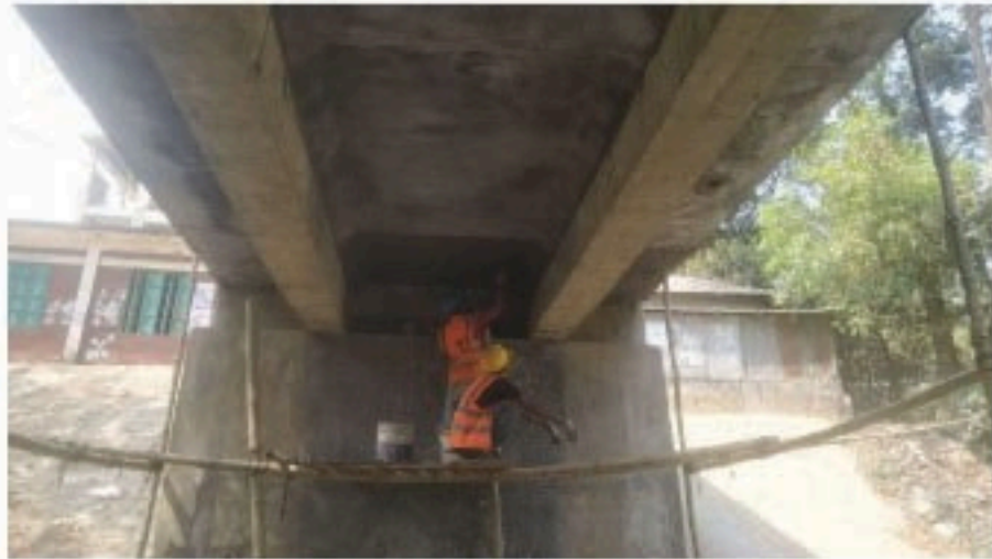
Fig 5.28.: Repairing of Deck Soffit (Middle)
