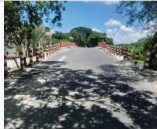
Fig 5.57.: Completed Major Maintenance under SupRB Project.
