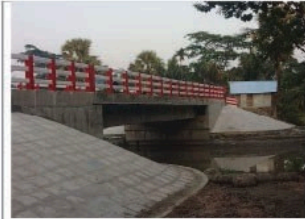
Fig 5.56.: Completed RCC Girder Bridge under SupRB Project.
