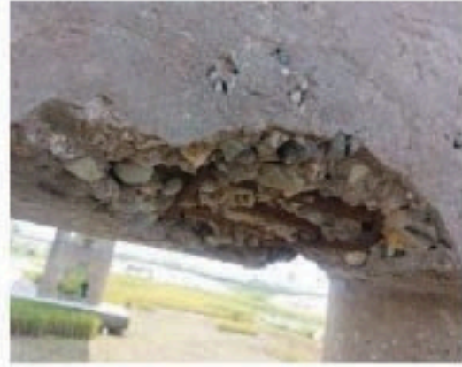
Fig 5.24.3: Girder bottom rebar
