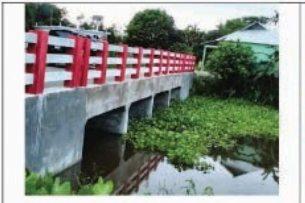
Fig 5.58.: Major Maintenance of Culvert under SupRB.
