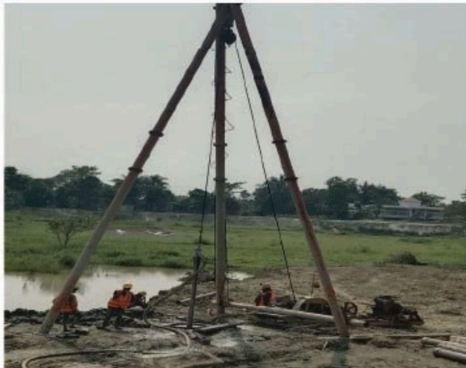
Fig 4.8 Ongoing Piling work on Bridge Replacement Category Under SupRB
