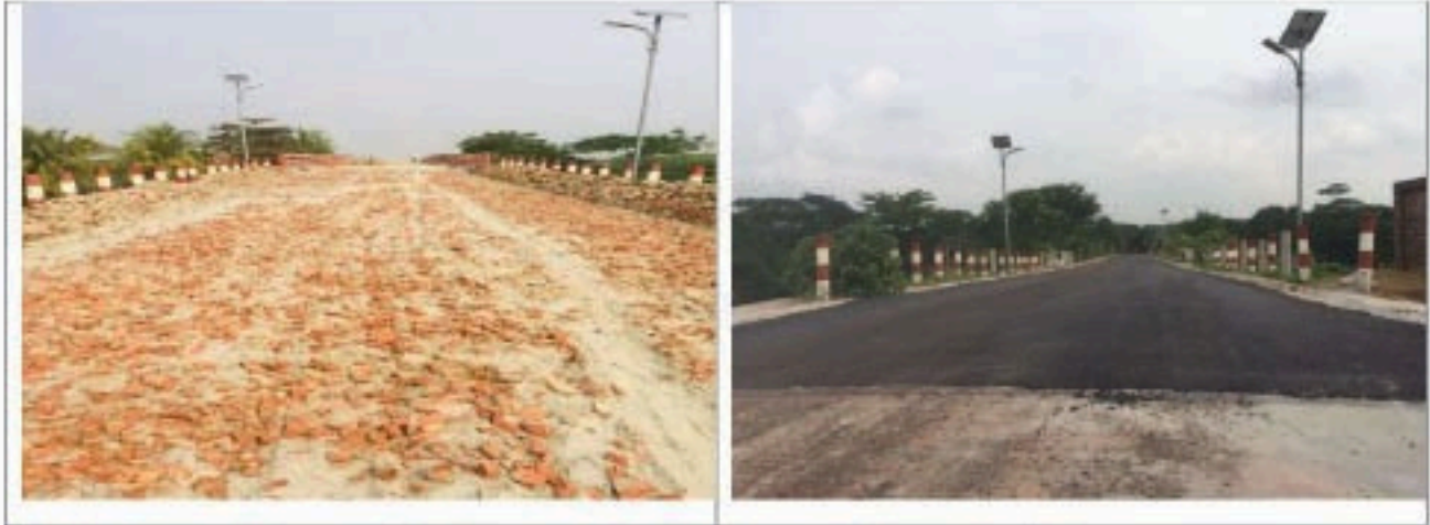
Fig 5.48.: Ongoing approach road and Completed Road work
