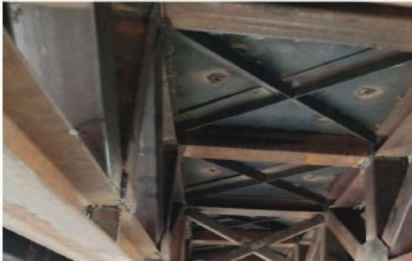
Fig 5.43.: Retrofitting Steel truss place on a pier cap with bearing
