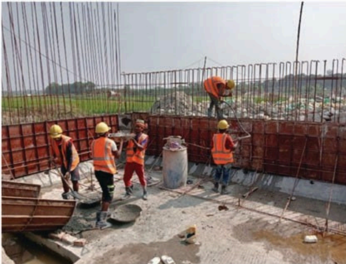
Fig 4.9 Ongoing Bridge Abutment Casting work
