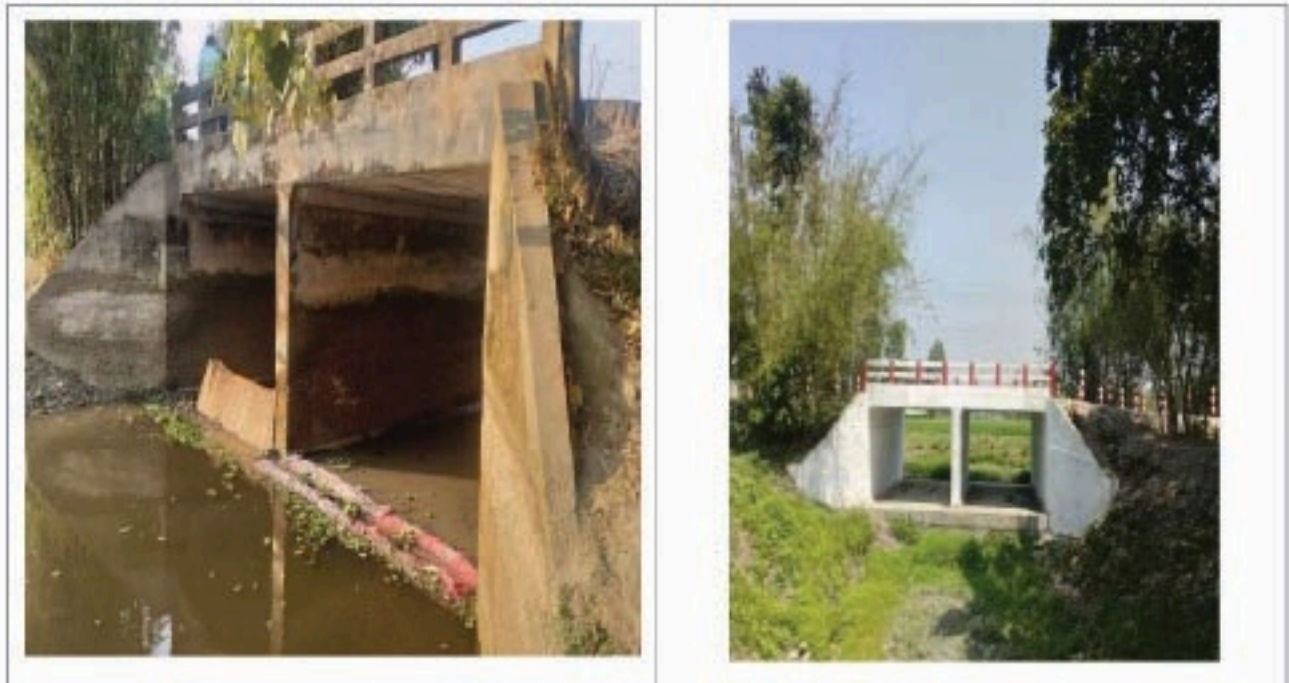
Fig 5.43. : Before and after Minor Maintenance of 2 vent RCC box Culvert
