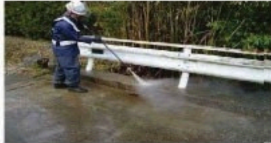
Fig. 5.2. Removing of soil and weed by jet water
