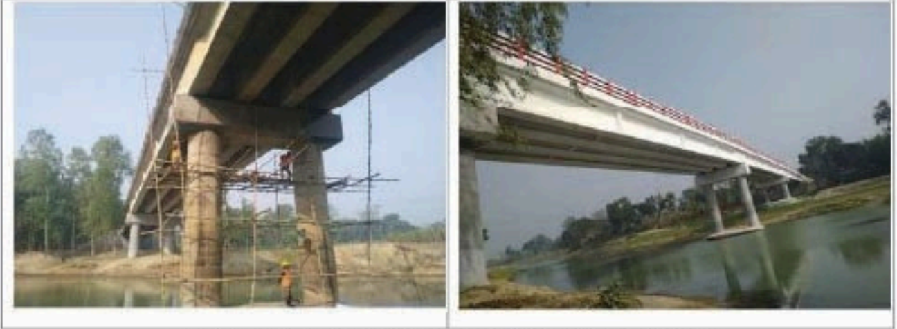
Fig 5.47.: Before and after Minor Maintenance PSC Girder Bridge
