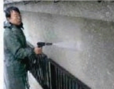
Fig.5.6 Cleaning concrete surface by jet water
