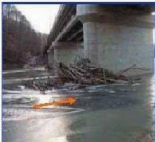
Fig.5.7. Pier with flow obstruction
