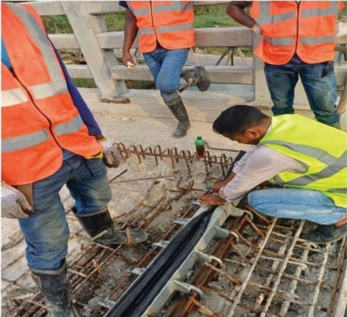
Fig 4.16 Installation of strip seal expansion joint
