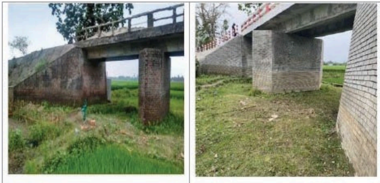
Fig 5.44.: Before and after minor maintenance of Brick Culvert
