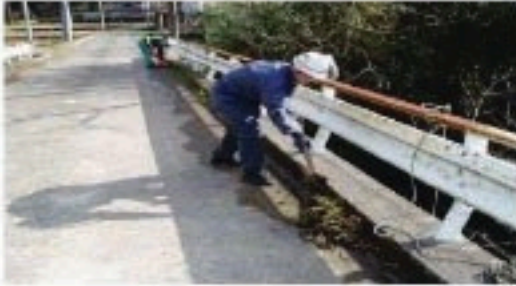
Fig. 5.1. Removing of soil and weed by shovel.
