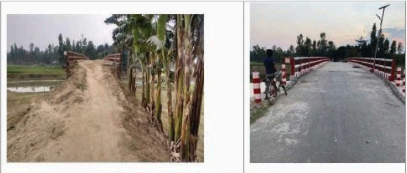
Fig 5.49.: Road work before and after Completion
