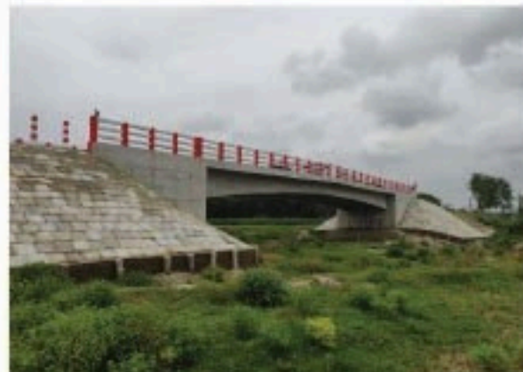
Fig 5.55.: Completed Bridge Arch Girder Bridge under SupRB Project.
