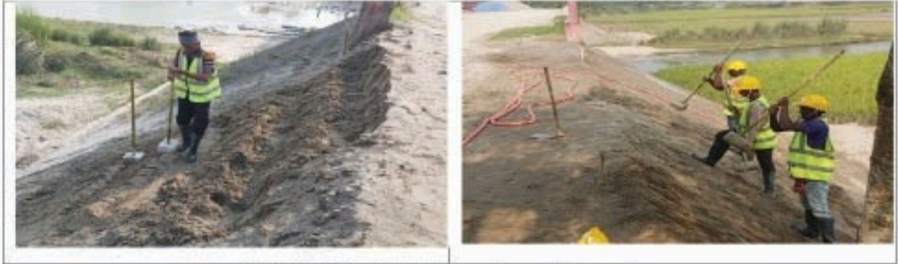
Fig 5.51: Embankment Slope Compaction work
