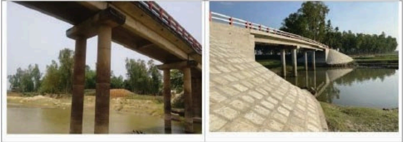
Fig 5.45. : Before and after Minor Maintenance work of 3 Span RCC Girder Bridge
