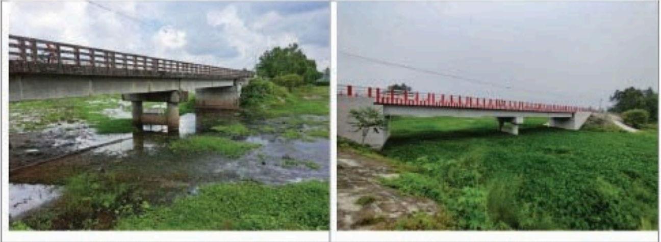
Fig 5.46.: Before and after minor maintenance of 2 span RCC Girder Bridge.
