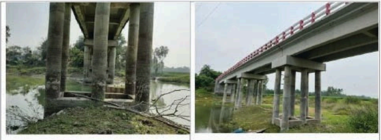
Fig 5.50.: Before and after Major Maintenance PSC Girder Bridge
