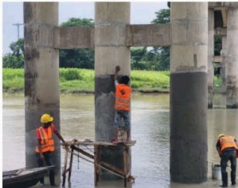
Fig 5.32.: Pier Repair by Polymer Mortar
