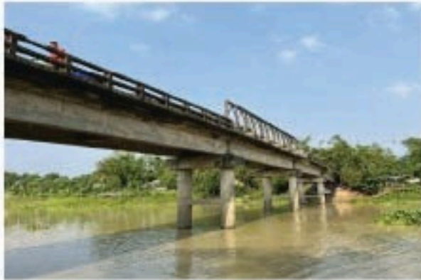
Figure 1: Existing Condition of Gopalpur Bridge
