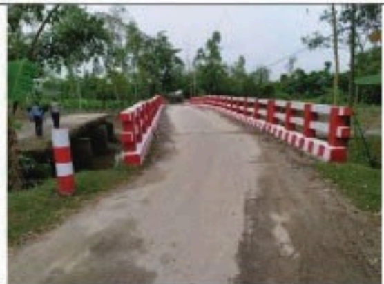
Fig 5.59.: Completed RCC Girder Bridge under Replacement Category of SupRB Project
