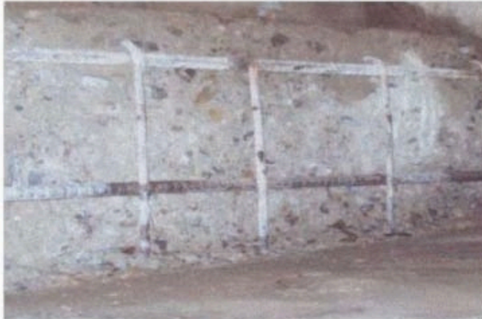
Fig 5.38.: Bonding coat application
