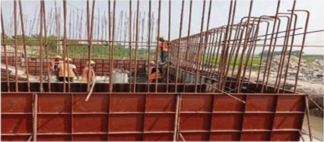
Fig 4.10 Ideal Shuttering
