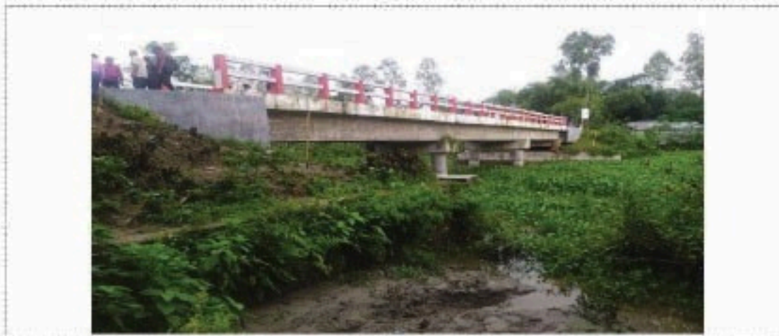
Fig 5.60.: Minor Maintenance of Bridge under SupRB Project
