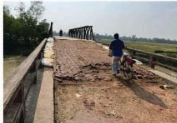
Figure 2: Baily Panel in Mid-Span
