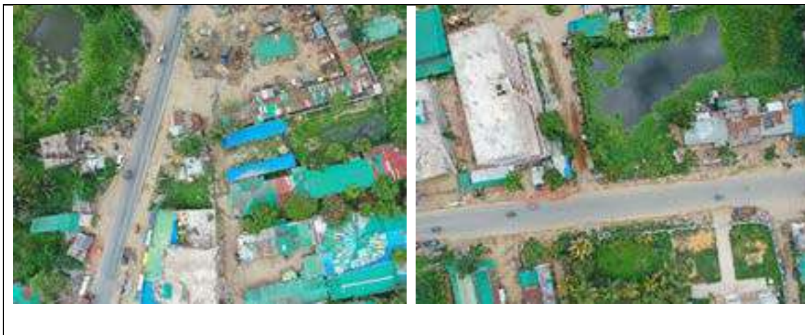
Figure 3-11: Drone Image of Ramu Upazila
