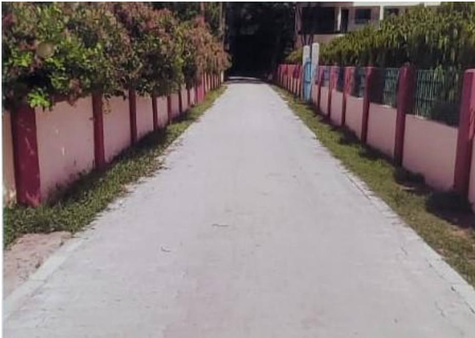
Rehabilitation of Paygram kashba judge Rd road from Ch. 00m - 1250m (e-tender/LGED/Khul/GOBM/22-23/W-40) Road ID: 247694026
