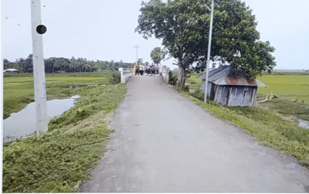
247943001-Improvement of Ajogara UP Office -Kola Bazar via Sreepur bazar Road (Start from Agaroa mtala R&H Road) by BC at Ch:4298-7290m under Terokhada Upazila(KDRIDP/Khul/W-141/2021-22)
