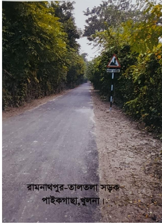
247644001 - Improvement of Ramanathpur-Taltala Road By BC (Ch.00m - 1200m)(KDRIDP/Khul/W-136/2021-22)
