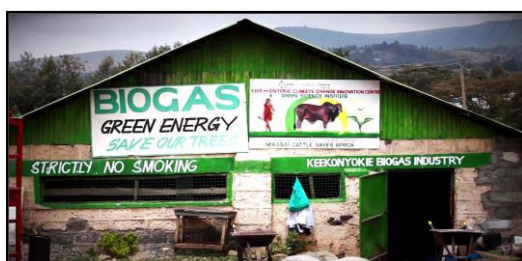
Biogas facility at Keekonyokie slaughterhouse
