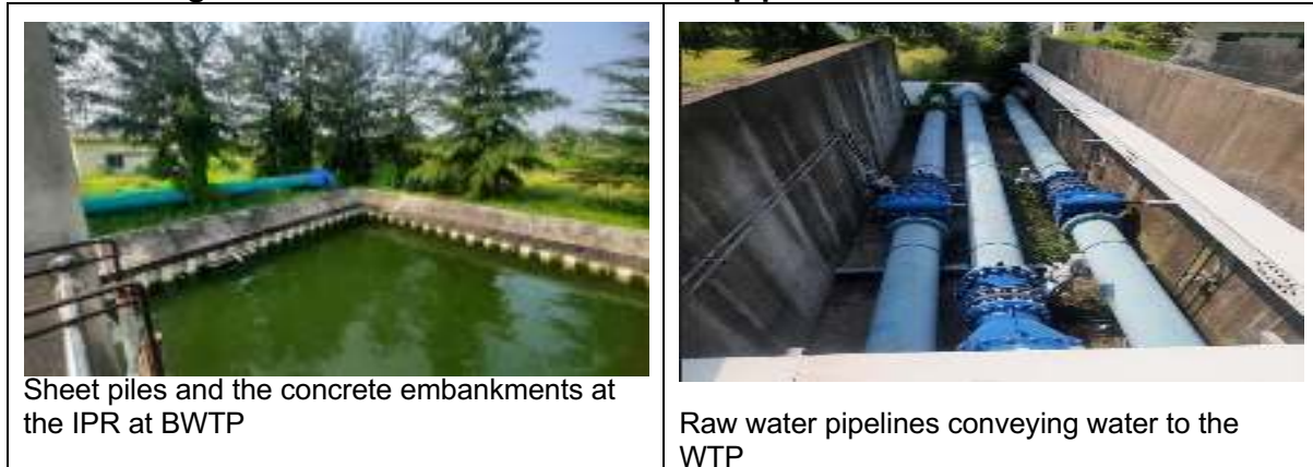
Figure 60: The embankments and the pipelines in the IPR at BWTP
