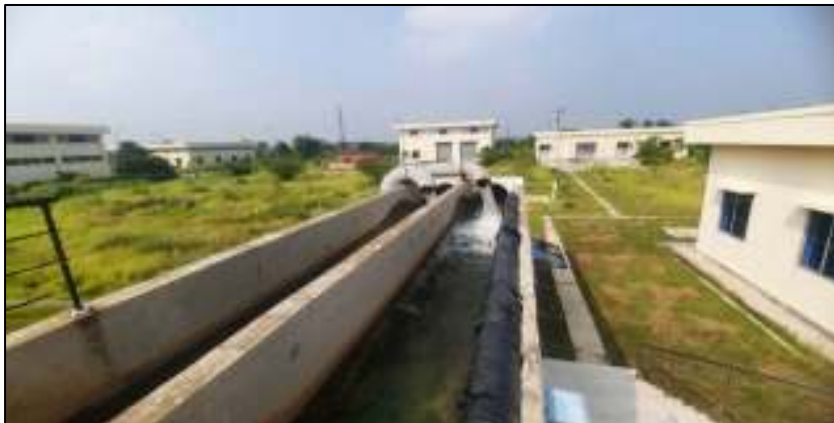
Figure 71: Backwash water is collected at a pond located near the BWTP, and sediments are allowed to settle before being recycled back to the BWTP
