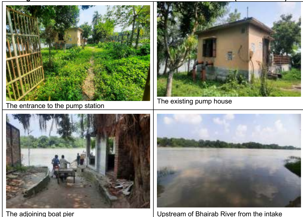
Figure 55: Photos taken at the intake location at the Afil Gate (Bhairab River)
