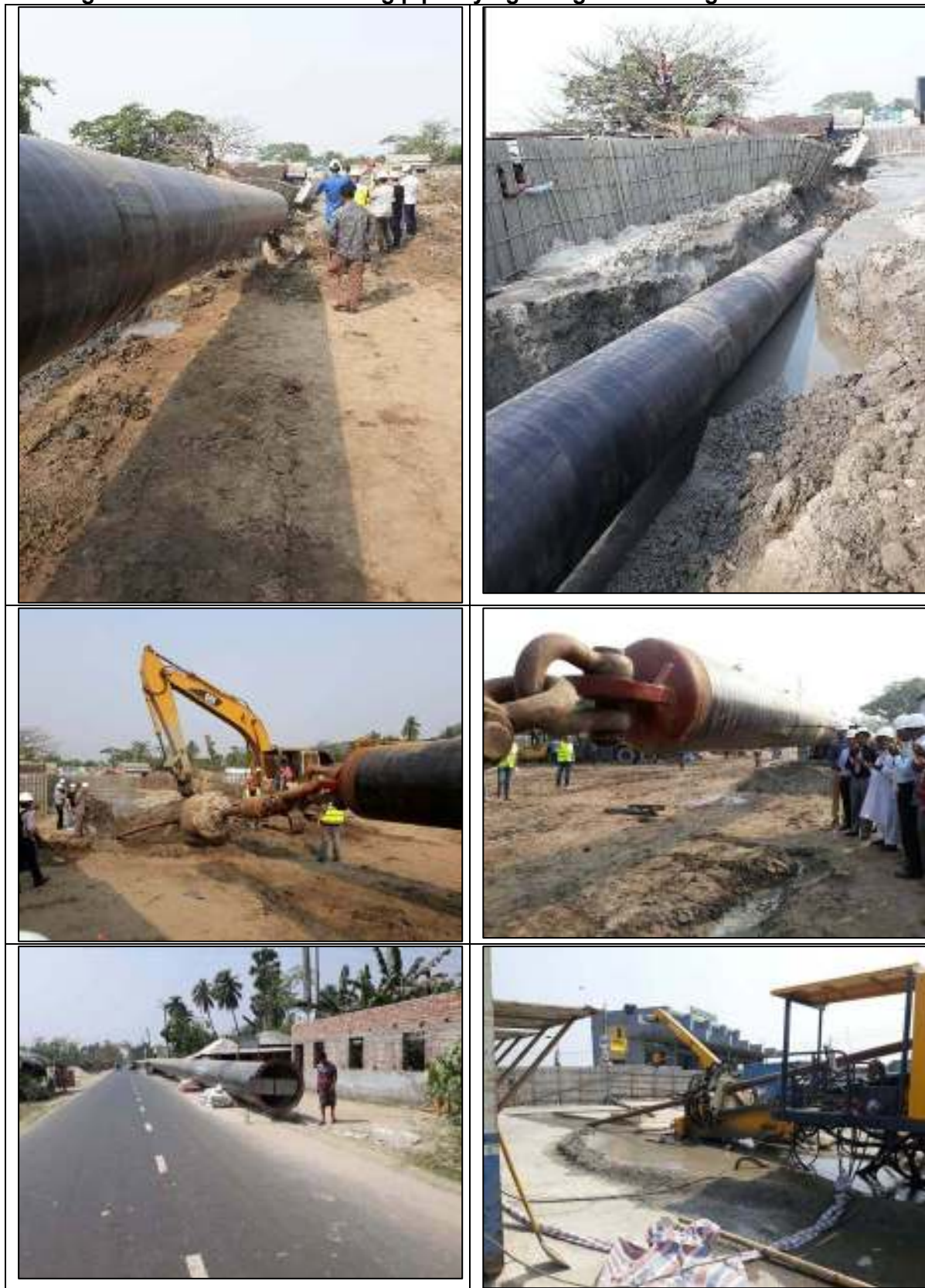
Figure 67: Photos taken during pipe laying using HDD during KWSP Phase I
