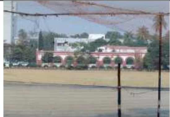
An old building within Khulna city
