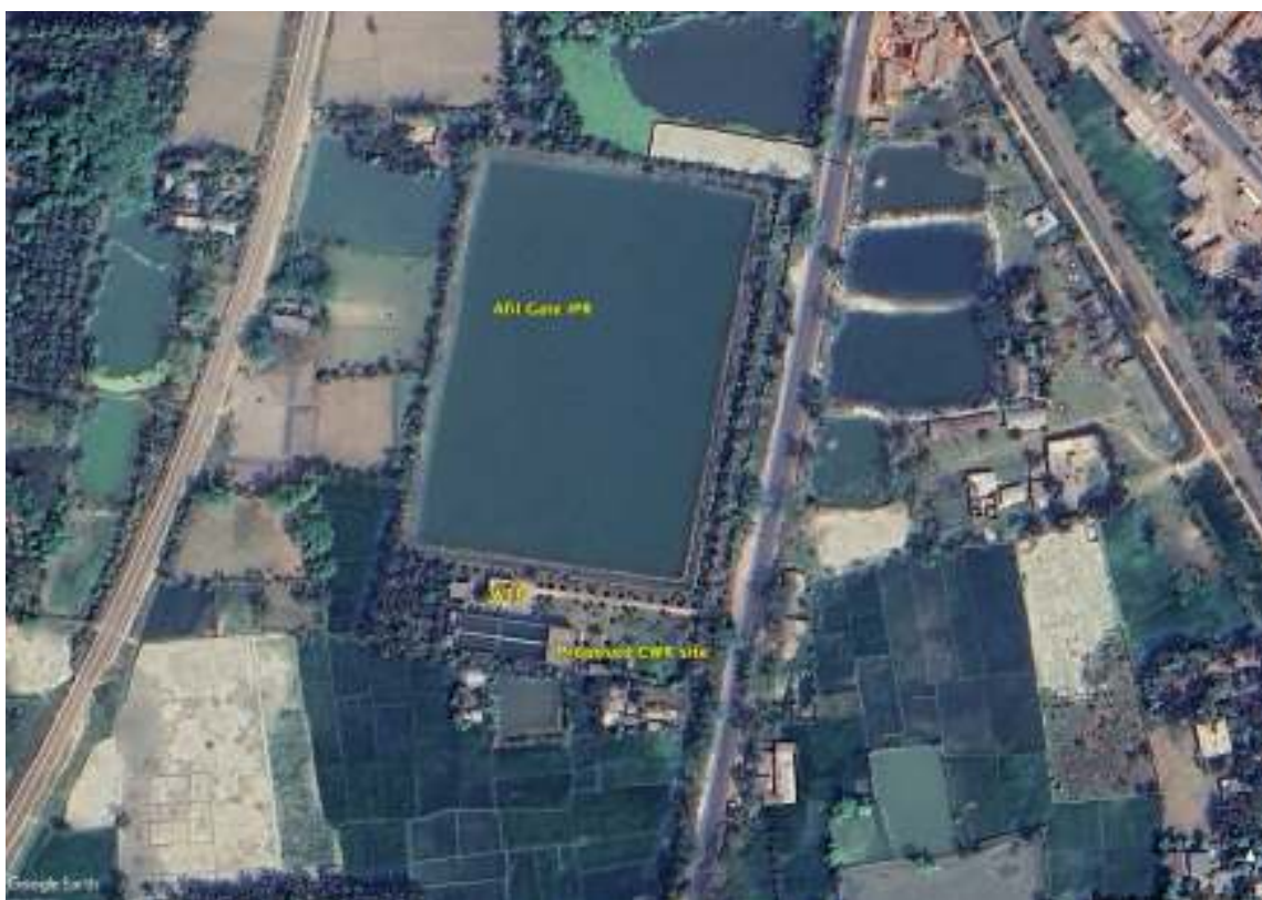
Figure 8: Water Treatment Plant and IPR at Afil Gate
