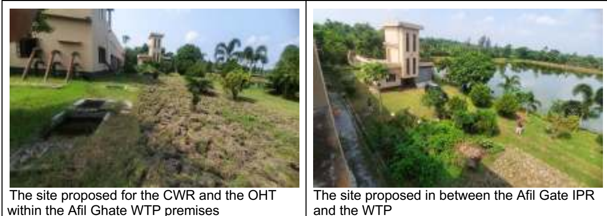
Figure 65: Photos taken at the site proposed for CWR 3, OHT and pump house
