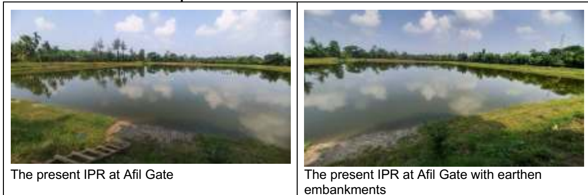
Figure 58: Photos taken at the location of Impounding Reservoir at Afil Gate where the dept will be increased from 3 m to 10 m
