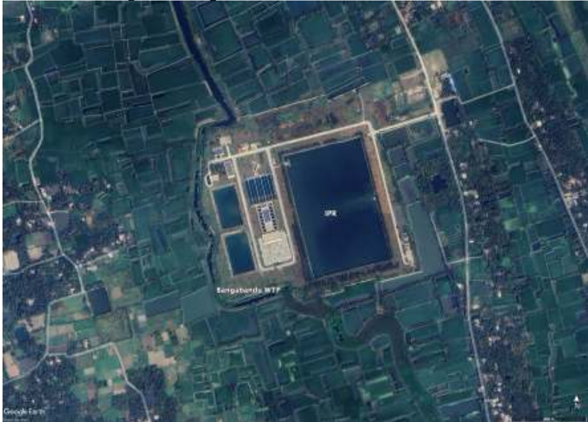
Figure 6: Bangabandhu Water Treatment Plant and IPR
