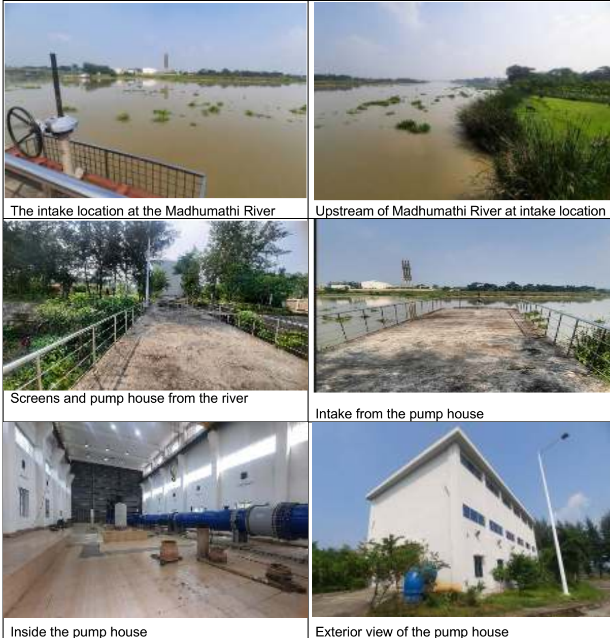
Figure 54: Photos taken at the Mollahat intake and raw water pump house
