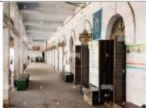
Old Train station building of Khulna
