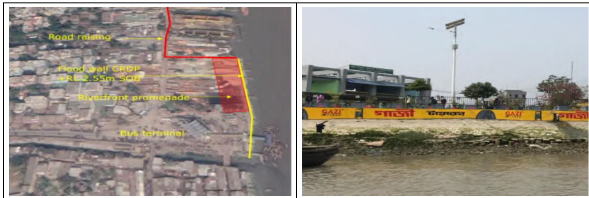
Figure 3.15 Current Situation of Riverfront North of Rupsha Ghat (2021)
