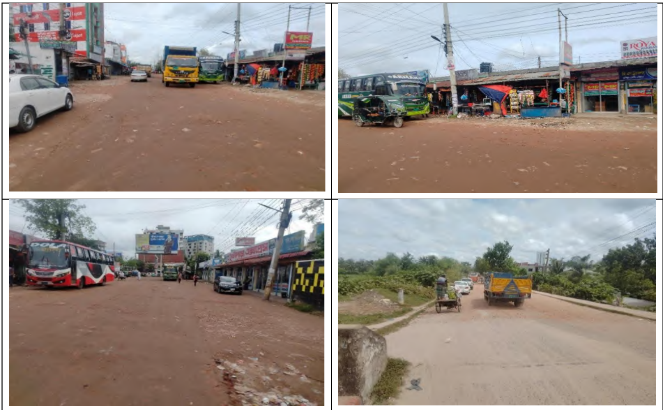
Figure 3.18 Existing Site Condition of Sonadanga Bypass Road
