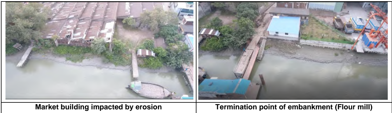
Figure 3.7 Drone Footage of Shoreline Showing Existing Condition of Subproject 1 (2021)
