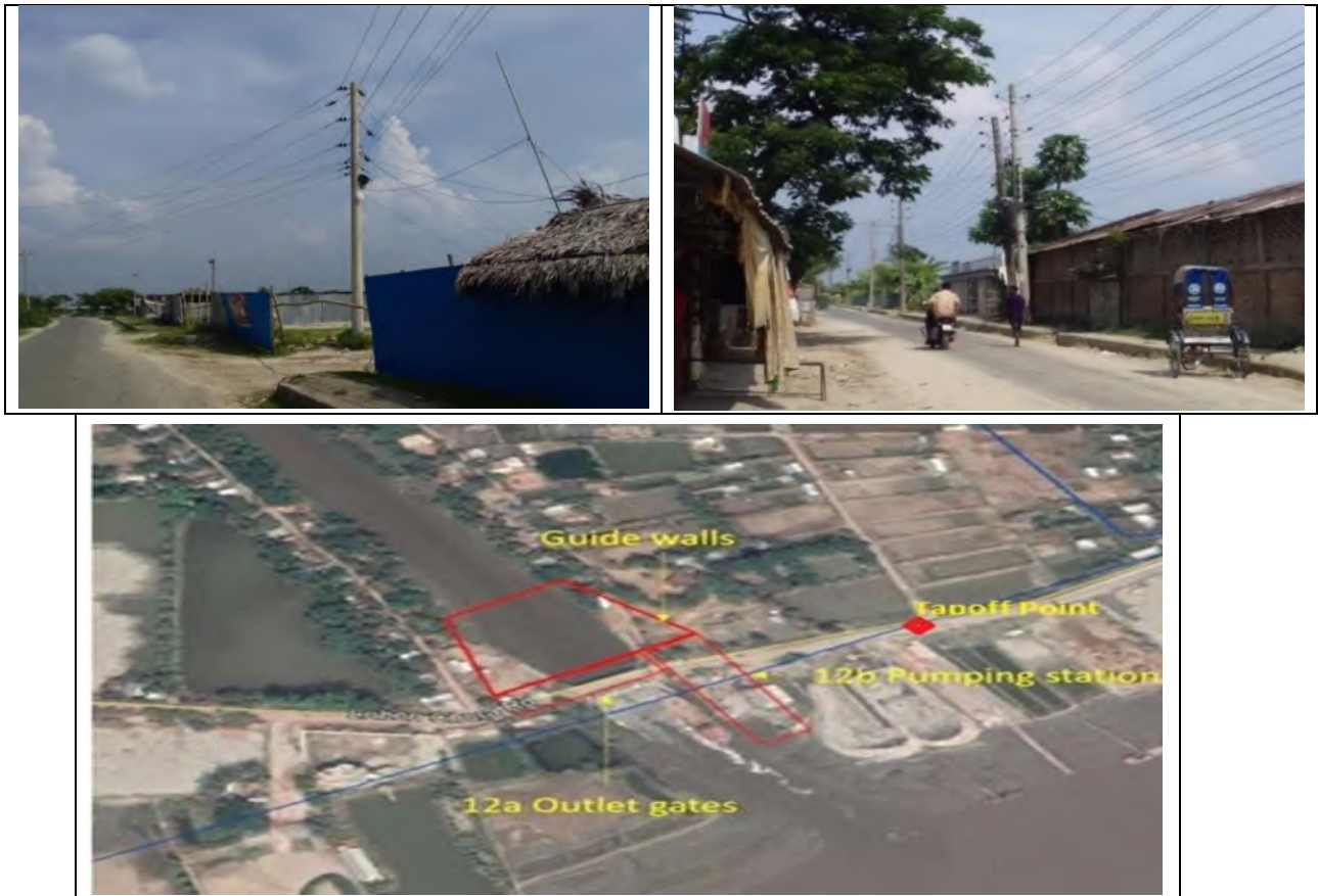
Figure 3.36 Location for Power Supply tap off Point at Labonchara and Nearest Point at Alutola
