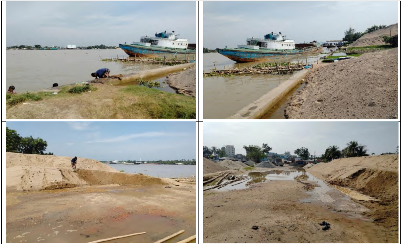
Figure 3.12 Existing Site Condition of Proposed Rupsha Riverfront Park Area (2025)
