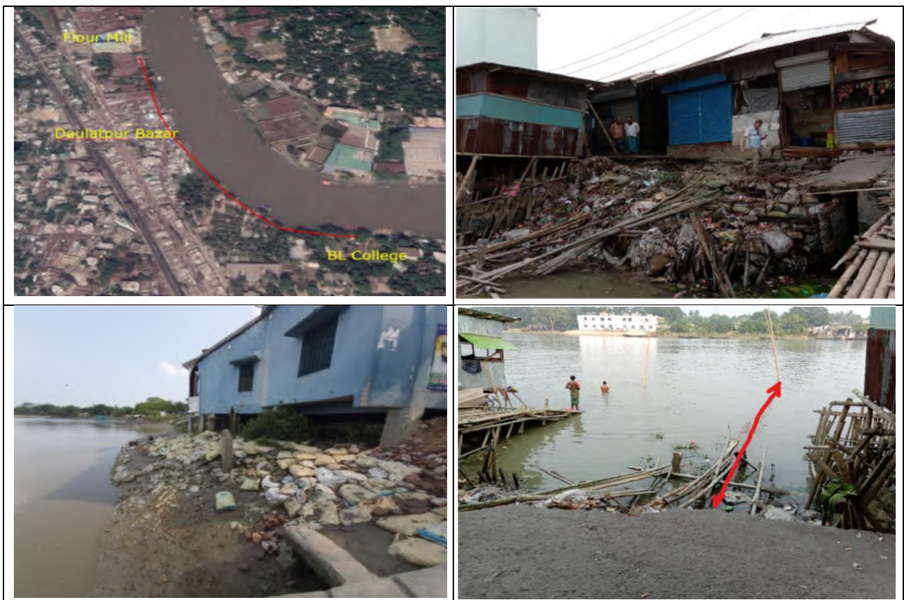
Figure 3.5 Existing Condition along the shoreline at Daulatpur Bazar (2021)
