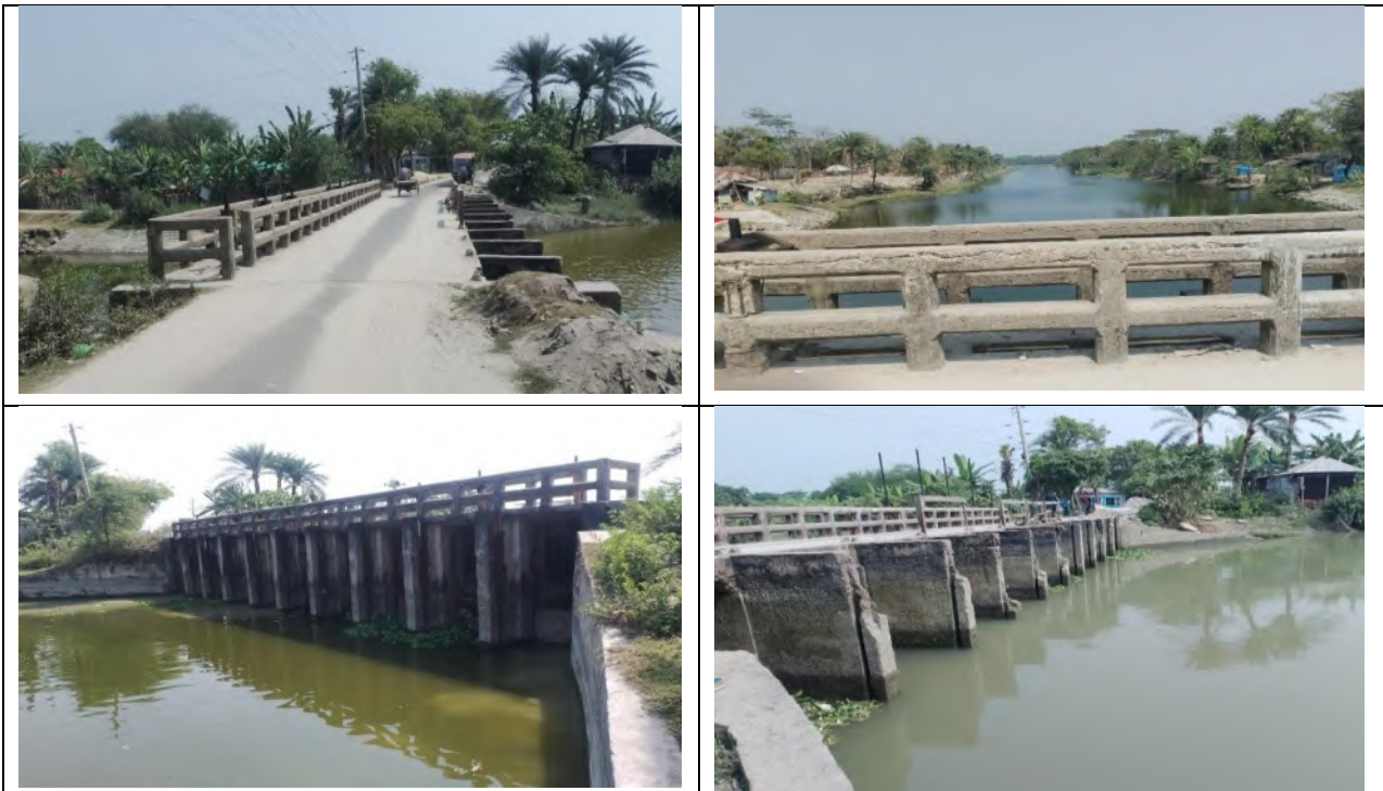
Figure 3.38 Existing Site Condition of Alutola Outlet Gates (2025)
