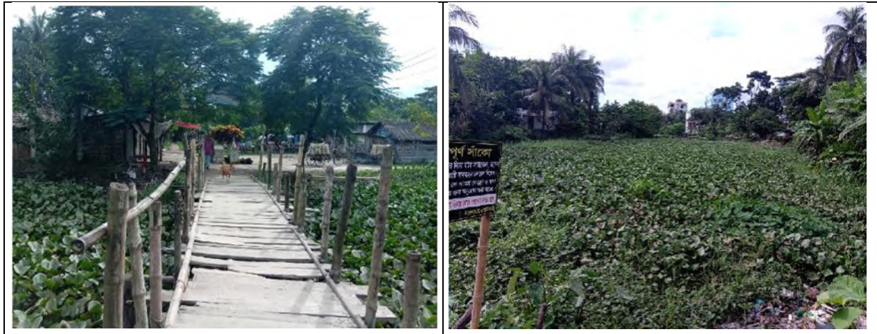
Figure 3.45 Existing Conditions of the Nirala Khal (2021)
