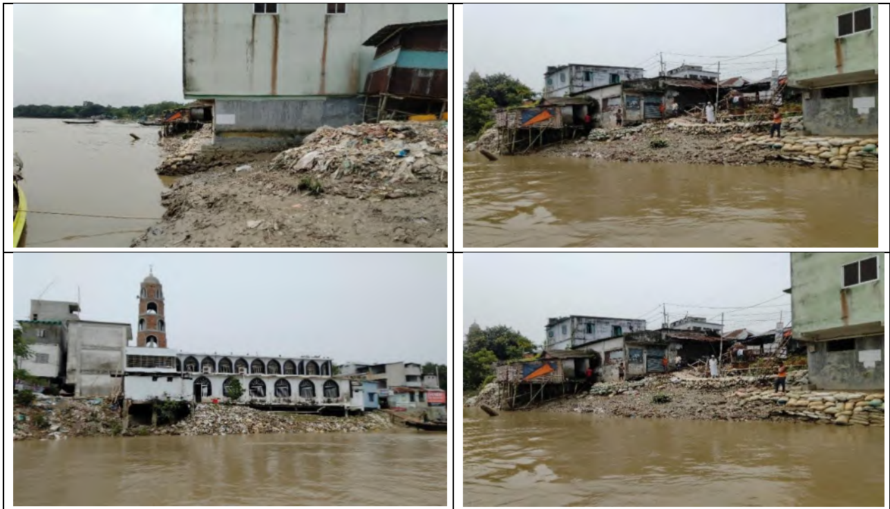
Figure 3.1 Existing site condition of Daulatpur Embankment Area (2021)
