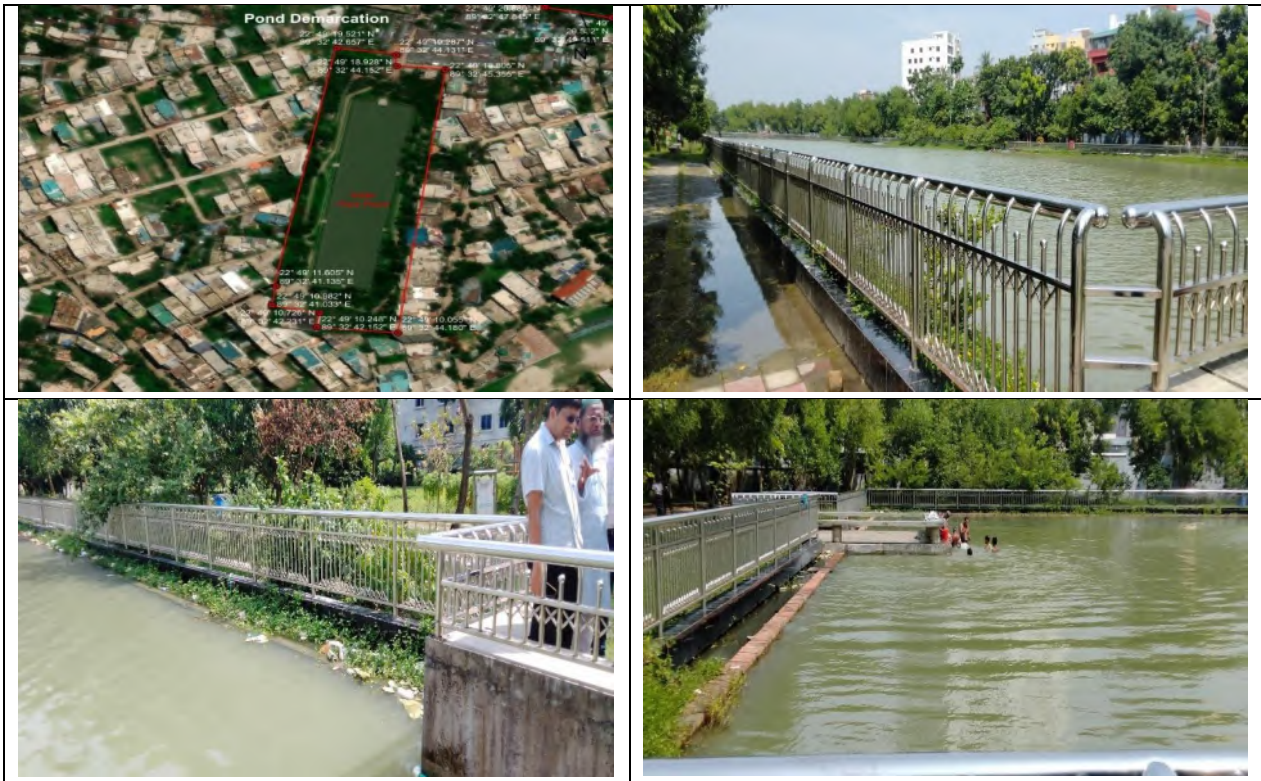
Figure 3.80 Existing Condition of Solar Park Pond (2021)
