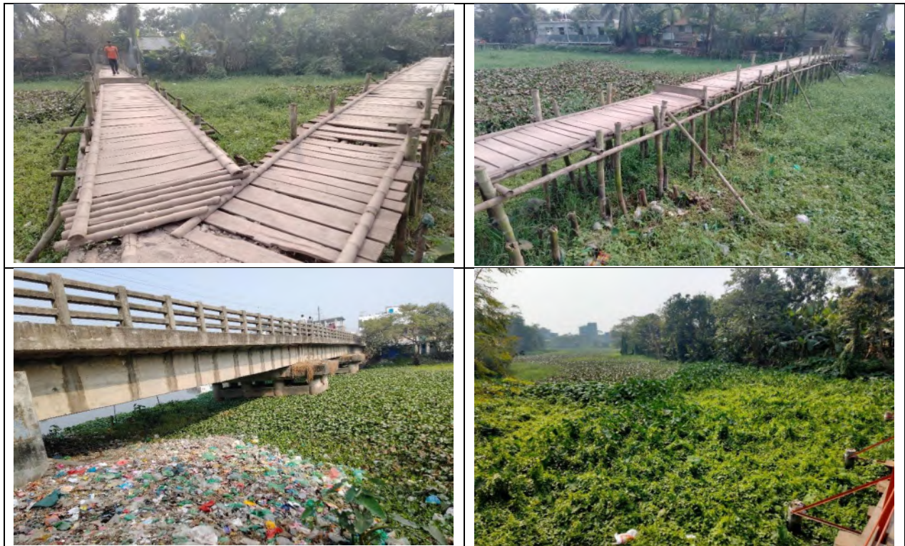
Figure 3.48 Existing Conditions of Bridge Location of the Nirala Khal (2025)
