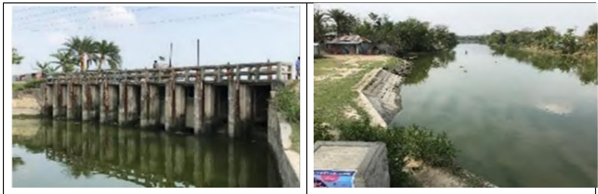
Figure 3.40 Existing Conditions of Alutola Outlet Gates (2021)
