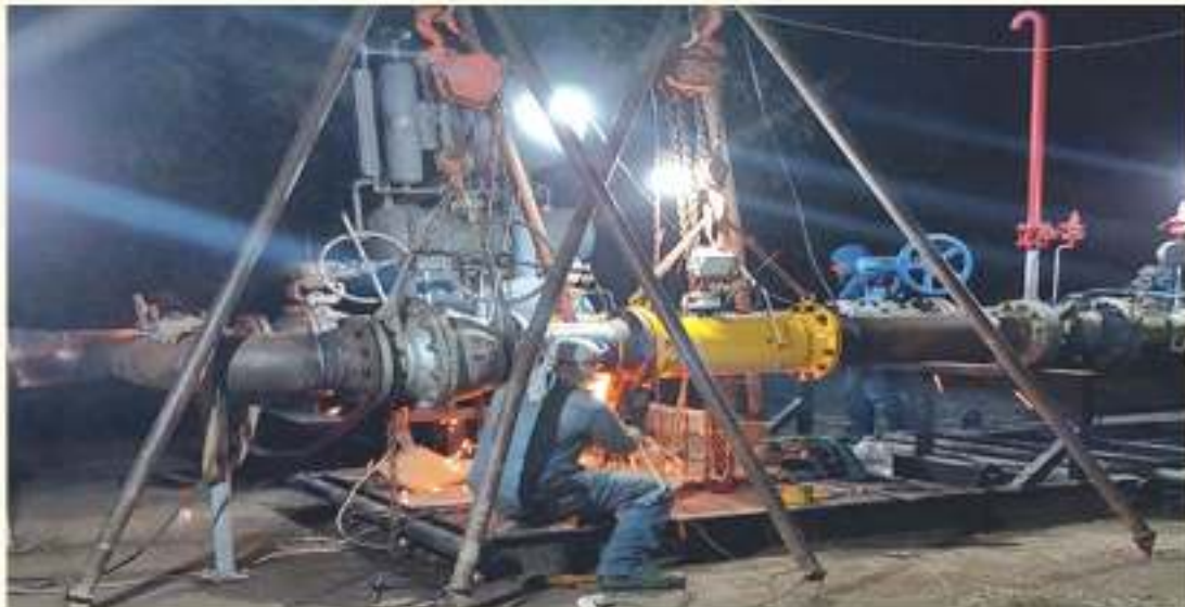
Installation of Meter through Fabrication at KEPZ CRS
