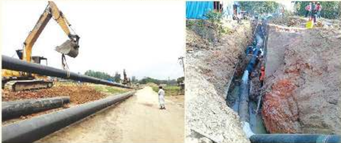
▶ Pipeline Installation Activities under the Mirsharai Upgradation Project.
