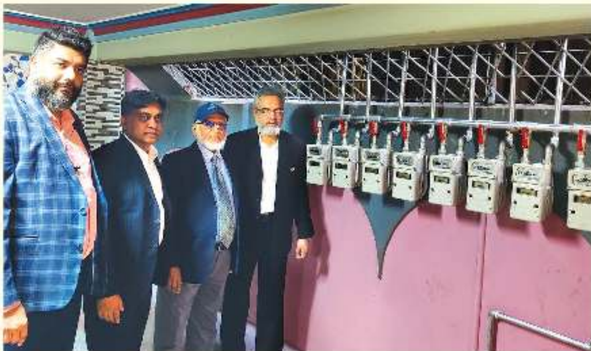
■ Inspection of Pre-paid Meter Installation Activities in Residential Customers' Premises.
