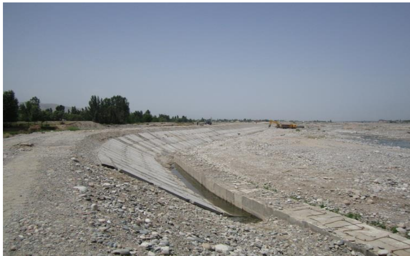
Figure 37: Under Construction River Bank Protection with Slab and CC cubes
