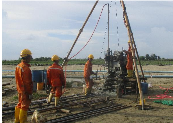
Figure 44: Soil test for jetty construction
