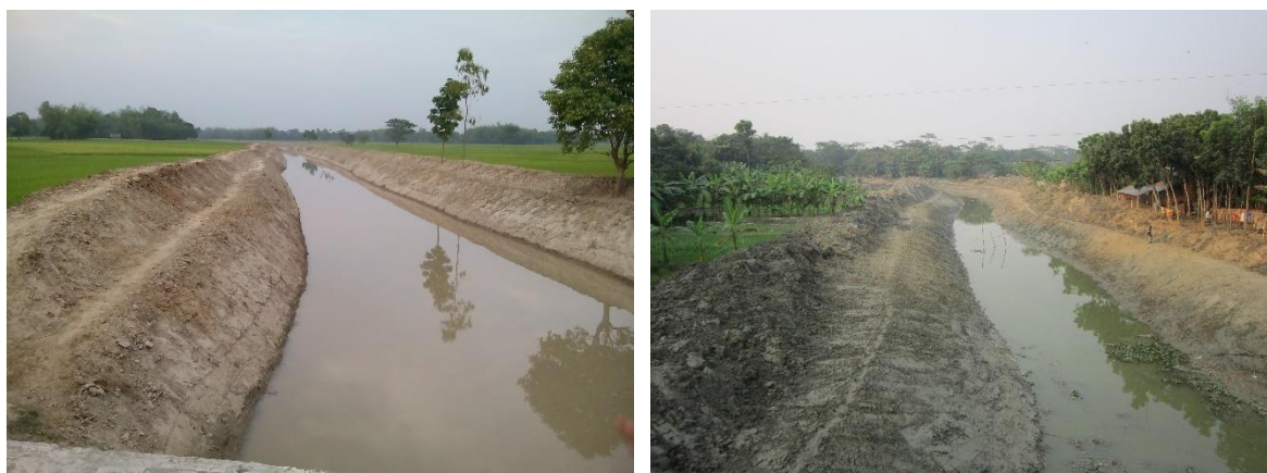
Figure 19: Khal re-excavation
