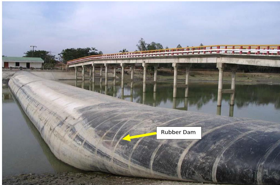
Figure 21: Use of Rubber Dam
