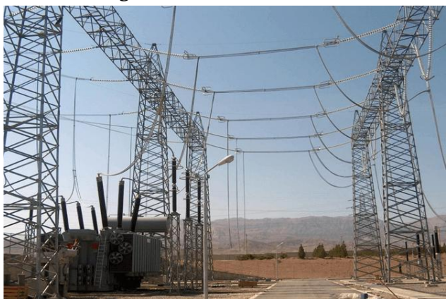
Figure 62: Busbar Assemblies
