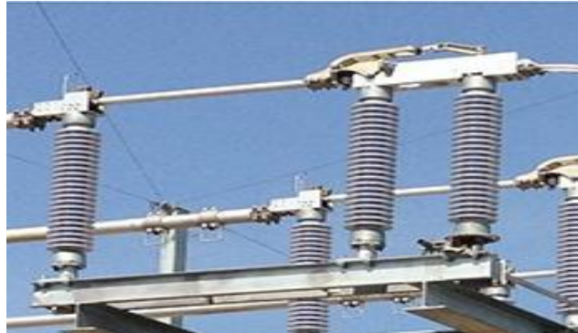
Figure 60: Disconnect switches
