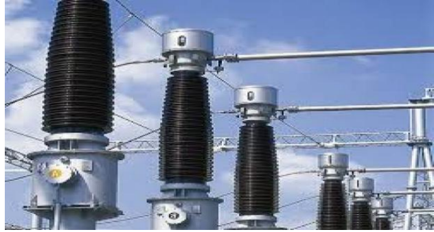
Figure 59: Current Transformers
