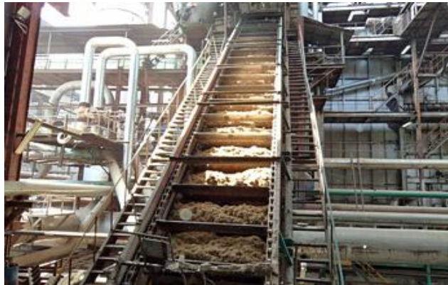
Figure 89: Material Handling and Storage
