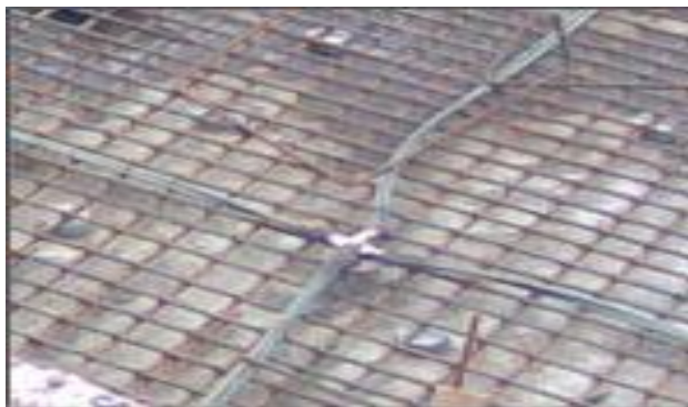
Figure 52: Grounding System
