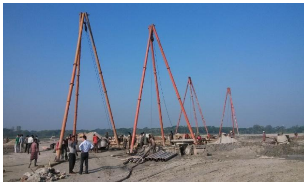
Figure 20: Boring Work for Piling
