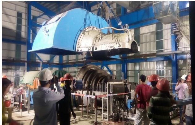
Figure 29: Steam Turbine
