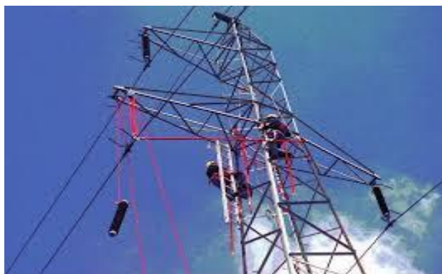
Figure 46: Insulator Fitting
