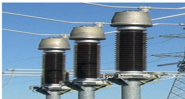
Figure 58: Voltage Transformers
