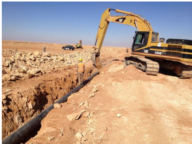
Figure 80: Back Filling
