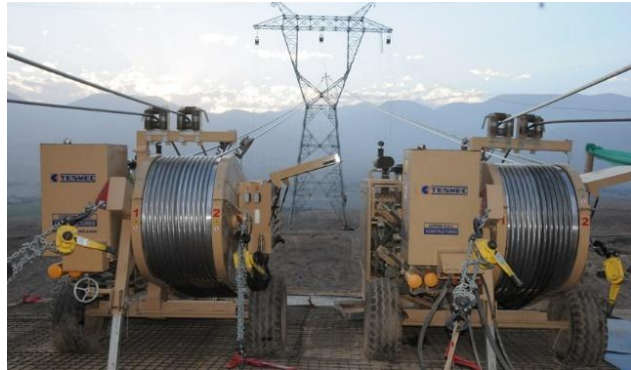
Figure 47: Stringing of Conductor
