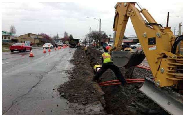
Figure 71: Trenching
