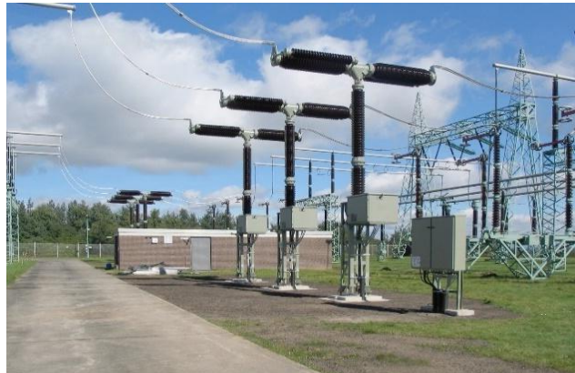
Figure 61: Circuit Breakers
