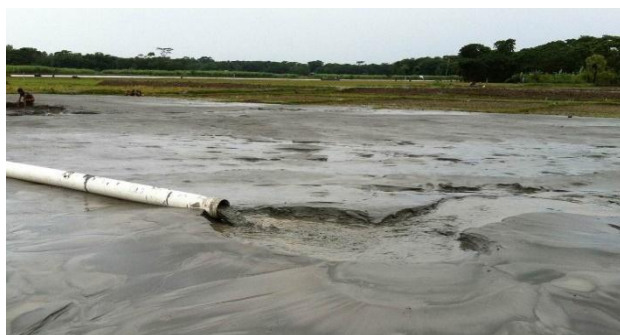
Figure 16: Land Development Work
