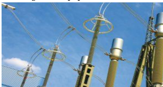
Figure 57: Lightning Arresters
