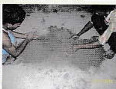
Mixing of Soil Cement with Water
