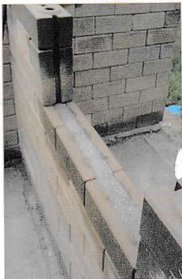
FIGURE 8: PLACEMENT OF MORTAR UP TO CEILING HEIGHT
