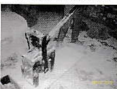
Mechanical Compaction after hand Compaction
