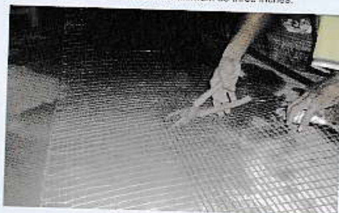
Figure 2: Preparation of mesh
