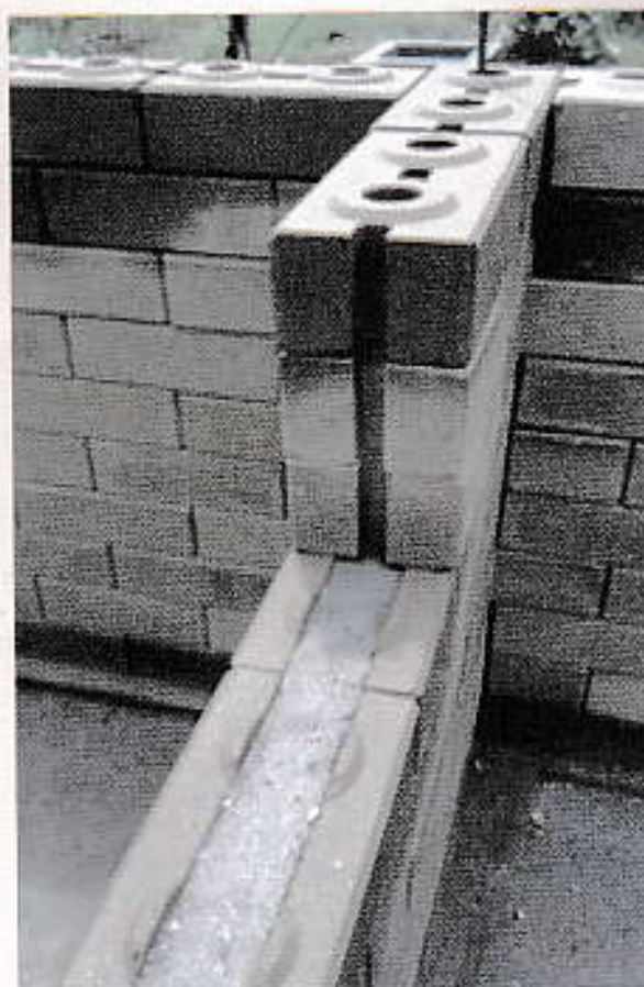
FIGURE 8: PLACEMENT OF MORTAR UP TO CEILING HEIGHT
