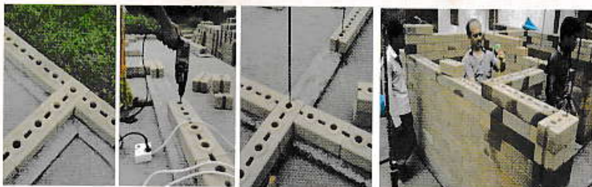
FIGURE 7: PLACEMENT OF FIRST COURSE OF BRICKS
