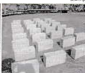
Curing in open air and Shed
