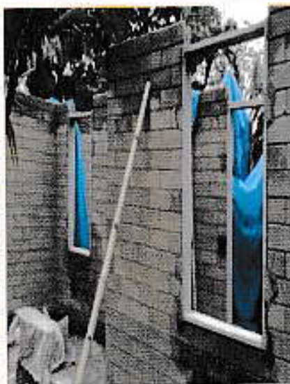
FIGURE 9: PLACEMENT OF CHOWKATH
