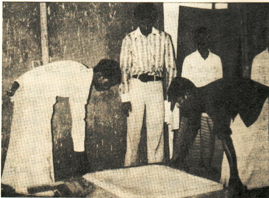
Fig. 6. Casting of funicular D.C. Shell on Process (ref. Fig. 2.)
