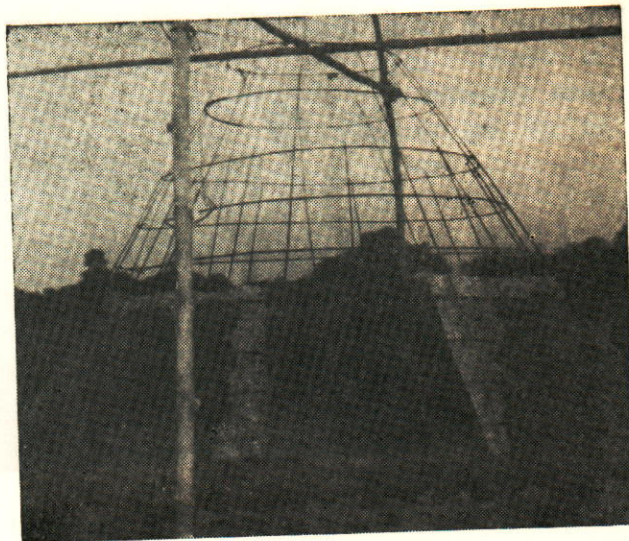
Fig. 2. Paste of mortar is being placed over chicken netting reinforcement
