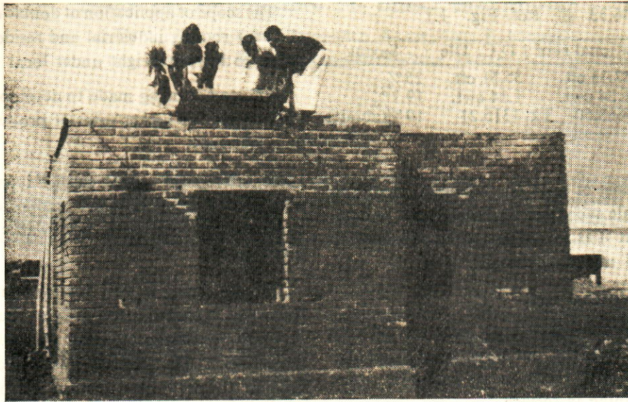
Fig. 7. Construction of funicular D.C. Shell roof in process
