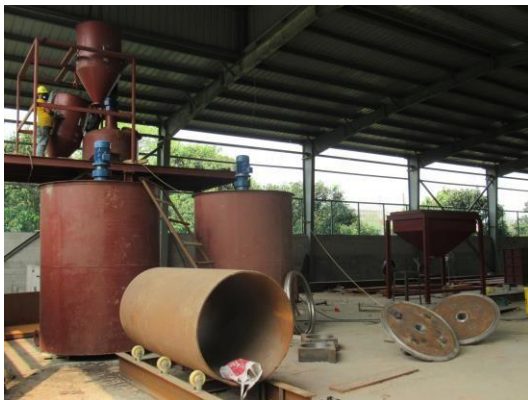
Figure: Setting up work of Equipment tank, ball mill)
