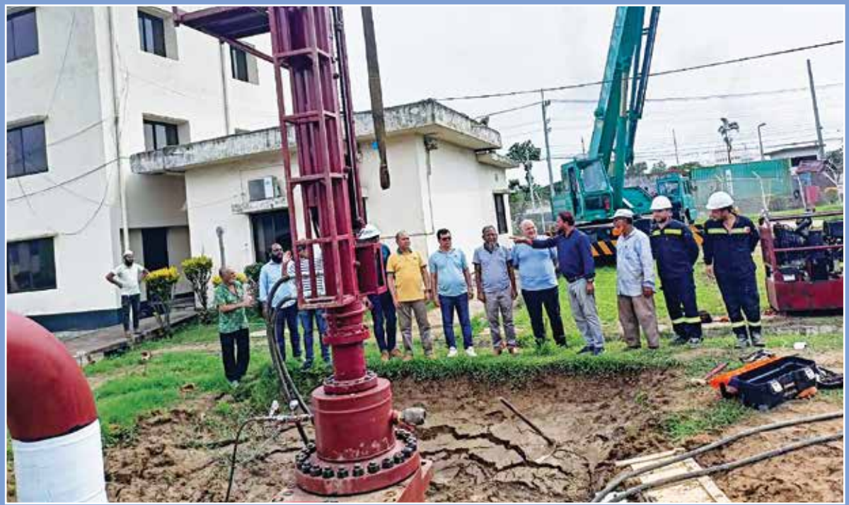
On Stream Hot tapping activities at Faujdarhat CGS under 'Installation of Gas Stations on Off-Transmission Points and Modification Project' of GTCL.
