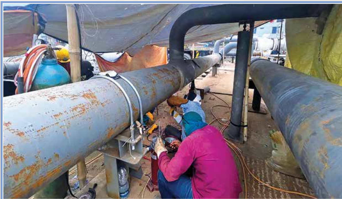
Mechanical fabrication activities of Ashulia CGS under Installation and Modification of Gas Stations at Off-Transmission Points of GTCL
