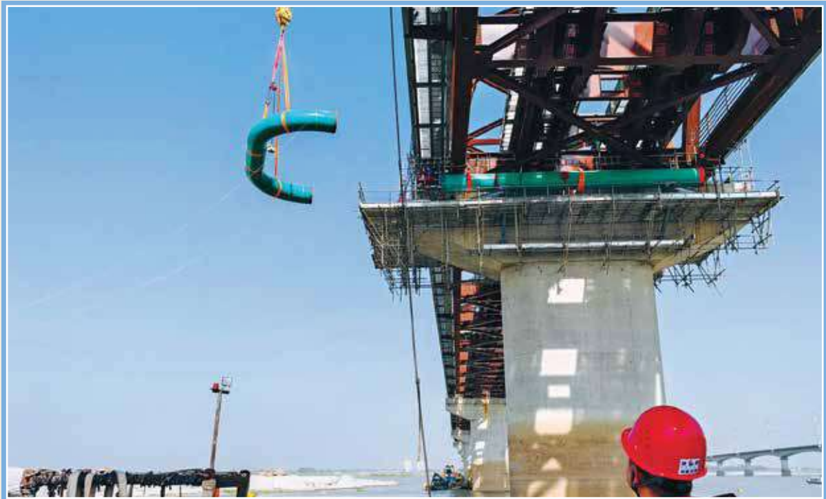
Installation of expansion loop for the gas transmission pipeline at Jamuna Railway Bridge
