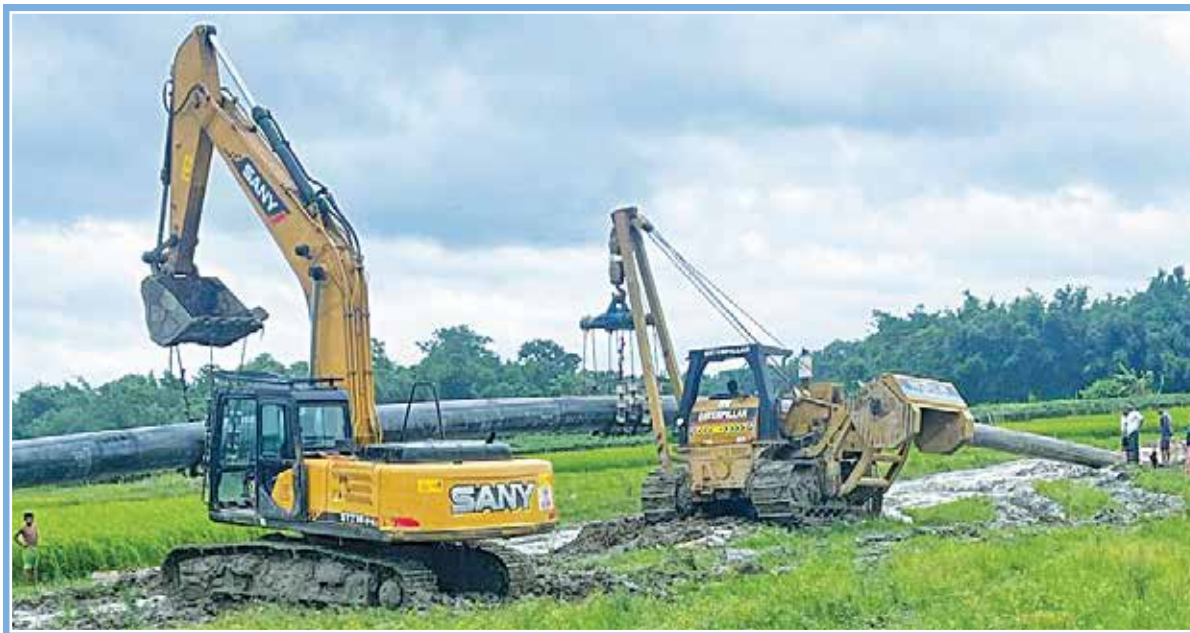
Pipeline replacement works: 24" dia Arial kha River crossing using HDD method
