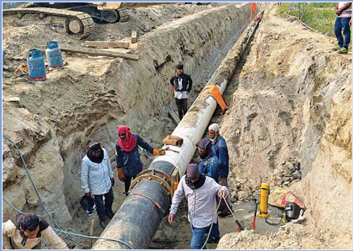
24" dia Brahmaputra River crossing tie-ins activities after HDD river crossing works
