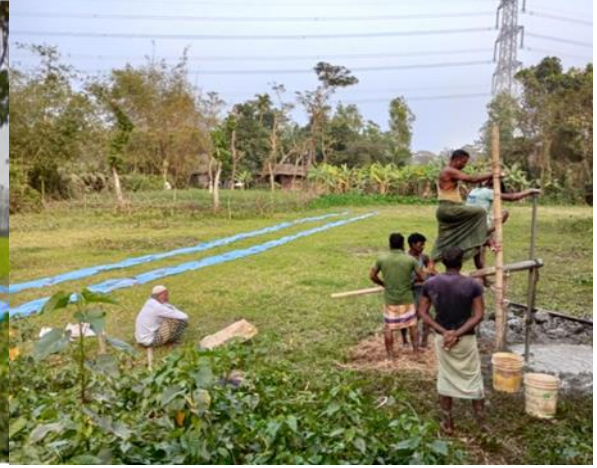
Figure 7: Samples Collected Through Local Wash Boring (Tubewell Boring)
