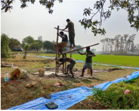
Figure 7: Samples Collected Through Local Wash Boring (Tubewell Boring)
