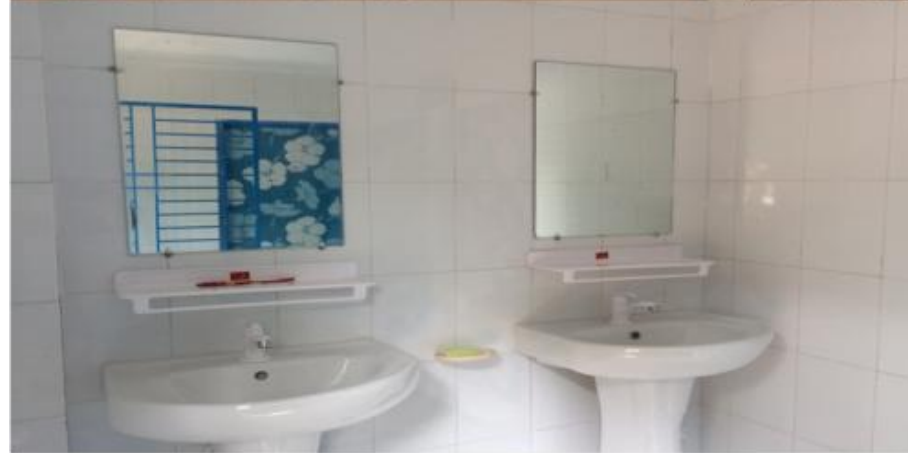
WASH Block at Ward-5
