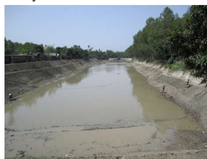
Khal re-excavation in Joshore
