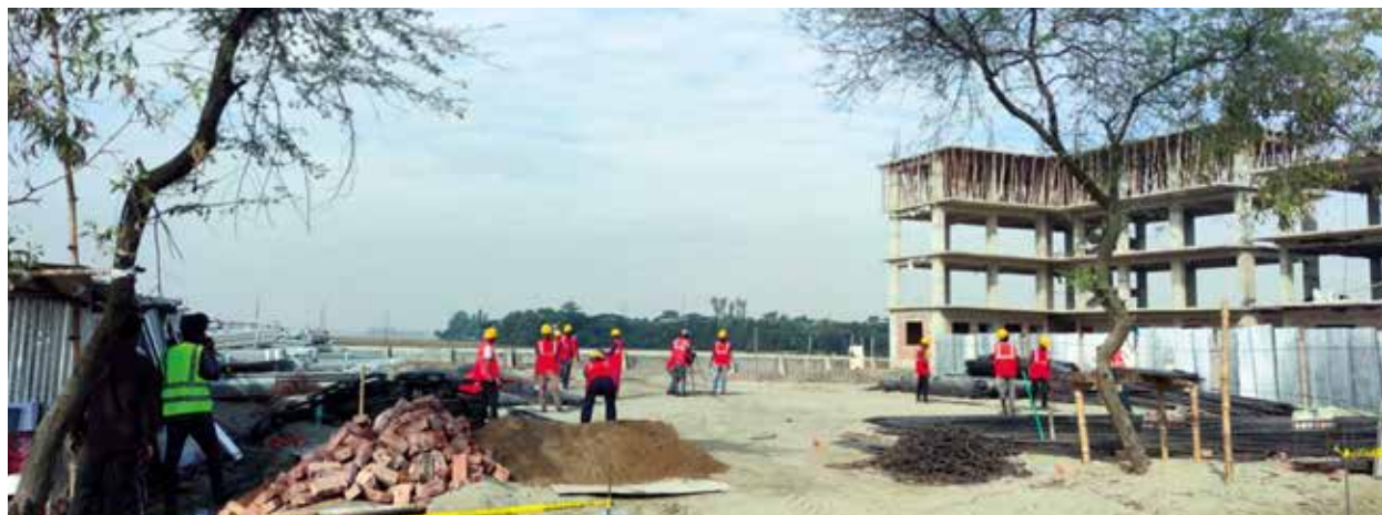
Residential building construction work of the Sonagazi 75 MW solar project
