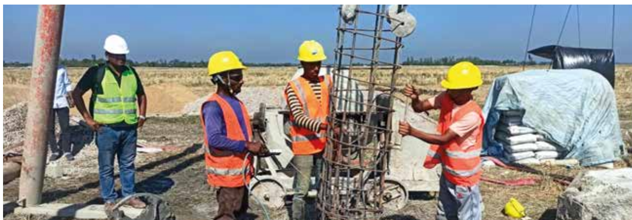
Transmission Line Piling Work
