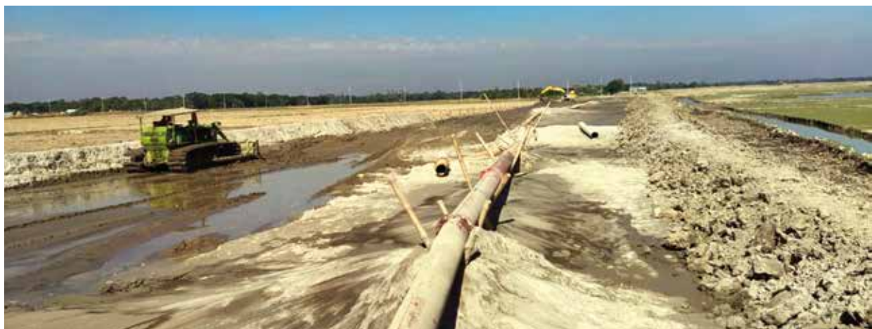
Land Filling Work of Sonagazi 75 MW solar project
