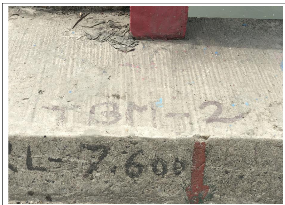
Fig: 7 Bench Mark (BM) on Musapur Regulator Deck
