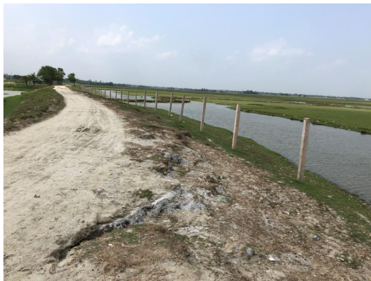
Figure 6: Existing Road side Canal along western boundary
