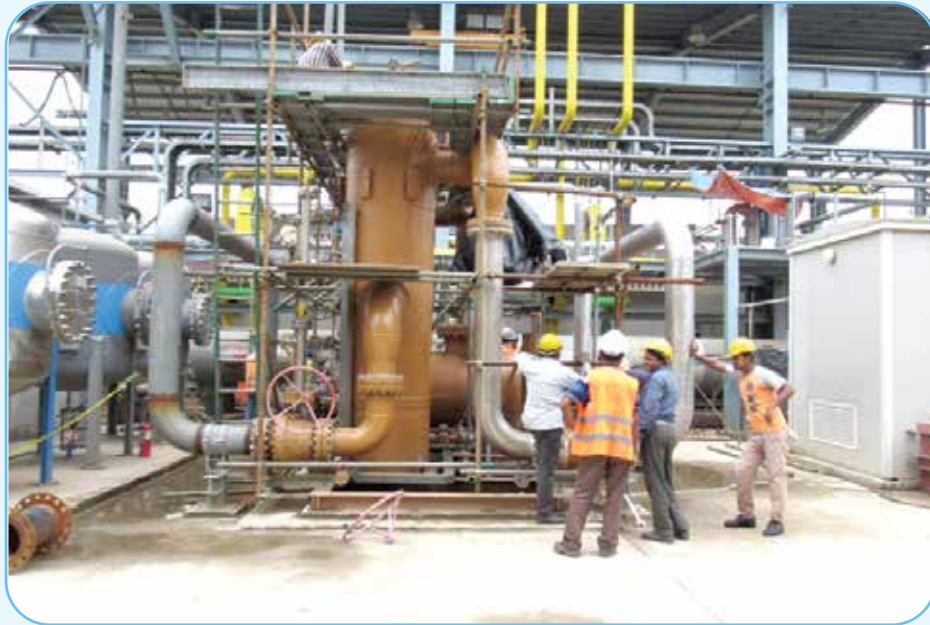
GBC (Fuel gas SS pipe line air blowing work)
