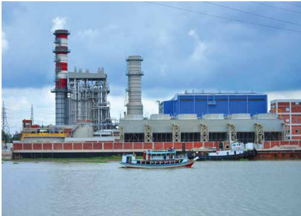
Haripur 412 MW Combined Cycle Power Plant
