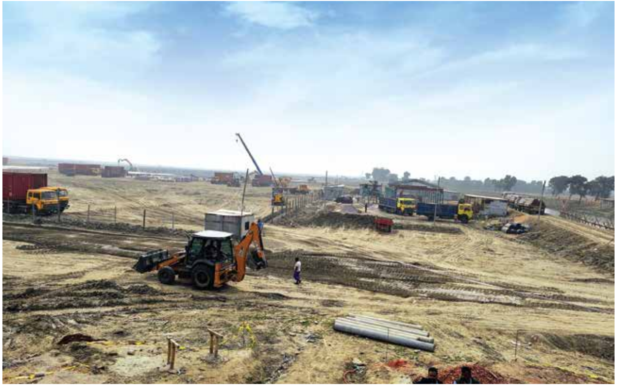
Construction works is going on at Sonagazi 75 MW Solar Power Plant Construction Project
