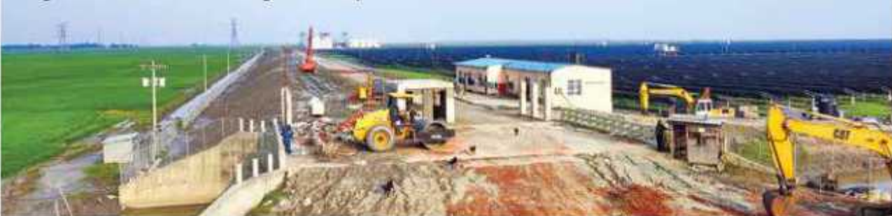
Sonagazi 75 MW Solar Power Plant during construction period
