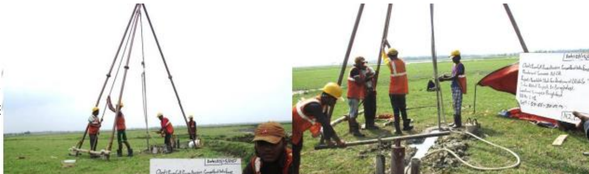
Figure 6: Geotechnical investigation site work
