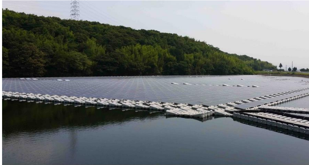
Figure 12: Floating solar plant of 1008 kWp located near Ono city, Japan
