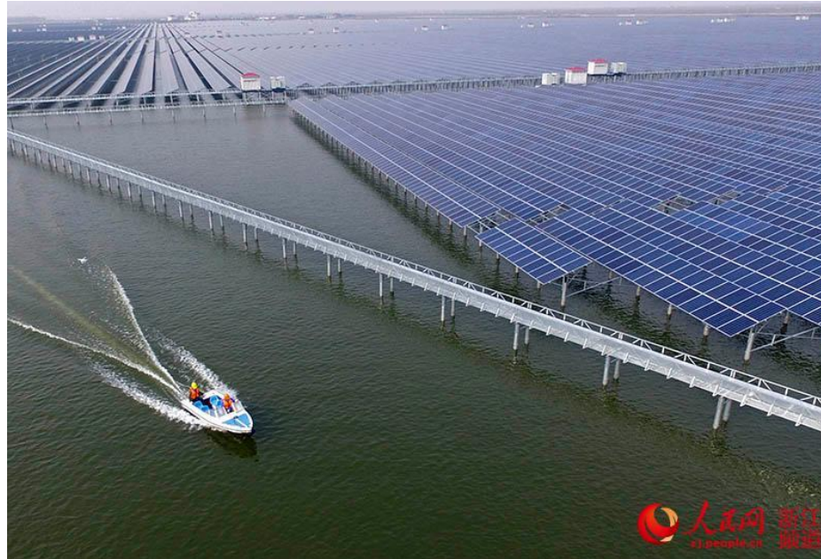
Figure 48: Eelevated PV plant concept for a fish farm underneath a 200MW PV in Zhejiang, China
