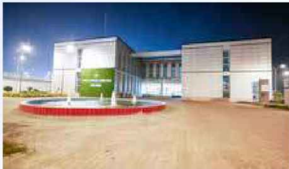
Daserkandi Sewage Treatment Plant
