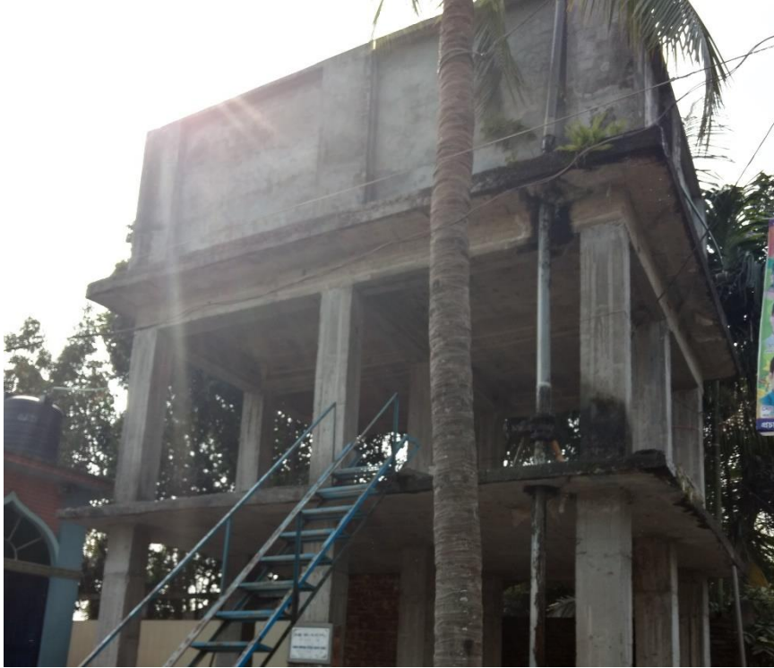
Figure 5: PTW with Overhead Reservoir (at Thulthulia bazar of Demra Union)
