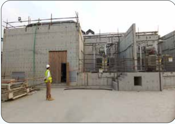
Figure 9: W35_Blower & Electrical Building
