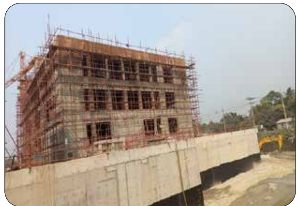
Figure 27: W91_Administrative & Lab Building
