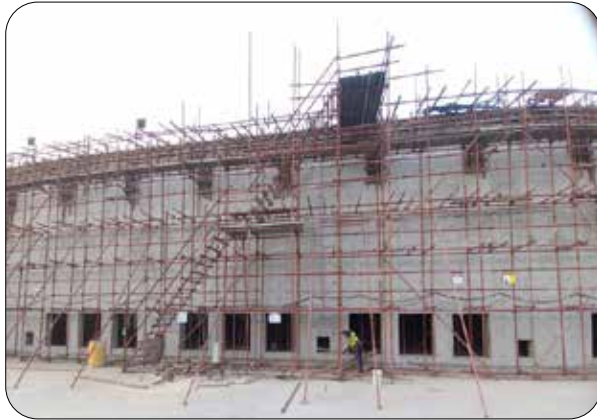
Figure 19: W45_Pumping Station Building
