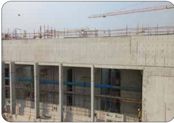
Figure 5: W20_Densadeg Channel & Pipe Gallery
