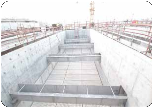
Figure 3: W30_Gravity Filter Pre-cast Slab & Metallic Trough
