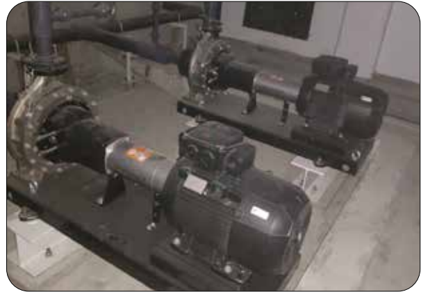
Figure 17: Lime/Alum Pump
