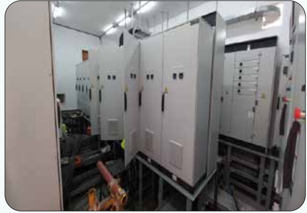
Figure 10: W35_ Electrical Panel & Cable pulling
