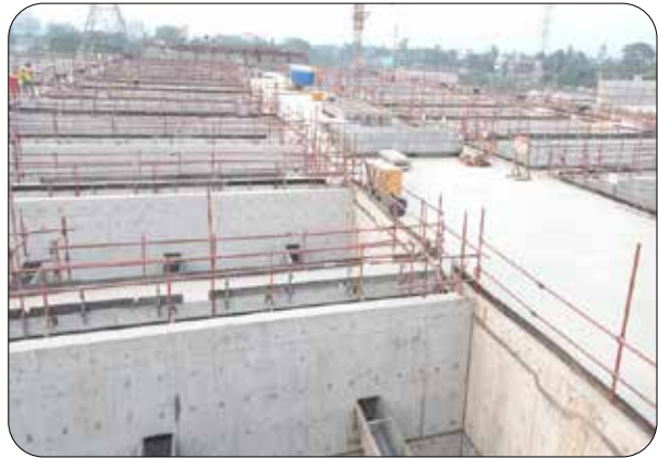
Figure 2: W30_Gravity Filter Top View
